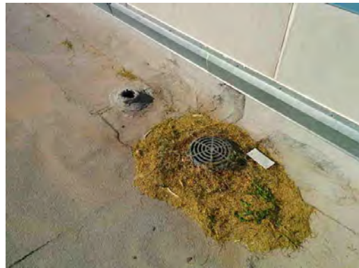
Guerrero ES - Debris at Roof Drain
