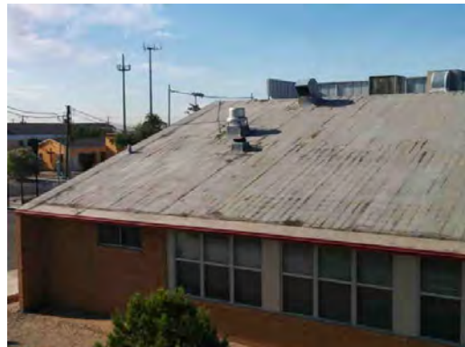
Hillside ES - Worn Roofing Material
