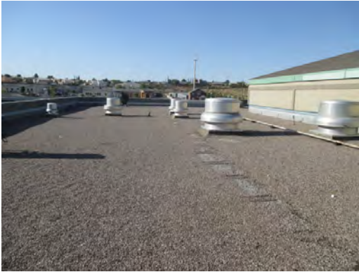
Franklin 9th Grade Center - Roof General Condition 01
