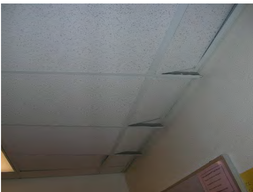
Chapin HS - Ceiling Damage
