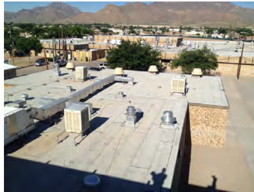
Charles MS - Roof Condition
