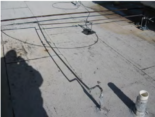
Schuster ES - No Support or Insulation on Water Supply
