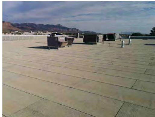
Irvin HS - Roof General Condition
