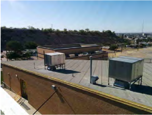
Lamar ES - Rooftop Units
