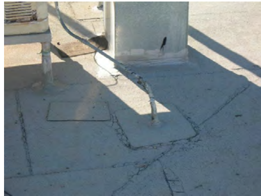
Putnam ES - Roof General Condition 04
