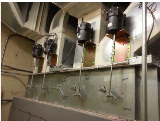
Clendenin ES - Carrier Air Distribution Dampers
