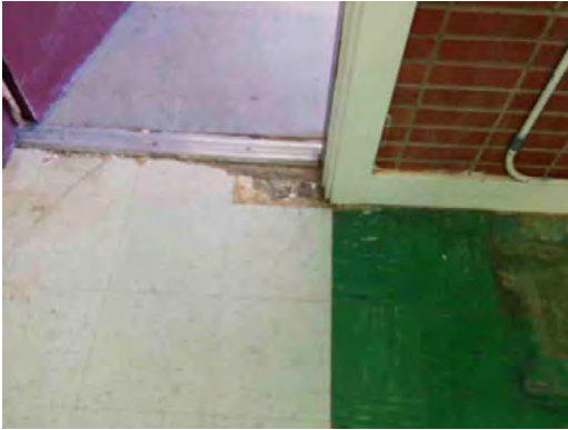
Wainwright ES - Damaged Floor at Threshold
