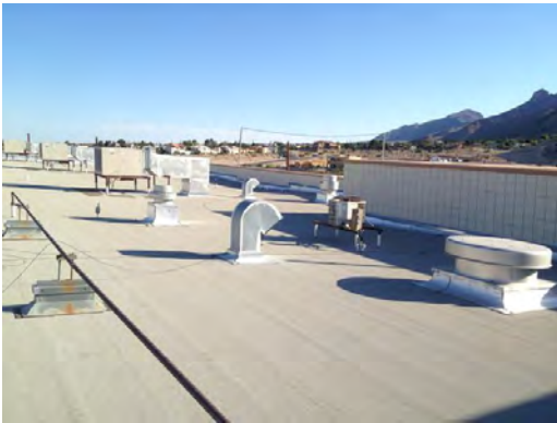
Green ES - Roof General Condition
