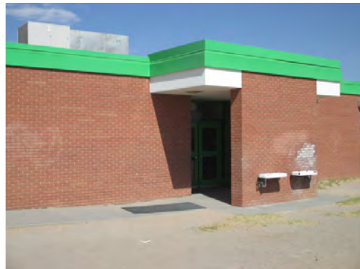
Roberts ES - Exterior Brick Requires Cleaning
