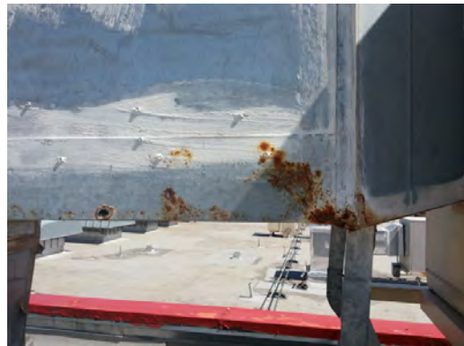
Bradley ES - Perforated Evap Duct
