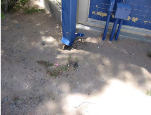
Schuster ES - Missing Splash Block
