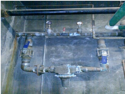
Crosby ES - Leaking Water Piping
