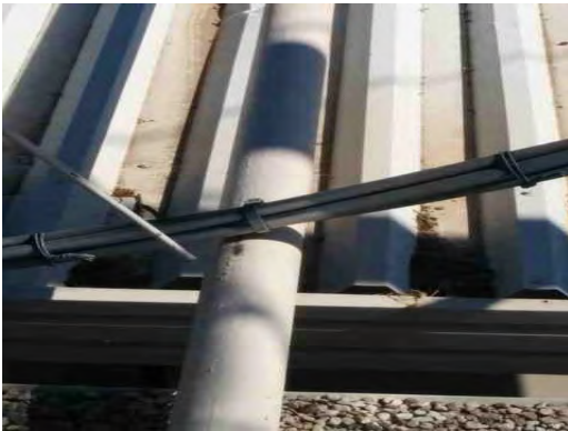
Wainwright ES - Electrical Wires Laying on Roof
