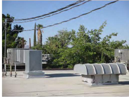
Polk ES - Rooftop Equipment 04
