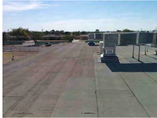
Bliss ES - Roof General Condition 01
