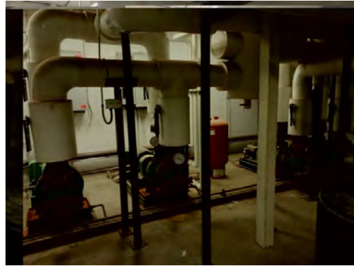
Aoy ES - Chilled Water Supply and Return Pumps
