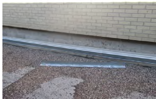
Franklin 9th Grade Center - Counter Flashing Damage
