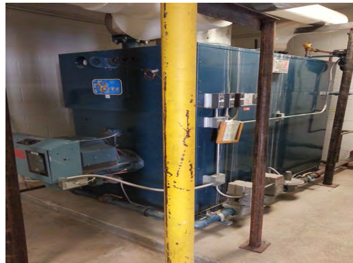
Aoy ES - Rite Heating Boiler
