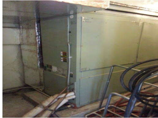
Alta Vista ES - Missing Insulation on Refrigerated Piping
