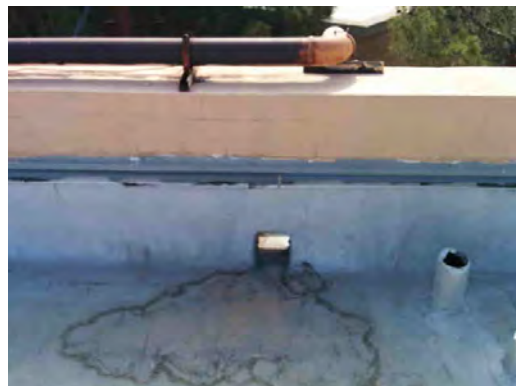
Vilas ES - Evidence of Ponding at Drain
