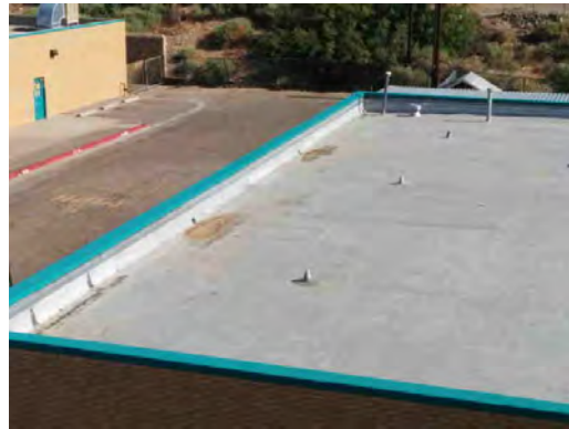
Center for Career & Tech - Roof General Condition
