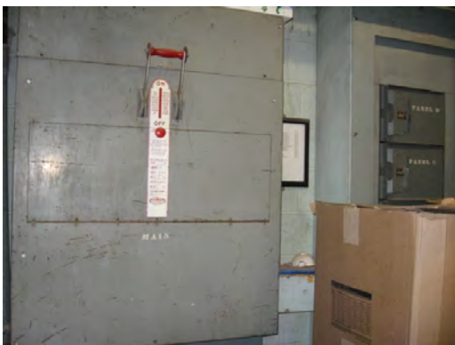
Dowell ES - Main Electrical Disconnect Switch
