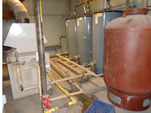
Coronado HS -Mechanical Room
