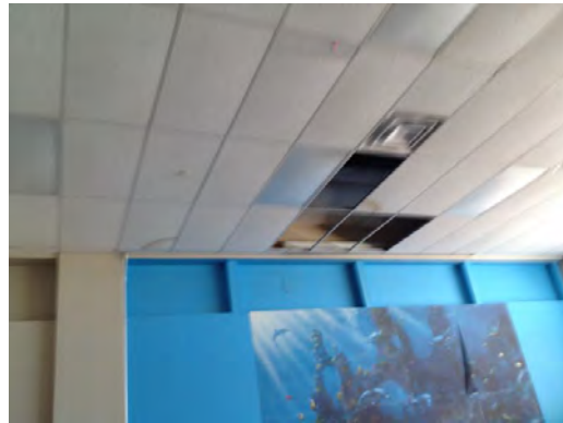
Brown MS - Missing Ceiling Tiles in Library
