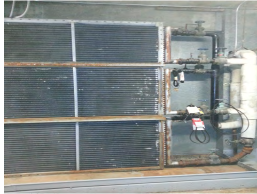
Clendenin ES - Chilled Water Coil
