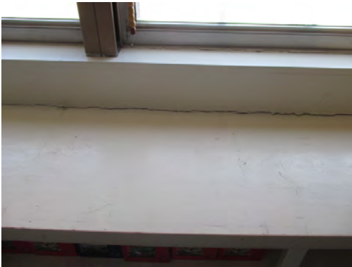
Cooley ES - Cabinetry Separating From Wall
