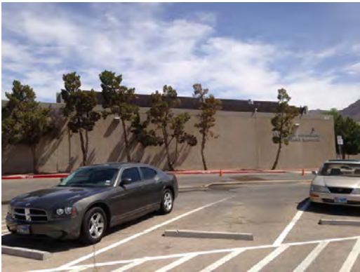
Johnson ES - Main Building Exterior
