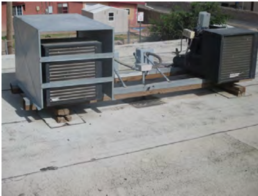
Clardy ES - Rooftop Equipment
