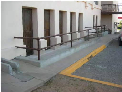
Alta Vista ES- Cracked Concrete Paving
