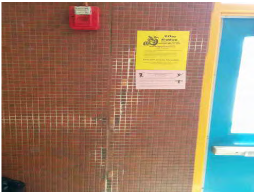
Rivera ES - Damaged Interior Ceramic Tile Wall
