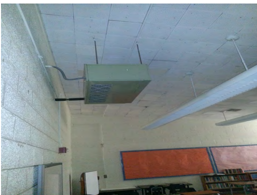
Burleson ES - Typical Classroom Heating Cooler
