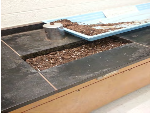
Crosby ES - Abandoned Lab Sinks
