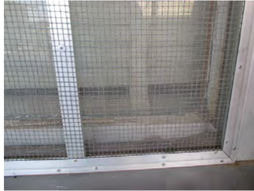
Roberts ES - Main Building Window
