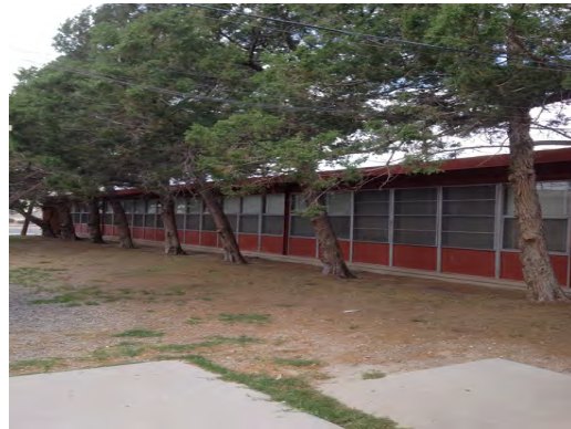
Stanton ES - Windows General Condition
