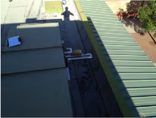
Aoy ES - Kitchen Roof Condition
