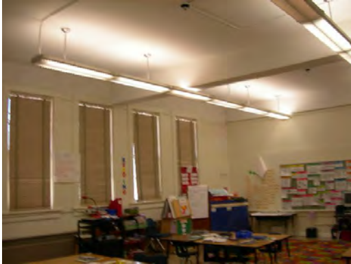
Alta Vista ES- Typical Ceiling
