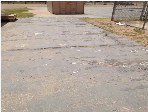
Stanton ES - Damaged Pedestrian Paving
