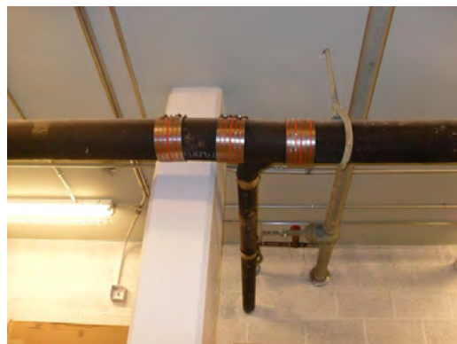
Armendariz MS - Sewer Lines
