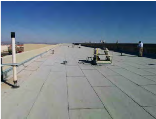
Hornedo MS - Roof General Condition
