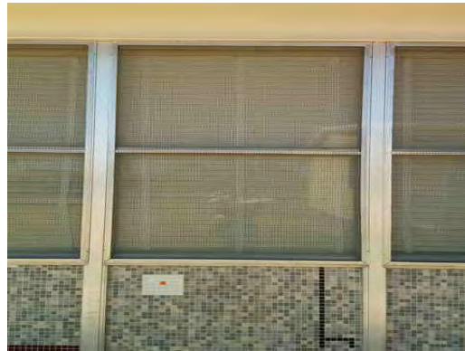
Dowell ES - Mismatched Tile at Window
