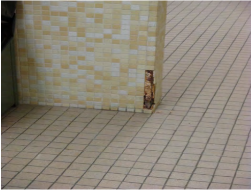
Roberts ES - Damaged Interior Tile Wall
