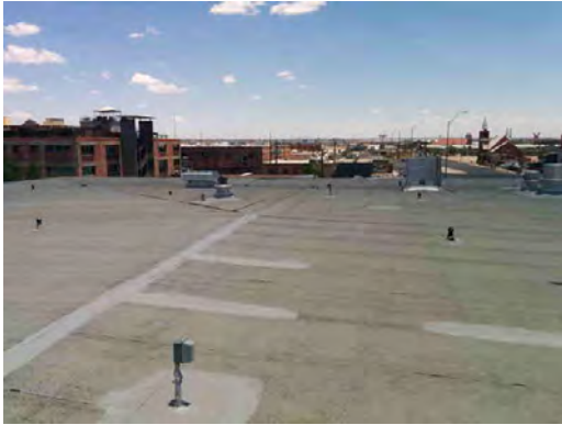
Telles Academy HS - Roof General Condition
