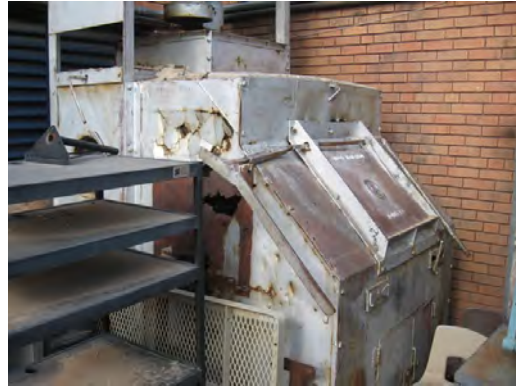
Dowell ES - Abandoned Incinerator in Mechanical Yard
