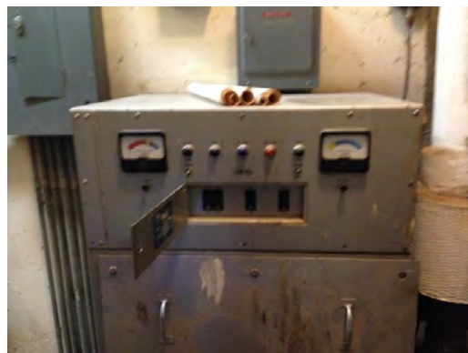
Clendenin ES - Electrical Equipment
