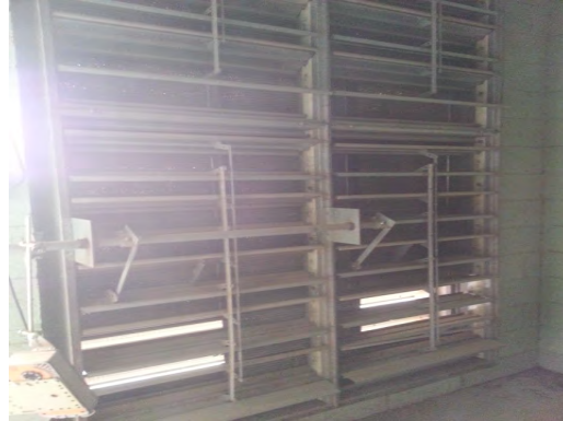
Cielo Vista - Non Working Damper at Room Evap
