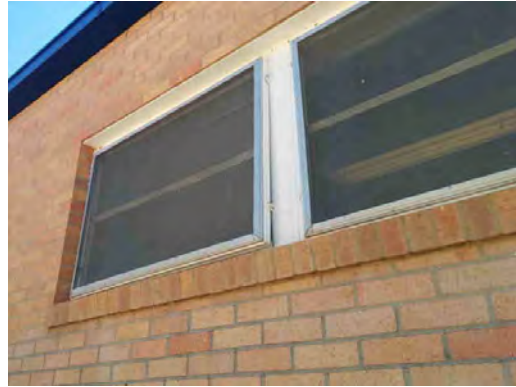
Irvin HS - Damaged Windows
