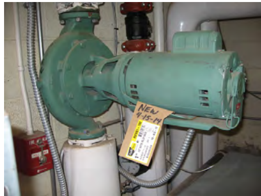
Schuster ES - Boiler Water Circulation Pump
