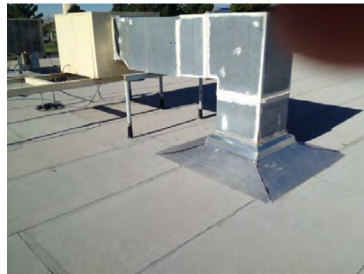
Burleson ES - Roof General Condition 01
