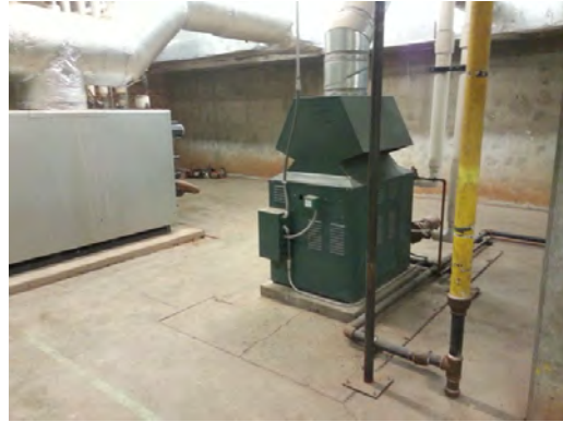
Burgess - Hot Water Boiler
