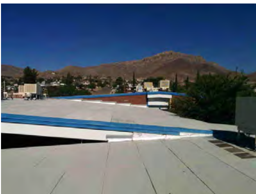
Park ES - Roof General Condition
