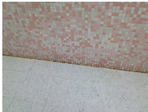
Morehead MS - Damaged Tile Wall
