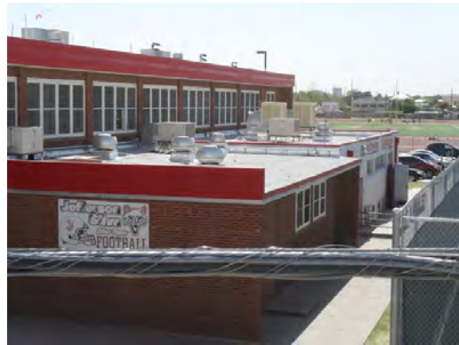
Jefferson HS - Locker Room Rooftop Equipment
