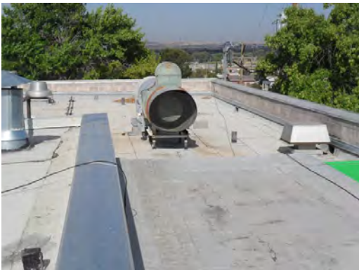
Roberts ES - Kitchen Roof Exhaust
