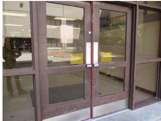
Franklin 9th Grade Center - Aged Exterior Metal Doors
