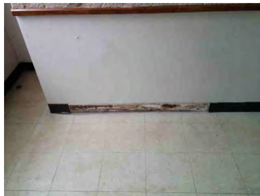
Guillen MS - Damaged Cove Base
