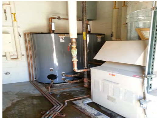
Green ES - Twin Water Storage Tanks
