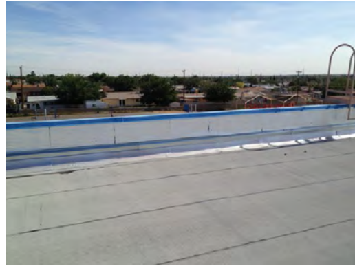
Collins ES - Roof General Condition 02
