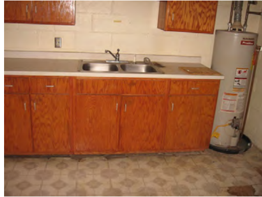
Dowell ES - Kitchen and Water Heater in Custodian Quarters
