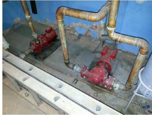
Alta Vista ES- Domestic Hot Water Pumps
