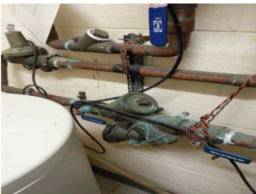
Green ES - Water Softener Backflow Preventer
