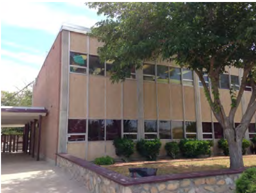
Address HS - Building 4 Rear Elevation
