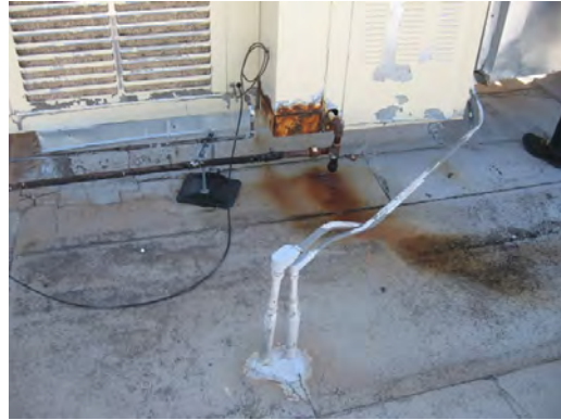
Schuster ES - Corrosion at Rooftop Unit
