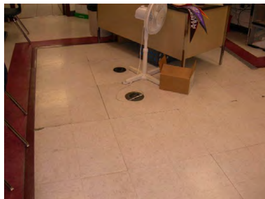
Chapin HS - Damaged VCT Flooring
