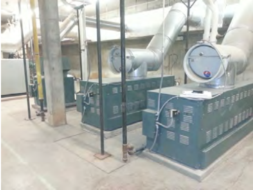
Burgess - Building 12 Heating Pumps
