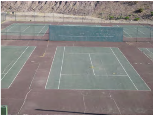
Franklin 9th Grade Center - Cracked and Weathered Paving at Play Areas
