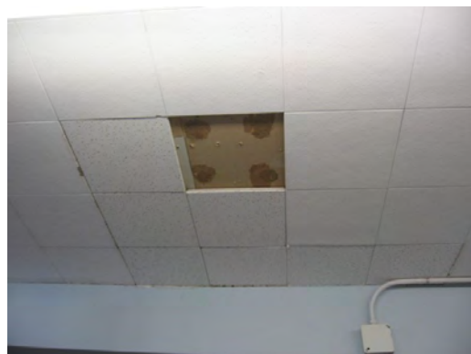
Schuster ES - Missing Ceiling Tile
