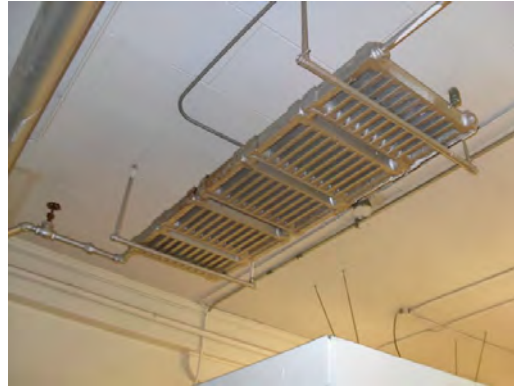
San Jacinto Auit - Radiant Heater
