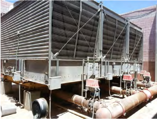
Chapin HS - Cooling Towers
