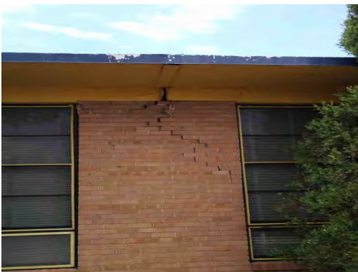
Hughey ES - Cracked Brick Wall
