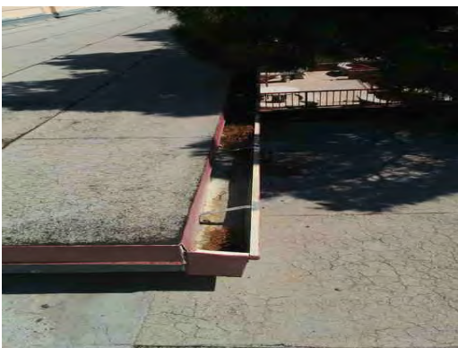
Travis ES - Debris in Gutter
