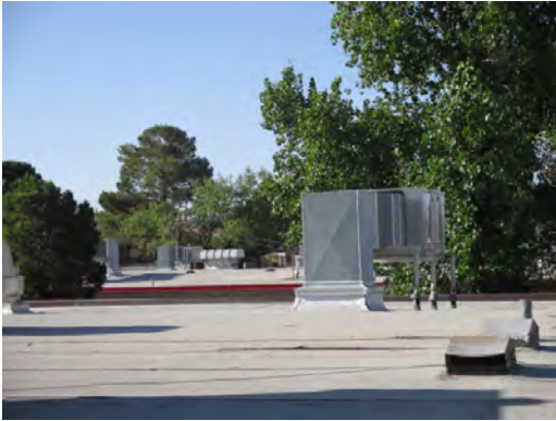
Polk ES - Rooftop Equipment 03
