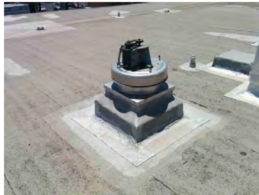
Telles Academy HS - Damaged Roof Exhaust Fan
