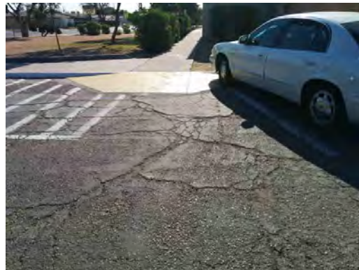
Bonham ES - Cracked and Worn Asphalt Paving 02
