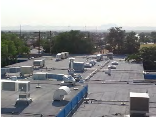
Collins ES - Rooftop Equipment 05
