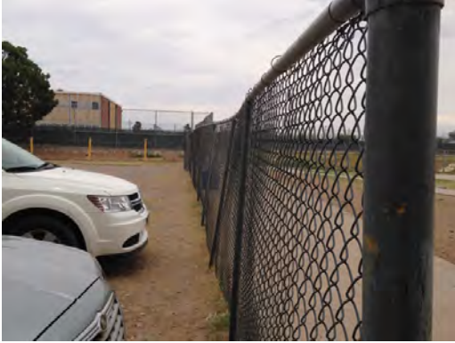
Address HS - Damaged Chain Link Fence
