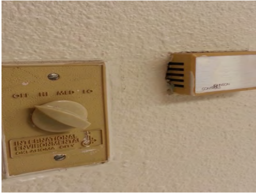
Burleson ES - Heating Controls
