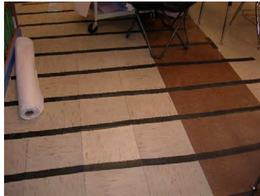
Bradley ES - Damaged VCT Flooring
