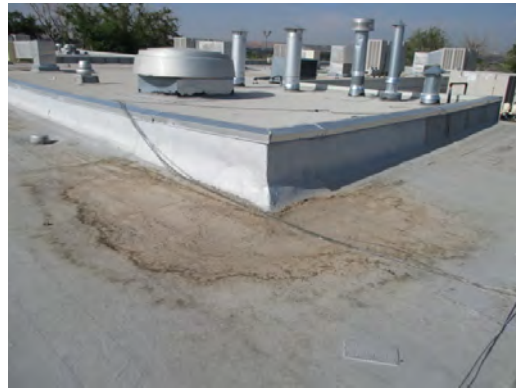
Roberts ES - Evidence of Ponding on Roof
