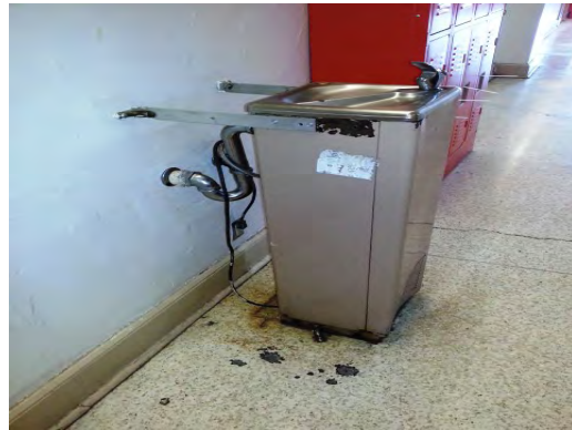
El Paso HS - Damaged Drinking Fountain
