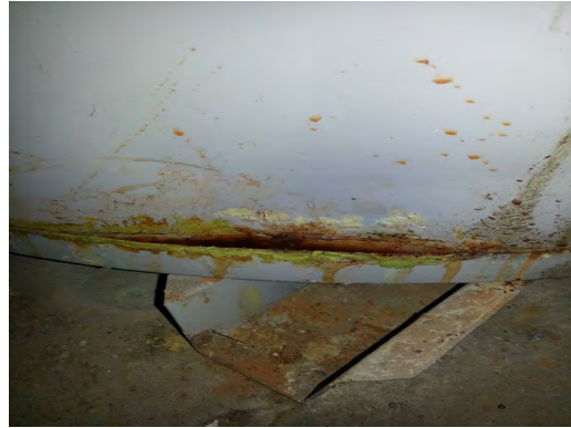
Burleson ES - Damaged Hot Water Boiler
