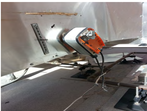
Rusk ES - Dislodged Dmaper Motor on Duct 02
