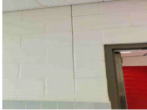
Magoffin MS - Cracked Interior CMU Wall
