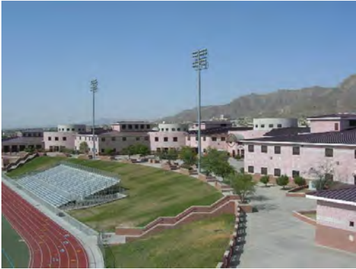
Chapin HS - Rear Elevation 03
