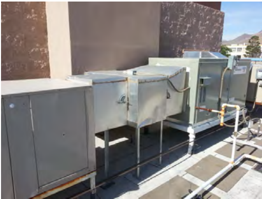
Collins ES - Gym Evap-Heater Combo
