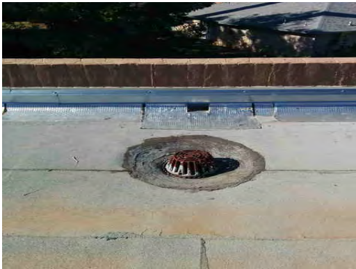
Barron ES - Roof Drain 01
