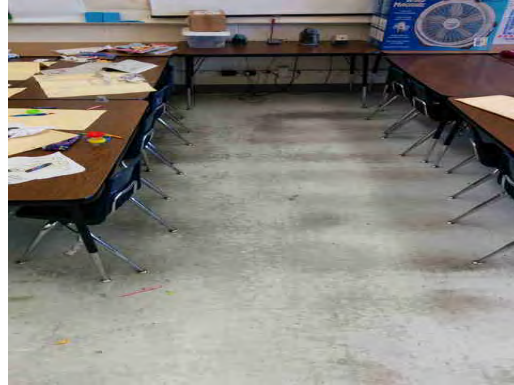
Bliss ES - Worn Flooring
