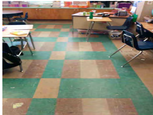
Park ES - Worn VCT Flooring
