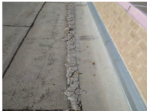
Cooley ES - Roof Flashing
