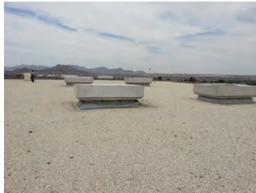
Coronado HS - Building 4 Roof Exhaust
