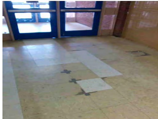
Lee ES - Damaged VCT Flooring 02
