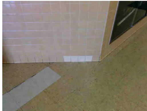
Lee ES - Mismatched Tile Repair
