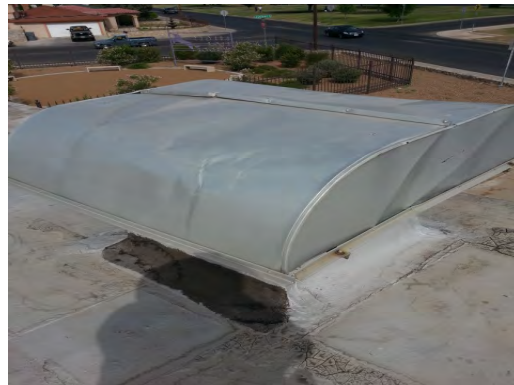
Burgess - Damaged Vent Housing
