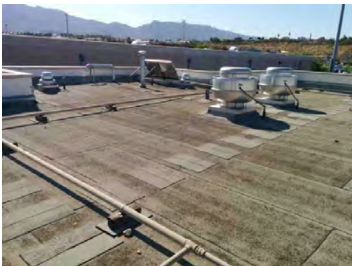
Franklin HS - Exhaust Fans
