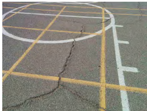
Hillside ES - Cracked Asphalt Paving
