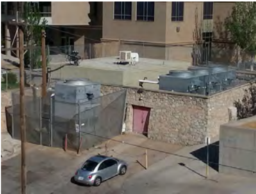
El Paso HS - Mechanical Building
