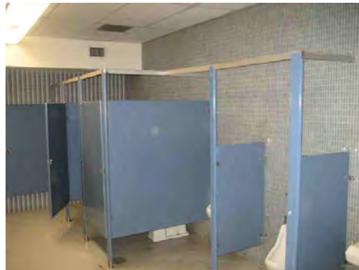
Crosby ES - Restroom Fixtures and Finishes 02
