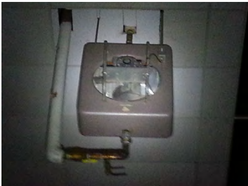
MacArthur ES MS - Unit Heaters in Gym
