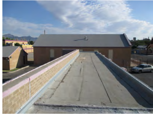
Cooley ES - Roof General Condition 02
