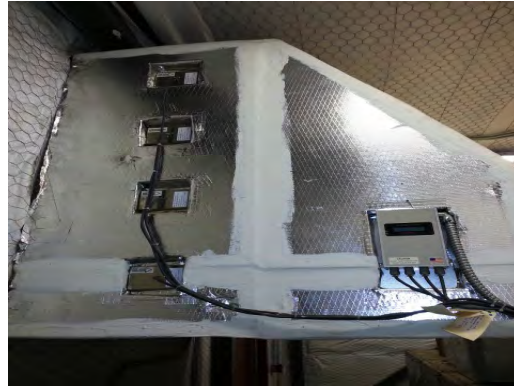
MacArthur ES MS - Intake Sensor in Rooftop AHU
