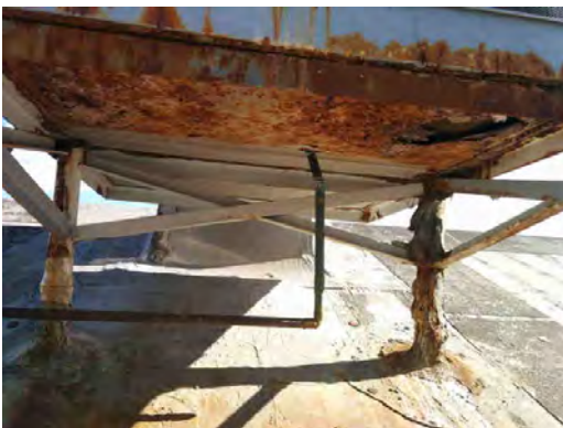
Hillside ES - Corroded Rooftop Equipment
