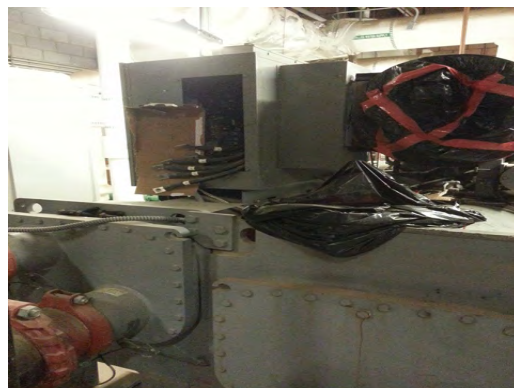
Chapin HS - Chiller Offline for Repair
