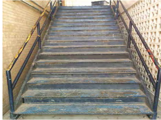
Irvin HS - Weathered Metal Stairs
