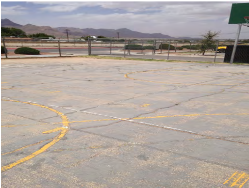
Stanton ES - Weathered, Cracked Paved Play Areas
