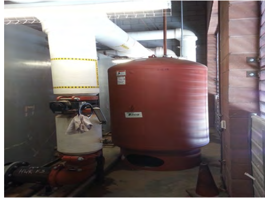
Chapin HS - Exp Tank
