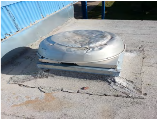
Collins ES - Damaged Exhaust fan
