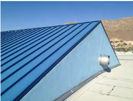
Clendenin ES - Roof Condition 03
