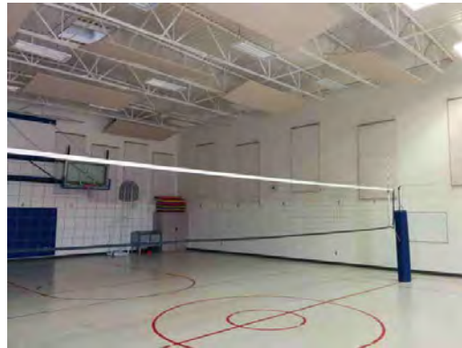
Hillside ES - Exposed Ceiling in Gym
