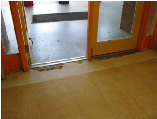
Roberts ES - Damaged VCT at Entry
