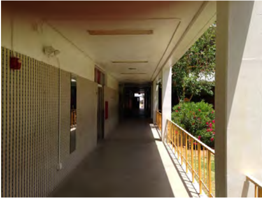
Terrace Hills MS - Exterior Covered Corridor
