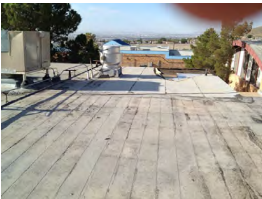
Bassett MS - Worn Roof Condition
