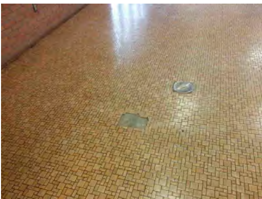
Irvin HS - Damaged Tile Flooring 02
