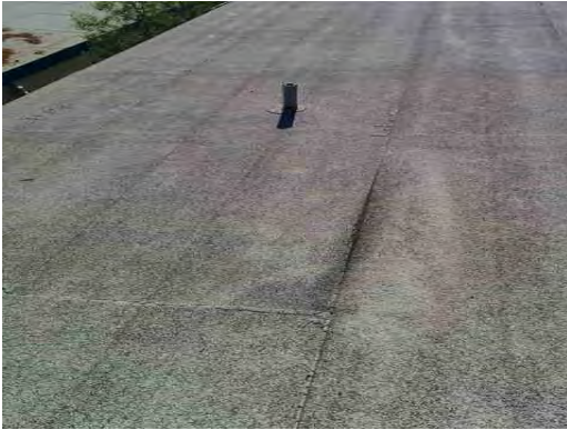
Park ES - Evidence of Ponding on Roof
