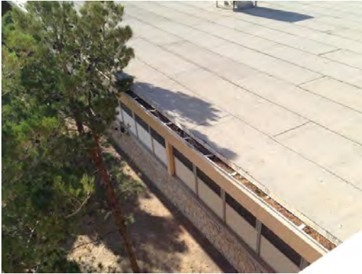
Crockett ES - Roof General Condition
