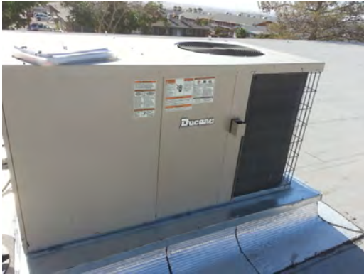
Clendenin ES - Furnace AC Combo Unit
