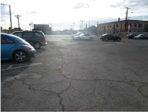
San Jacinto Auit - Cracked Asphalt Paving
