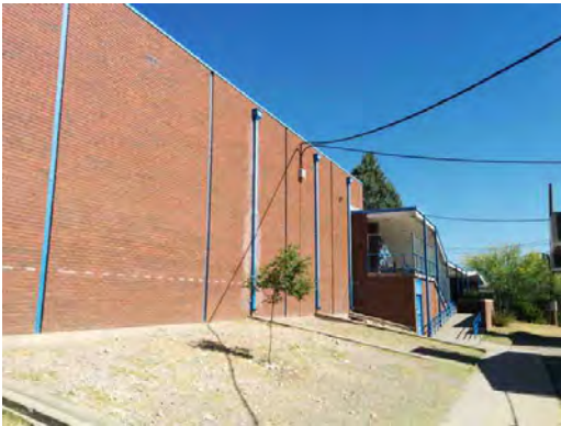
Park ES - Exterior Brick
