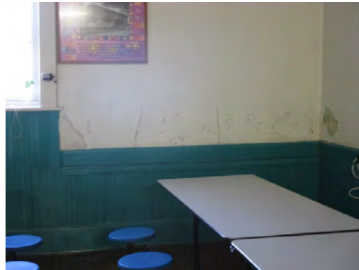
San Jacinto Auit - Damaged Interior Walls
