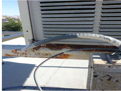
Burleson ES - Corroded Evap Cooler
