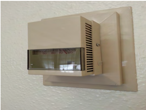
Rusk ES - Pneumatic Thermostat
