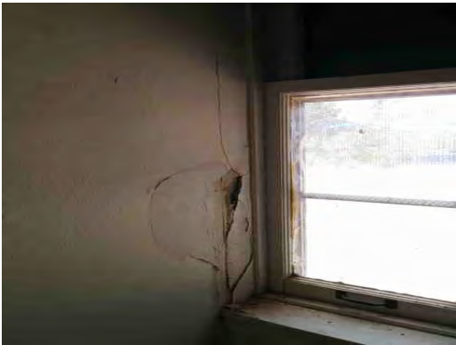
Hawkins ES - Damaged Interior Wall 02
