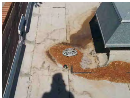
Lee ES - Debris at Roof Drain
