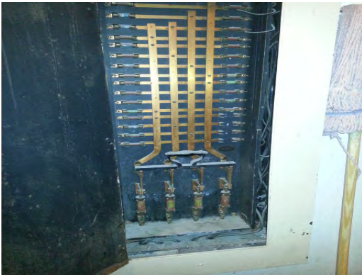
El Paso HS - Unprotected and Exposed Electrical Buss Bar
