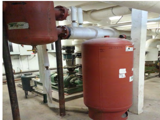
Aoy ES - Exp Tank and Separator
