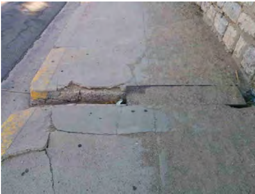
El Paso HS - Damaged Pedestrian Paving
