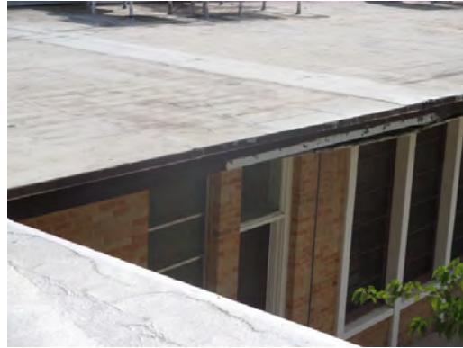
Clardy ES - Roof Condition
