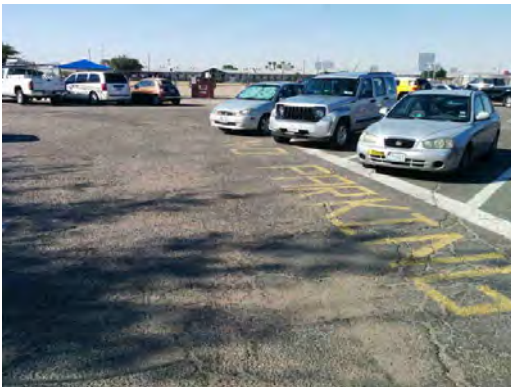
Bonham ES - Cracked and Worn Asphalt Paving 01
