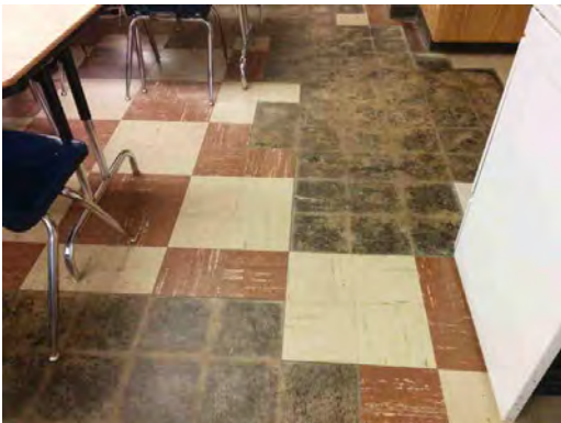
Irvin HS - Mismatched Tile Repair 03
