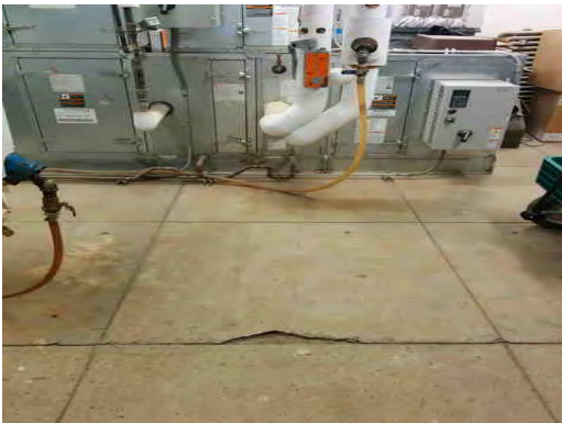
Vilas ES - Damaged Concrete Floor in Mechanical Room
