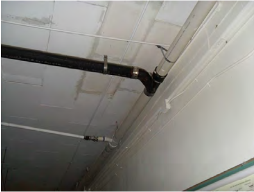
San Jacinto Auit - Sewer Line
