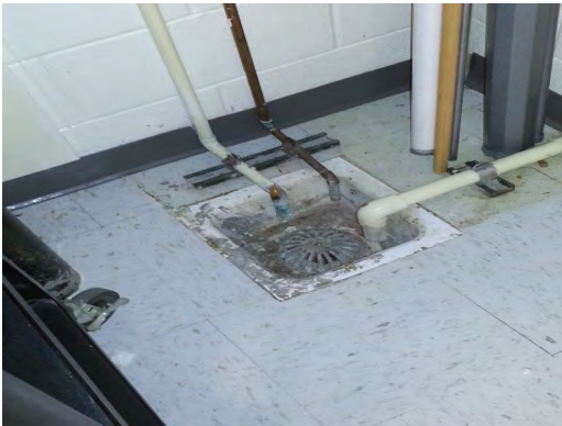
MacArthur ES MS - Floor Drain
