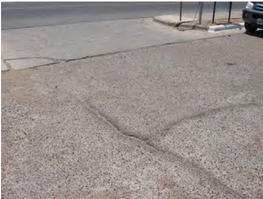
Schuster ES - Cracked Paving
