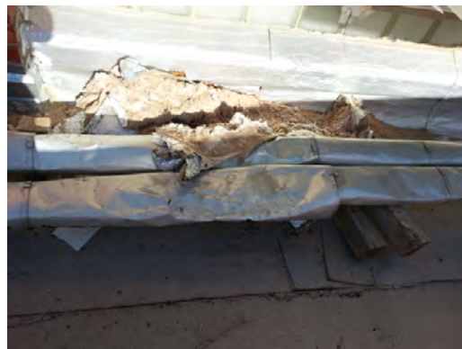
Milam ES - Damaged Insulation and Water Line Jacketing
