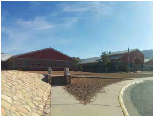
Tippin ES - Site Drainage Issues
