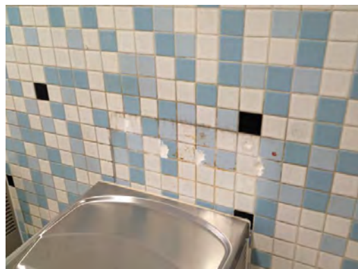
Collins ES - Damaged Tile Wall 01
