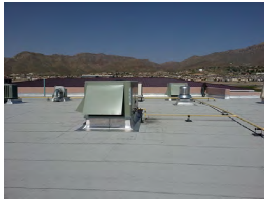
Chapin HS - Rooftop Equipment 02
