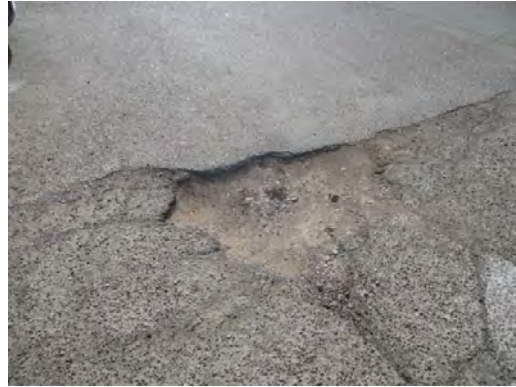
San Jacinto Auit - Damaged Asphalt Paving
