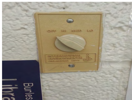
Burleson ES - Unit Heater Switch
