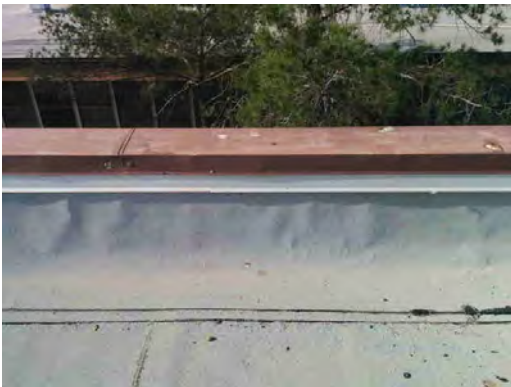
Hawkins ES - Bubbled Roofing Material
