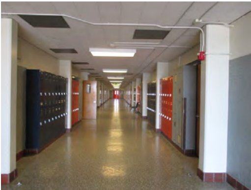
Henderson MS - Hallway Finishes
