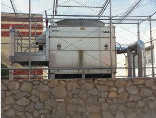
Coronado HS - Cooling Tower
