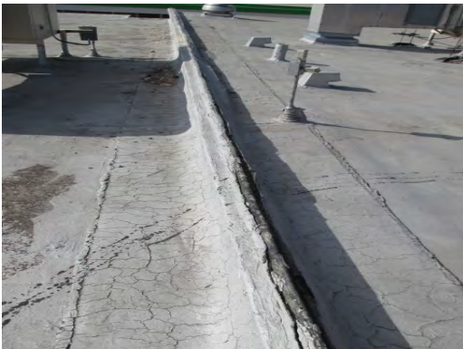
Roberts ES - Expansion Joint
