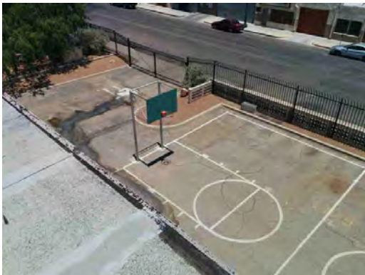
Telles Academy HS - Damaged Paving at Play Area
