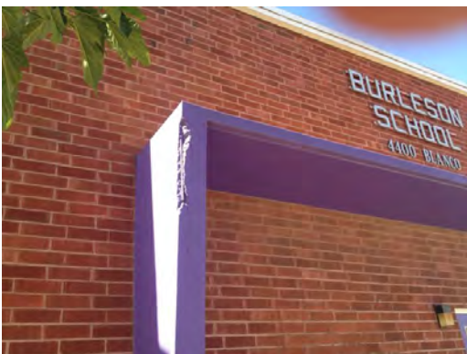
Burleson ES - Cracked Awning
