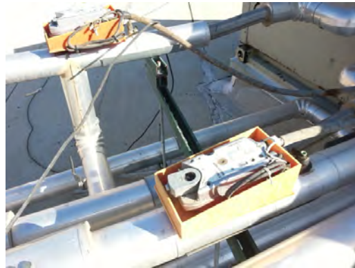
El Paso HS - Missing Valve Actuator Covers
