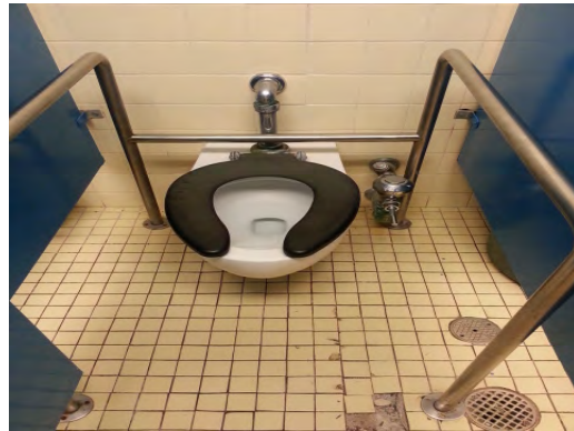
Collins ES - Damaged Foot Valve at Toilet 01
