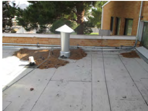
Clardy ES - Debris on Roof
