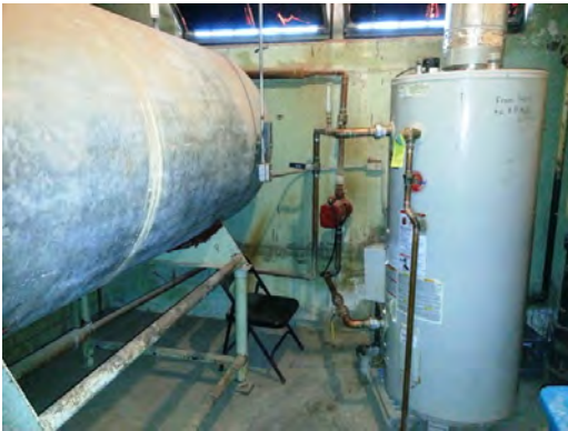
El Paso HS - Field House Mechanical Room
