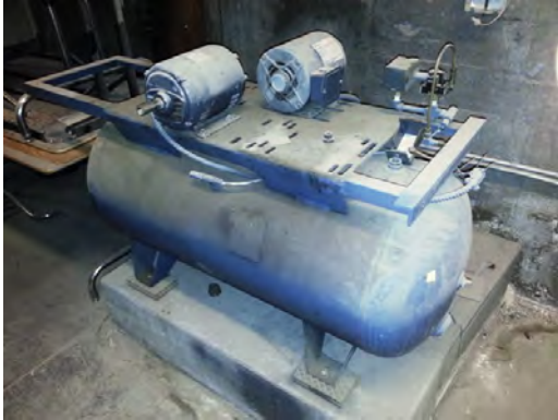
El Paso HS - Abandoned Air Compressor
