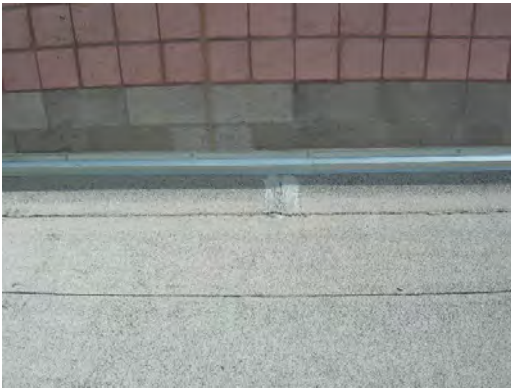
Chapin HS - Flashing Joint
