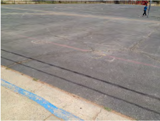
Collins ES - Cracks in Paved Area
