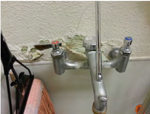
Green ES - Damaged wall Due to Shortened Water Splash
