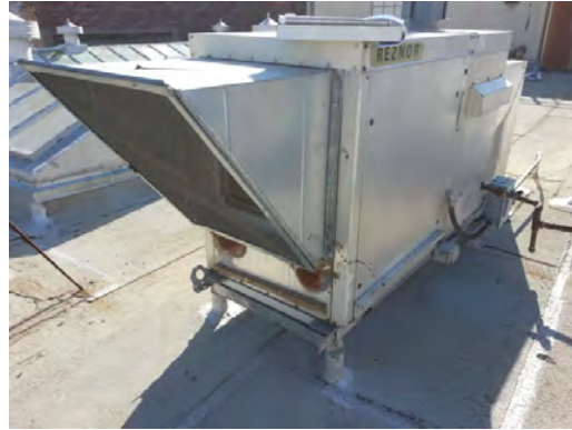
El Paso HS - MAU Main Building
