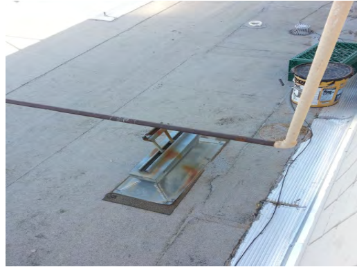
Green ES - Missing Tie Down Pipe Strap
