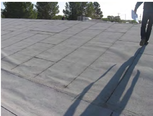
Schuster ES - Bubbled Roofing Material
