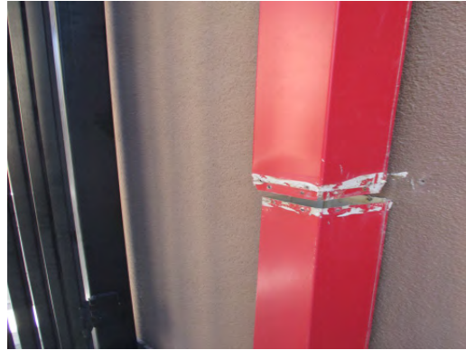
Polk ES - Damaged Downspout
