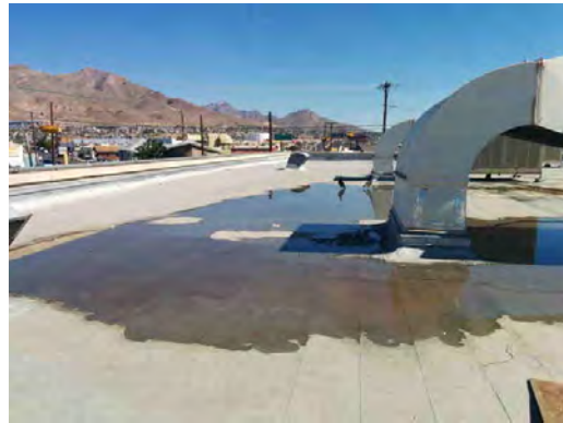
Beall ES - Ponding on Roof 01
