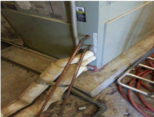
Alta Vista ES Missing Insulation
