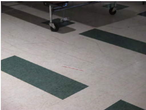
Kohlberg ES - Damaged VCT Flooring
