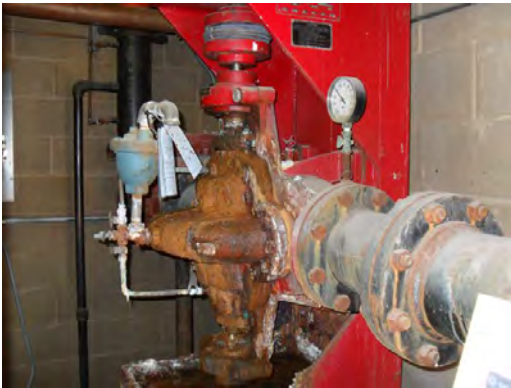
Silva Health Magnet HS - Corroded Fire Pump
