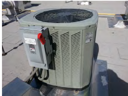
Chapin HS - Condenser
