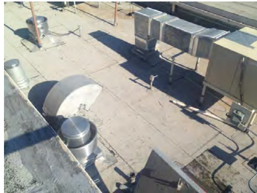
Burnet ES - Rooftop Equipment
