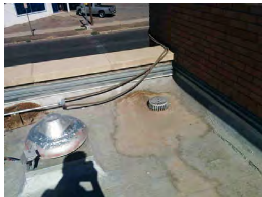
Beall ES - Evidence of Ponding on Roof Around Drain
