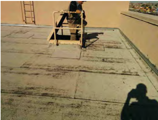
Bowie HS - Weathered Roof
