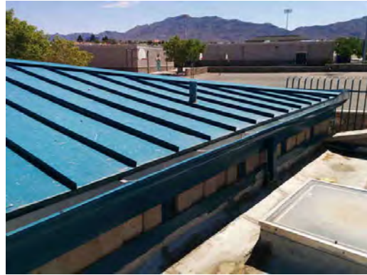
Franklin HS - Metal Roof
