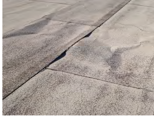
Lincoln MS - Bubbled Roofing Material
