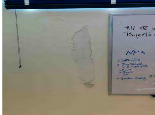
Bowie HS - Damaged Interior Wall 01
