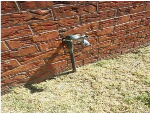
Bradley ES - Insulated Piping 01
