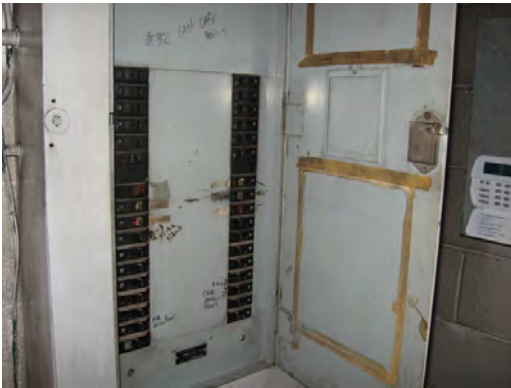
Dowell ES - Aged and Obsolete Electrical Panels
