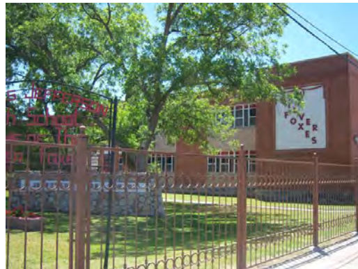
Jefferson HS - Building 1 Exterior
