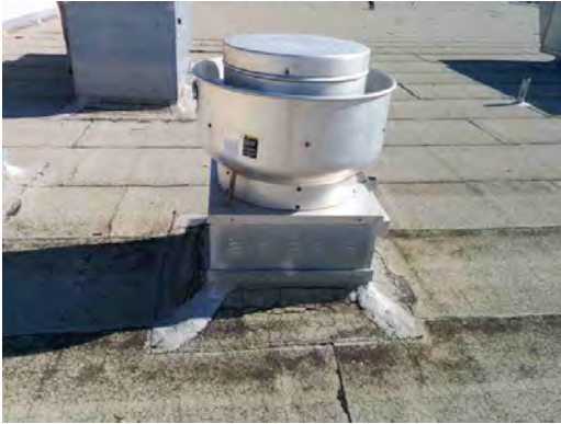
Center for Career & Tech - Exhaust Fan
