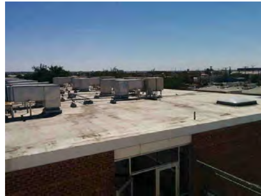
Douglass ES - Worn Roofing Materials 02
