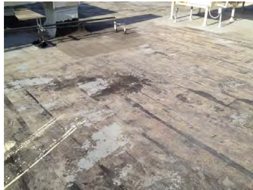
Rusk ES - Weathered Roof Material
