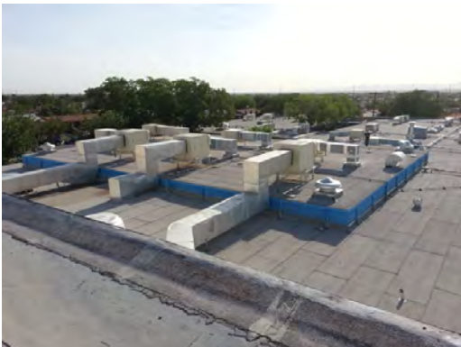
Collins ES - Rooftop Equipment 03
