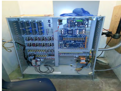
Rusk ES - Elevator Controls
