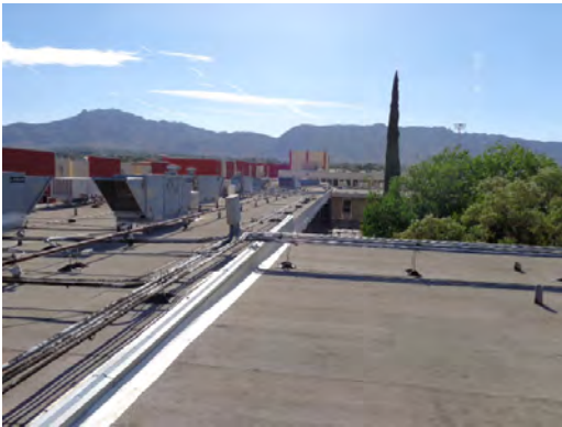
Coronado HS - Rooftop Equipment 02
