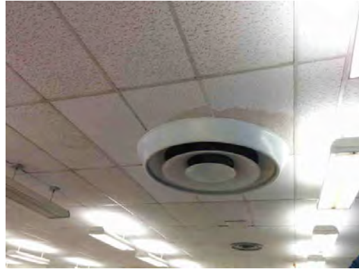
Park ES - Stained Ceiling Tiles
