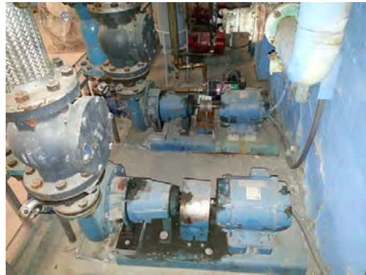
Alta Vista ES - Water Heating Pump
