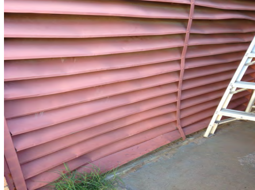
Stanton ES - Damaged Louvre
