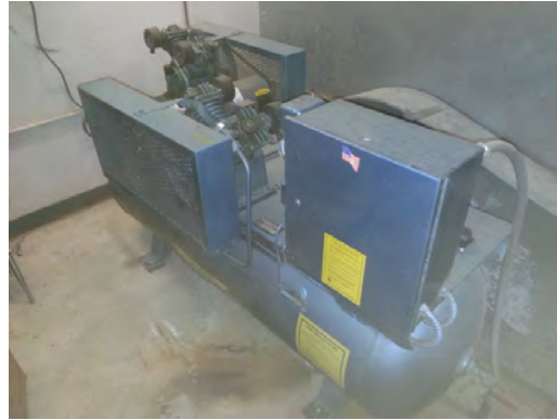
Clendenin ES - Pneumatic air Compressor
