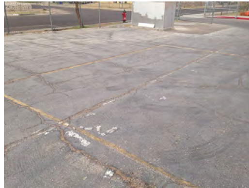
Terrace Hills MS - Weathered Asphalt Paving
