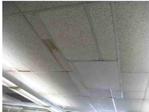
Crosby ES - Damaged Ceiling Tiles 02
