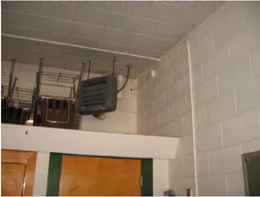
Dowell ES - Typical Hot Water Unit Heater
