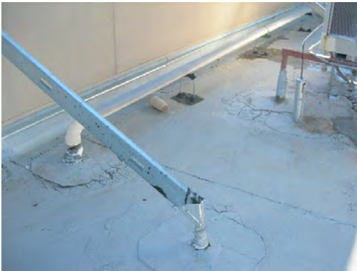
Brown MS - Weathered Parapet Roof 02
