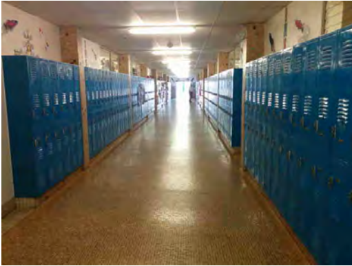
Irvin HS - Hallway Finishes
