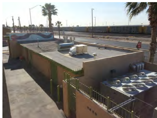
Aoy ES - Mech Building
