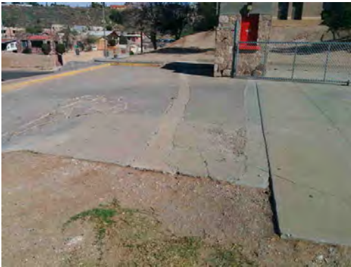
El Paso HS - Damaged Concrete Paving
