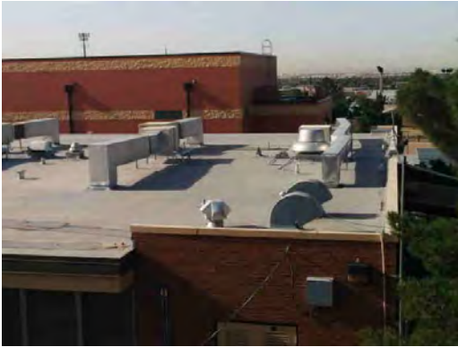
Hawkins ES - Rooftop Equipment 01
