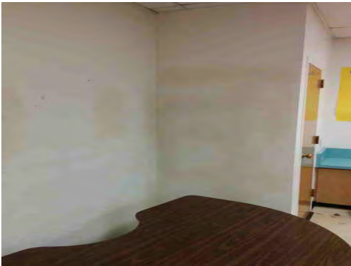
Bliss ES - Damaged Interior Wall
