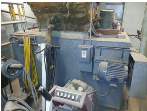
MacArthur ES MS - Dated AHU in Gym Windows
