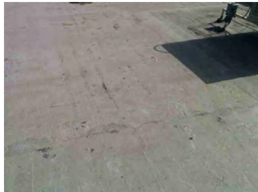
Vilas ES - Roof General Condition
