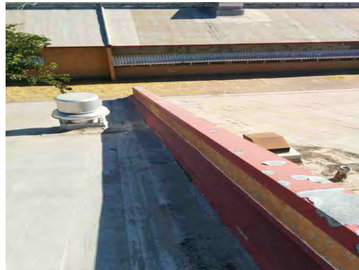
Hillside ES - Weathered Roofing 01
