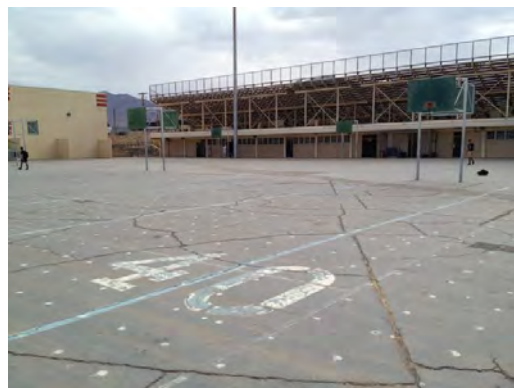
Coronado HS - Damaged Asphalt Play Area
