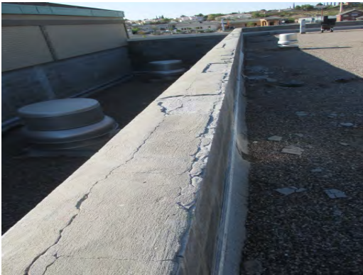
Franklin 9th Grade Center - Weathered Coping
