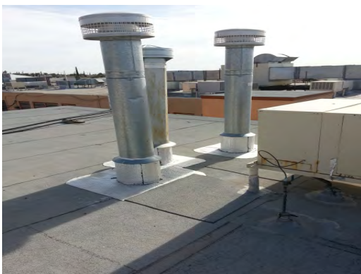
Rusk ES - Boiler Room Vent Stacks
