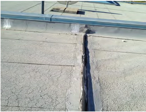
Clendenin ES - Roof Condition 01
