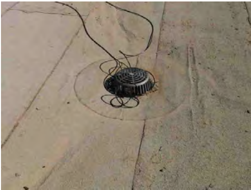
Irvin HS - Roof Drain
