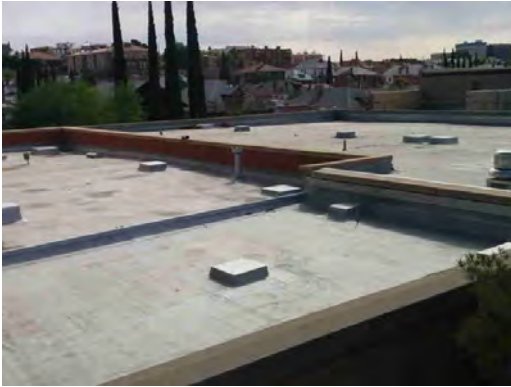
Vilas ES - Roof General Condition 02
