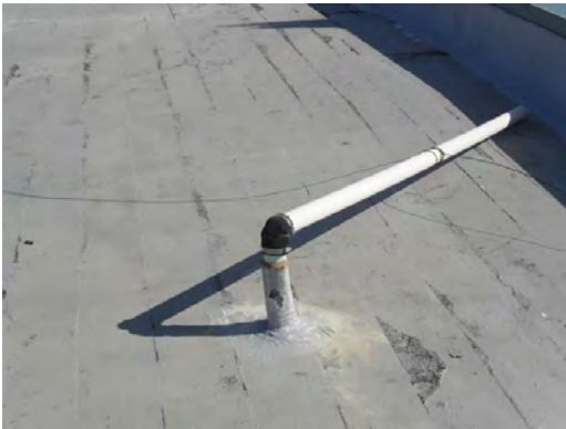
Kohlberg ES - Improper Vent on Roof
