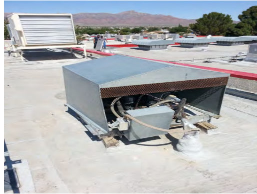
Bradley ES - Damaged Condenser Requires Replacement 02
