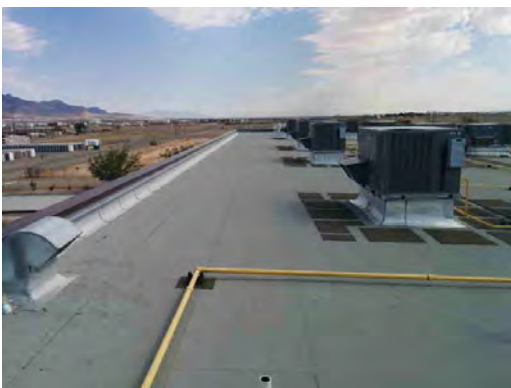
Hughey ES - Rooftop Units
