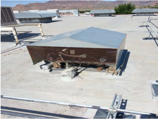
Bradley ES - Damaged Condenser Requires Replacement 01
