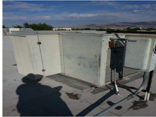
Burgess - Ac Coil Combo Unit
