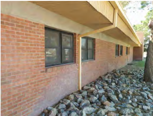
Lee ES - Exterior Brick Needs Cleaning
