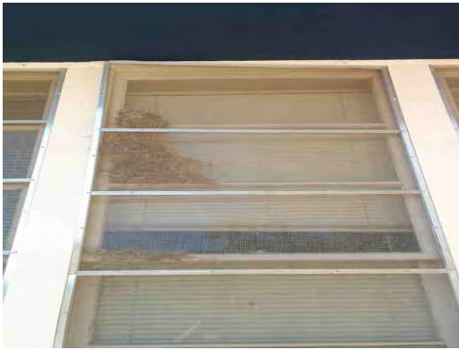
Bonham ES - Typical Windows
