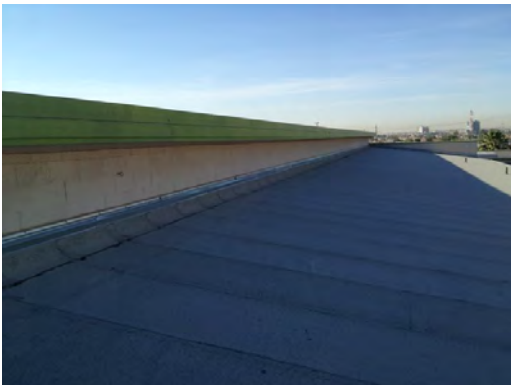
Aoy ES - Roofing General Condition 01
