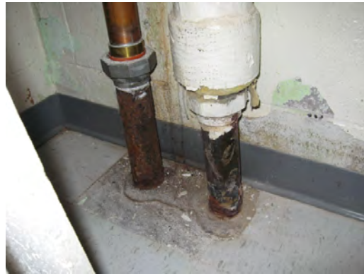
Schuster ES - Old to New Heating Water Connection
