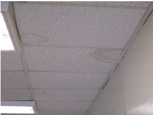
Roberts ES - Stained Ceiling Tiles
