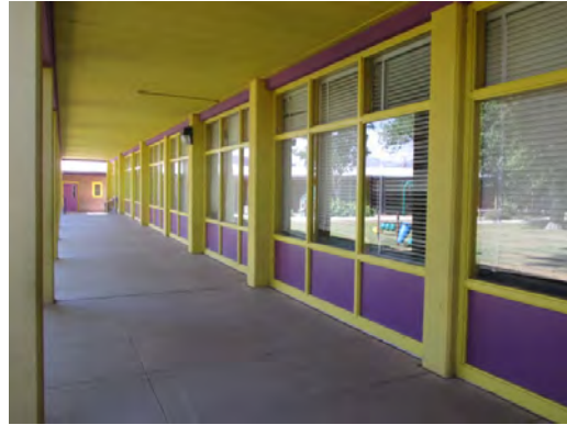
Cooley ES - Main Building Windows
