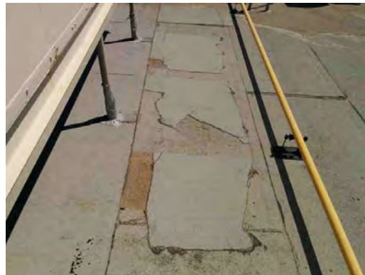
Hornedo MS - Damaged Roofing
