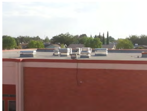
Cielo Vista - Arts building Roof
