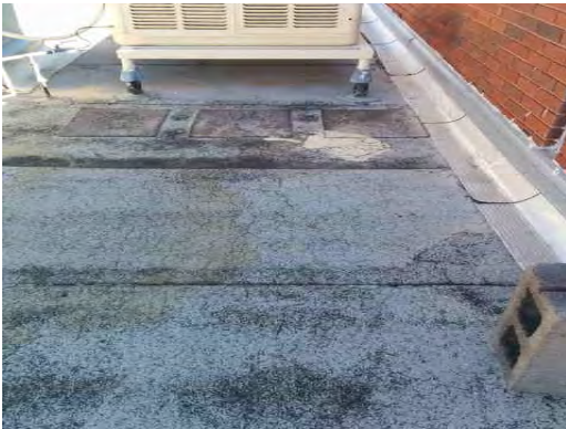
Park ES - Weathered Roofing
