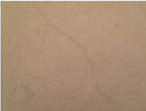
Rusk ES - Crack in Concrete Wall
