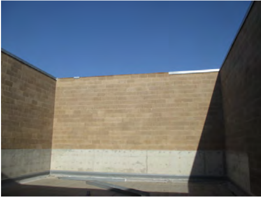
Silva Health Magnet HS - Missing Coping
