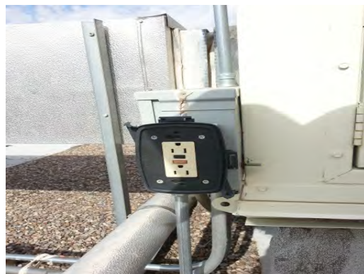
MacArthur ES MS - Replace AHU Electrical Outlet Cover
