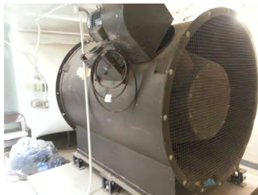
Clendenin ES - In Line Ventilation Fan
