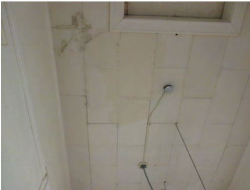
San Jacinto Auit - Damaged Interior Ceiling Tiles
