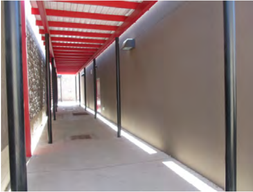
Polk ES - Covered Walkway
