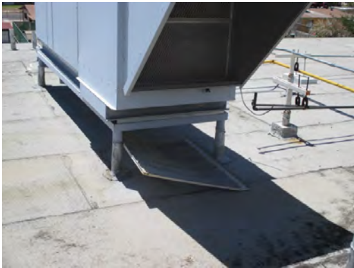
Henderson MS - Damaged Rooftop Unit
