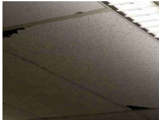
Barron ES - Damaged Ceiling Tiles 02
