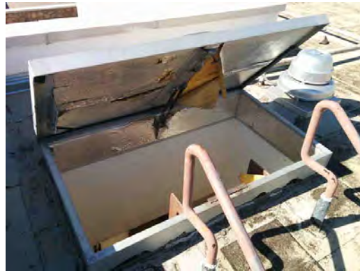
Franklin HS - Roof Hatch
