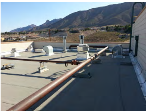
Green ES - Dining Rooftop Units
