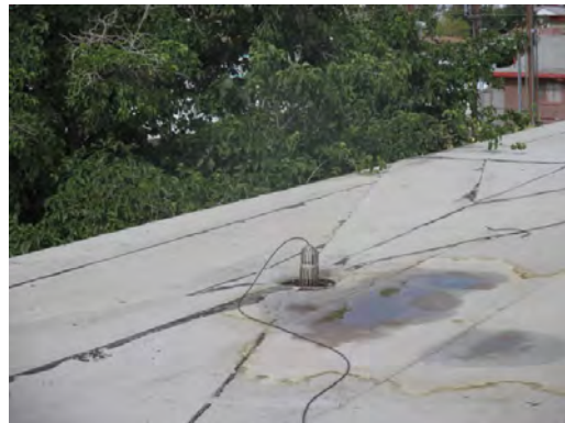
Clardy ES - Ponding on Roof
