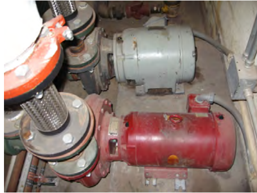
Schuster ES - Heating Water Circulation Pumps
