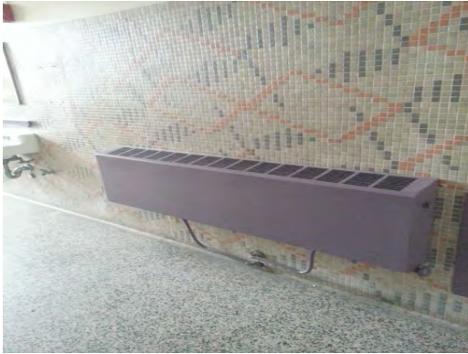
Burges - Typical Fin Tube Heater
