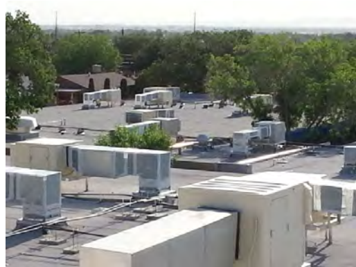
Collins ES - Rooftop Equipment 06
