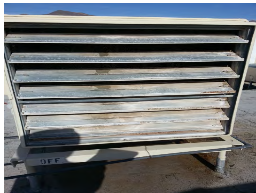
Collins ES - Weathered Evap Damper
