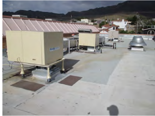
Canyon Hills MS - Rooftop Equipment 02
