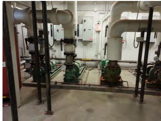
Aoy ES - Heating and Chilled Water Supply
