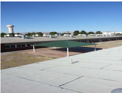
Burleson ES - Classroom Roof
