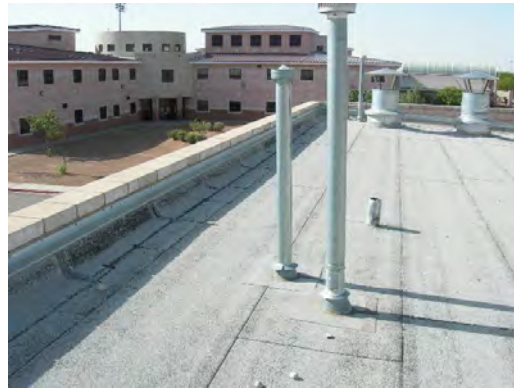
Chapin HS - Plant Roof
