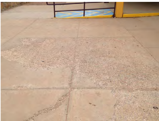
Address HS - Worn Pedestrian Paving
