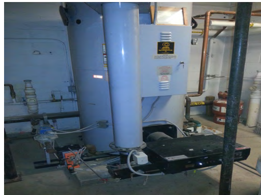
Aoy ES - Domestic Water Boiler
