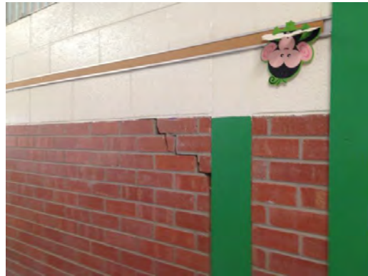
Burleson ES - Crack in Interior Wall
