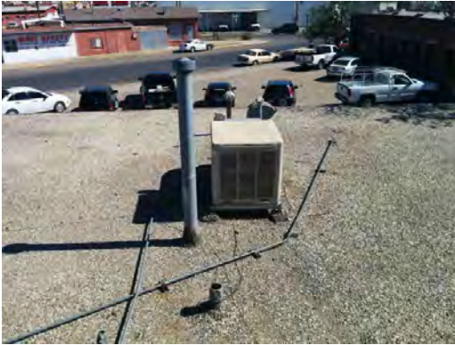
Beall ES - Rooftop Equipment
