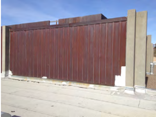
Johnson ES - Cafeteria High Wall at Roof
