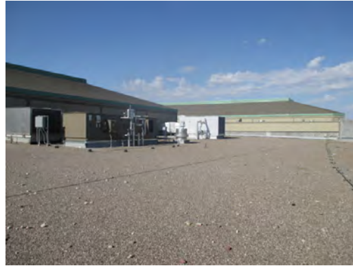
Franklin 9th Grade Center - Roof General Condition 02
