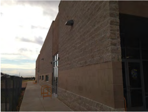
Terrace Hills MS - Exterior CMU Wall
