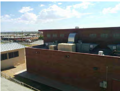
Travis ES - Rooftop Equipment
