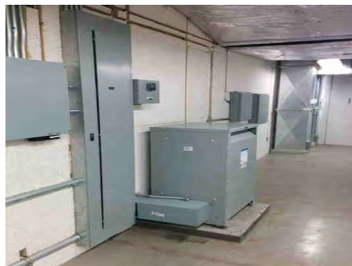
Hornedo MS - Electrical Equipment
