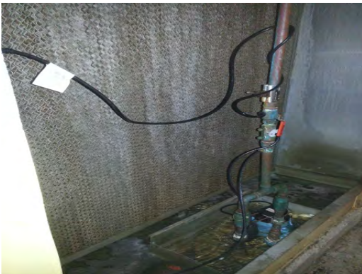
Cielo Vista - Room Evap Water Media Tray
