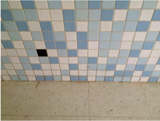
Collins ES - Damaged Tile Wall 02
