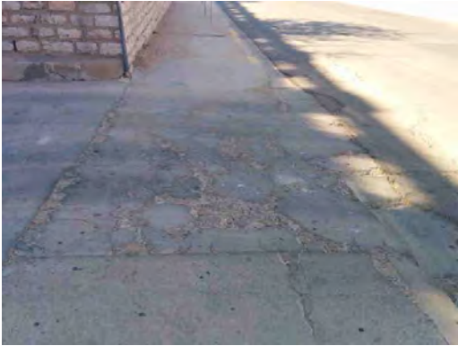
El Paso HS - Damaged Asphalt Paving
