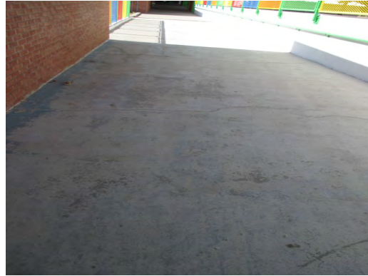
Roberts ES - Worn Epoxy Coated Walkway
