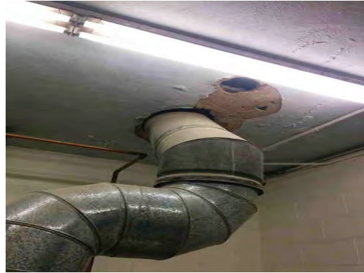
Bowie HS - Unsealed Penetration
