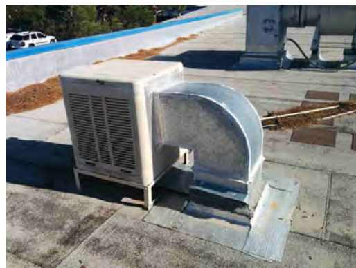
Park ES - Rooftop Equipment
