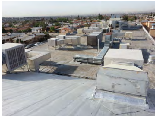
Rusk ES - Roof Top Equipment
