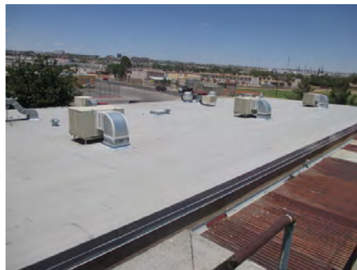
Henderson MS - Corroded Metal Panel Roof
