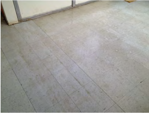
Collins ES - Worn VCT Flooring
