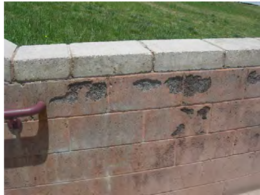
Chapin HS - Damaged Exterior Stair Wall
