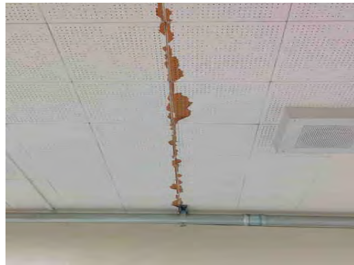
Hawkins ES - Damaged Adhered Tile Ceiling
