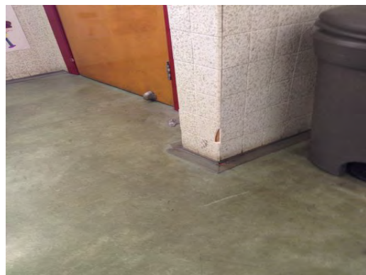
Rusk ES - Worn Hallway Floor
