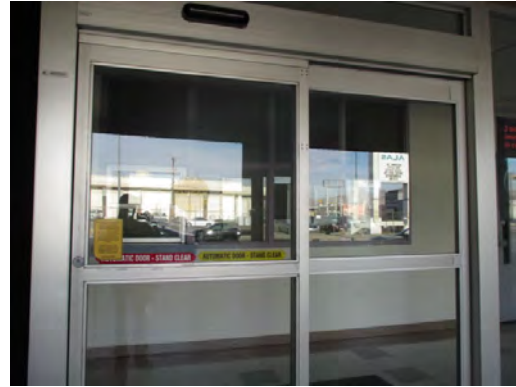
Telles Academy HS - Storefront Entry Doors
