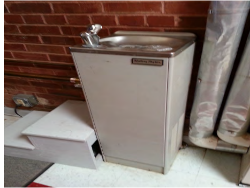
Milam ES - Dated Standing Water Fountain
