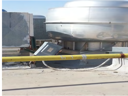
Crosby ES - Broken Disconnect Bracket
