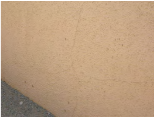
Putnam ES - Crack in Interior Wall
