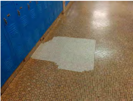
Irvin HS - Mismatched Tile Repair 01
