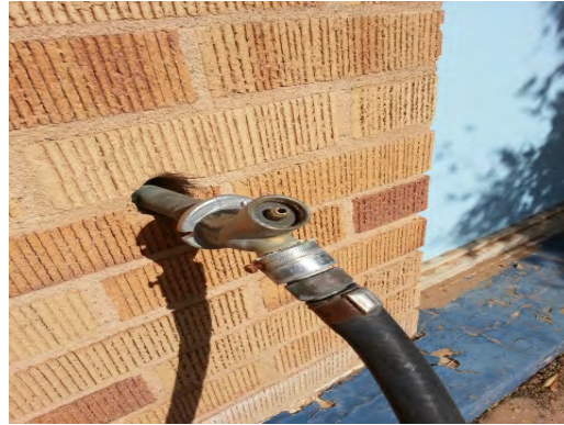
Clendenin ES - Broken Hose Bibb
