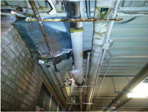
Burges - Multiple Repairs to Water Piping
