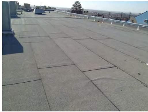
Clendenin ES - Roof Condition 02
