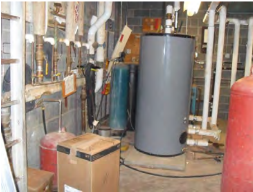
Newman ES - Mechanical Room 01
