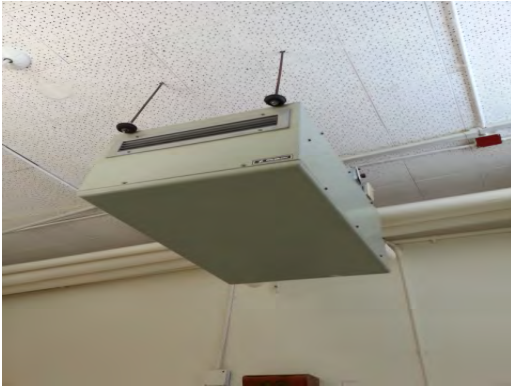
Milam ES - Typical Classroom Unit Heater
