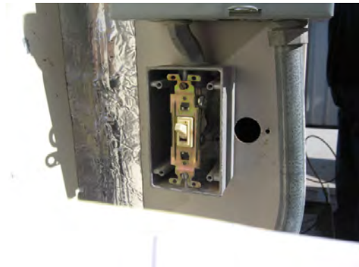
Schuster ES - Exposed Wiring
