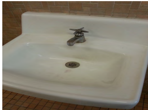
Crosby ES - Dated Plumbing Fixtures
