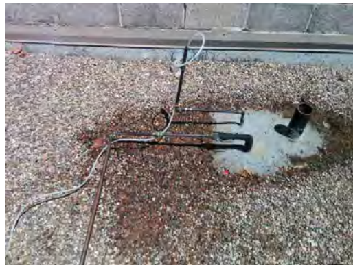
Magoffin MS - Evidence of Ponding on Roof
