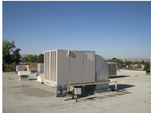
Polk ES - Rooftop Equipment 06
