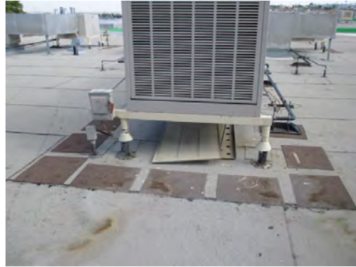
Roberts ES - Roof Debris
