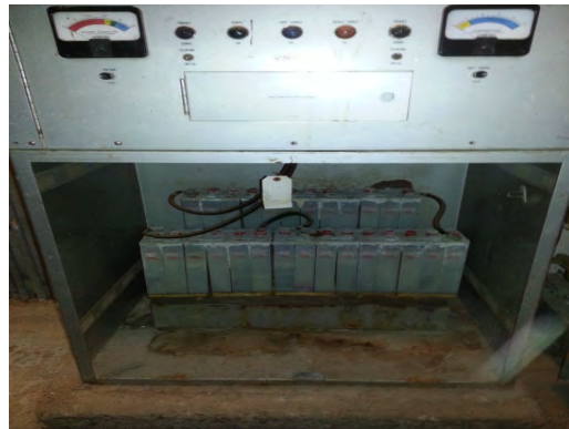
Clendenin ES - Aged Transformer
