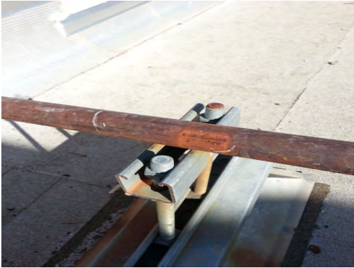
Green ES - Missing Gas pipe Tie Down Straps
