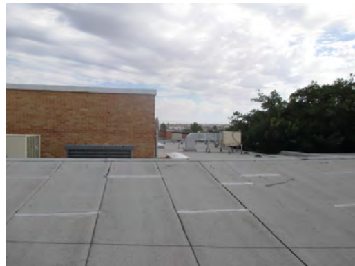
Clardy ES - Roof General Condition
