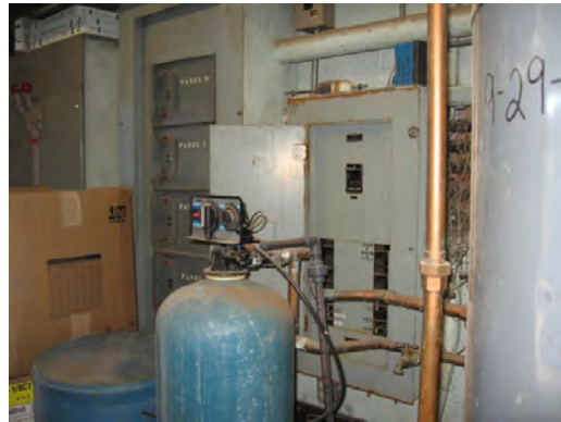
Dowell ES - Aged and Obsolete Electrical Switchgear
