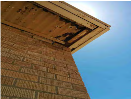
Magoffin MS - Damaged Soffit
