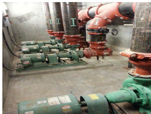
Chapin HS - Cooling Tower Pumps
