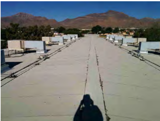
Dowell ES - Roof Condition
