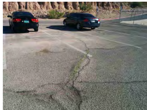
El Paso HS - Cracked Parking Lot Paving
