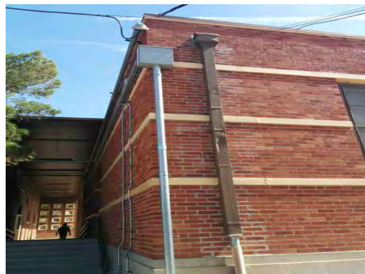
Hawkins ES - Damaged Downspout
