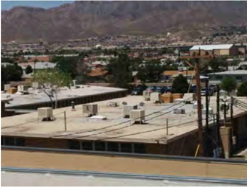
Magoffin MS - Rooftop Equipment
