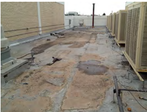
Morehead MS - Damaged Roofing, Evidence of Ponding
