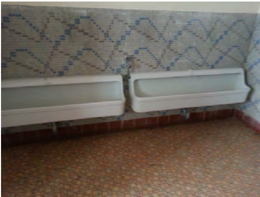
Burgess - Replace Trough Urinals
