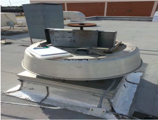
Burgess - Damaged Exhaust Fan
