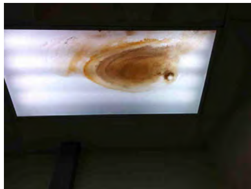
Barron ES - Damaged Light Cover
