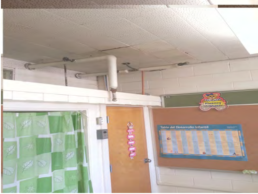
Burleson ES - Abandoned Unit Heater Piping
