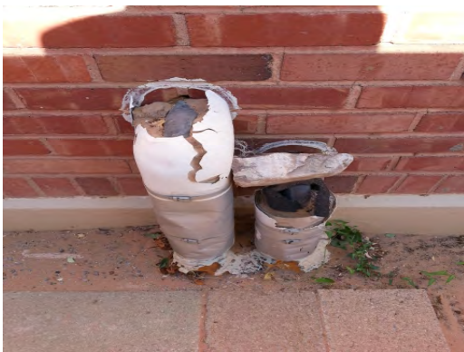
Milam ES - Damaged Insulation and Jacketing
