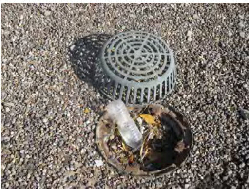
Franklin 9th Grade Center - Clogged Roof Drain
