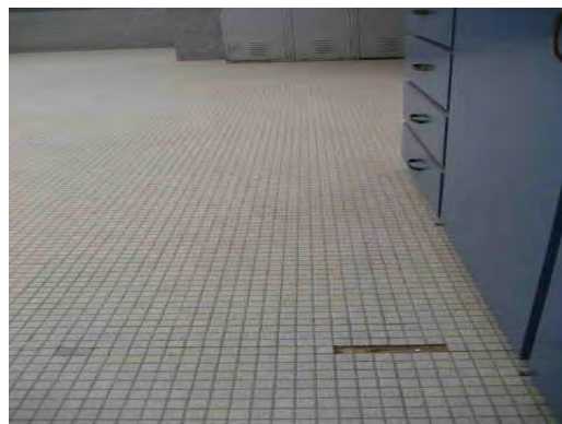
Crosby ES - Damaged Ceramic Tile Floor
