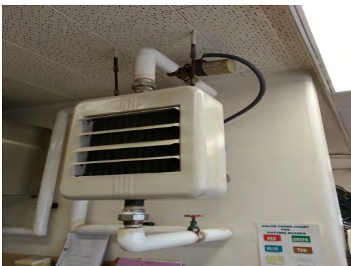
Milam ES - Kitchen Unit Heater
