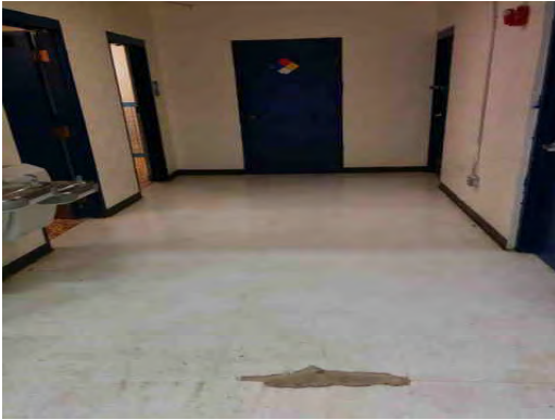
Irvin HS - Damaged VCT Flooring 02
