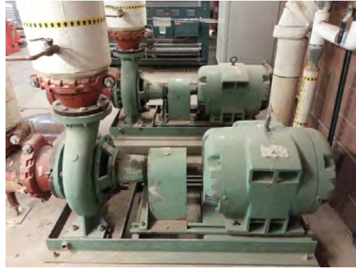
Chapin HS - Heating Water Supply Pumps
