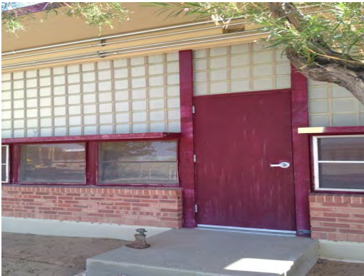
Milam ES - Typical Exterior Finish
