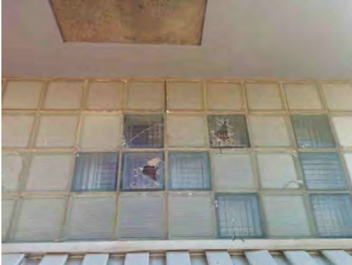
Hillside ES - Broken Glass Block Wall
