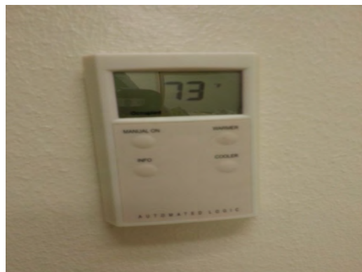
Cielo Vista - DDC Thermostat
