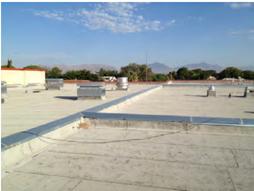
Cielo Vista - Roof General Condition
