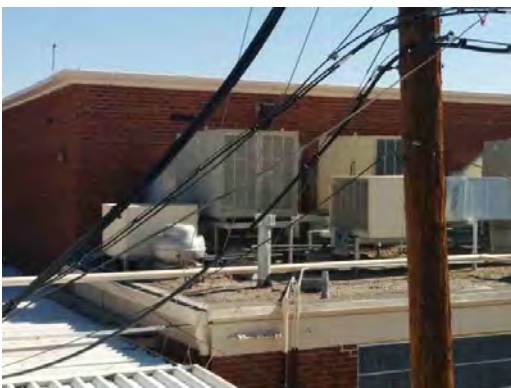
Wainwright ES - Rooftop Equipment
