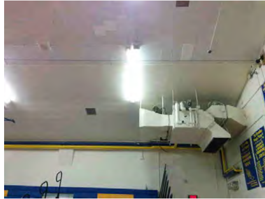
Armendariz MS - Gym HVAC
