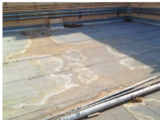
Rusk ES - Evidence of Ponding on Roof
