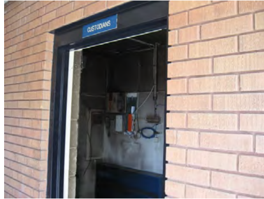
Dowell ES - Custodian Closet Condition After Trash Can Fire
