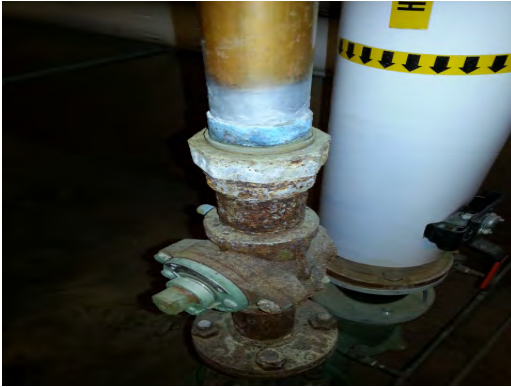
Milam ES - Leaking Water Pump
