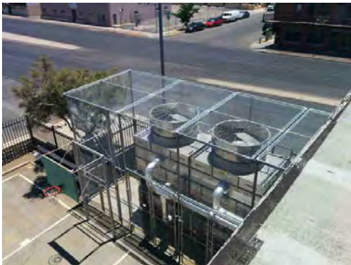
Telles Academy HS - Cooling Tower
