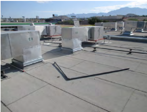
Roberts ES - Roof Debris
