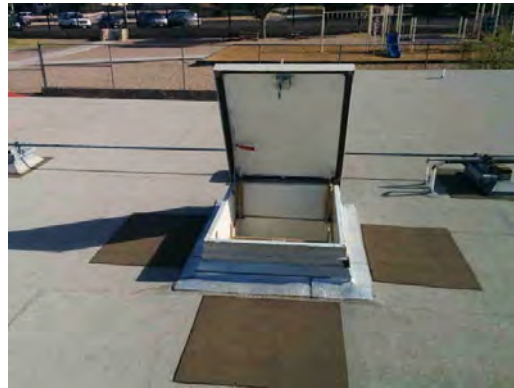
Hillside ES - Roof Hatch
