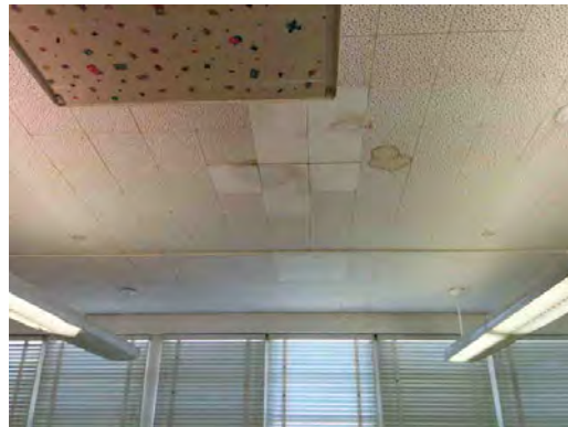
Wainwright ES - Damaged Ceiling Tiles
