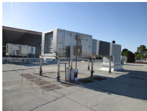
Polk ES - Rooftop Equipment 02
