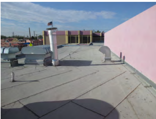
Cooley ES - Roof General Condition 01
