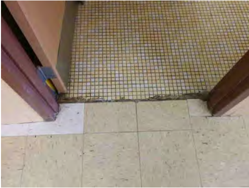
Lee ES - Damaged Ceramic Tile at Threshold
