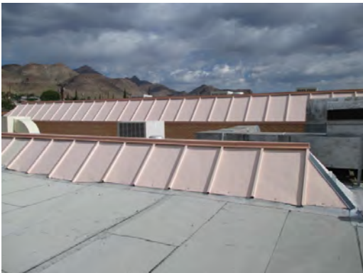
Canyon Hills MS - Roof General Condition
