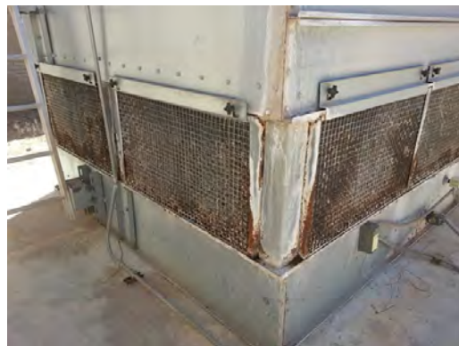
Brown MS - Corroded Tower Panels
