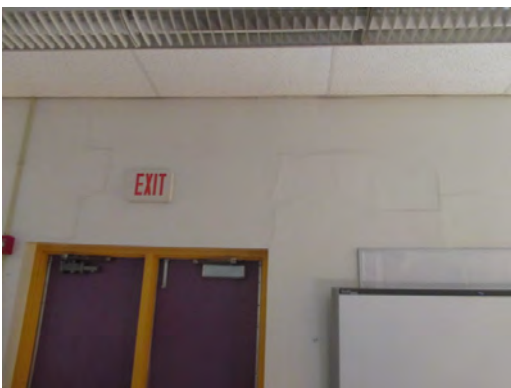
Cooley ES - Damaged Gypboard Wall
