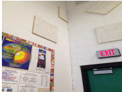
Aoy ES - Crack in Interior Wall 01
