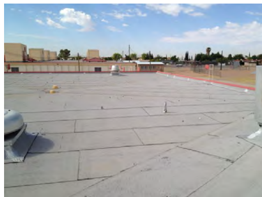
MacArthur ES MS - Gym Roof
