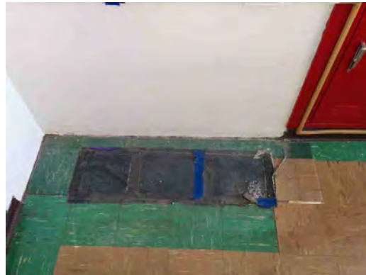
Bliss ES - Damaged VCT Flooring
