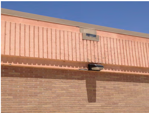
Lincoln MS - Building Mounted Lighting
