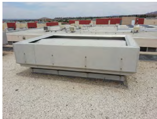
Coronado HS -Pneumatic Powered Exhaust Louvered Vents on Gym Roof
