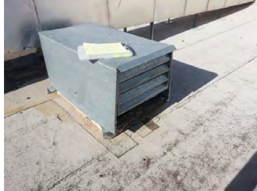
Collins ES - Aged and Weathered Freezer Condensers 02
