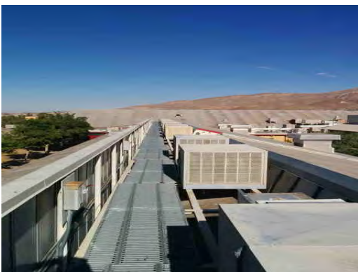
Hillside ES - Rooftop Equipment
