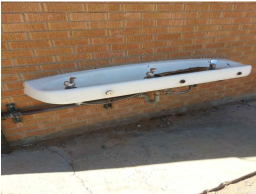
Crosby ES - Non-Operational Drinking Fountain
