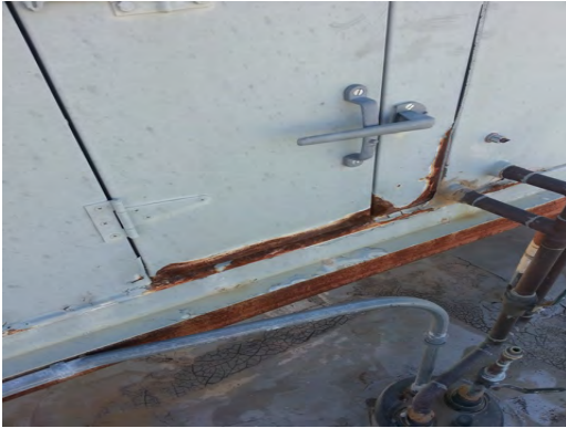
Crosby ES - Corroded Evap Unit
