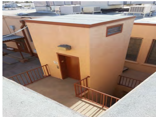
Rusk ES - Main Building Elevator
