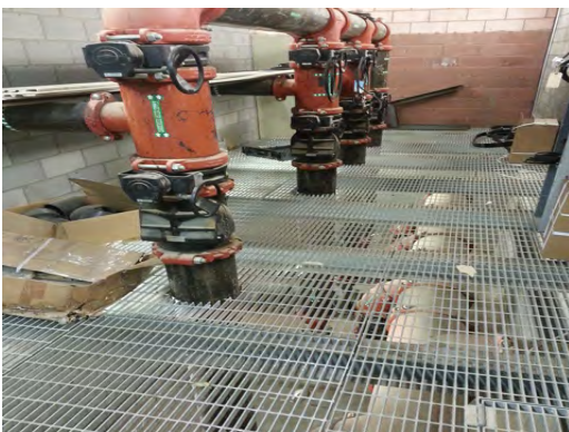
Chapin HS - Cooling Tower Distribution Piping
