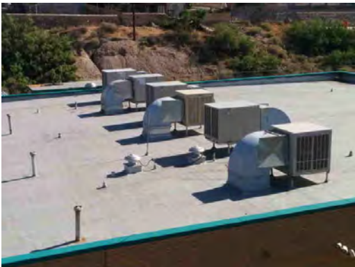
Center for Career & Tech - Rooftop Equipment
