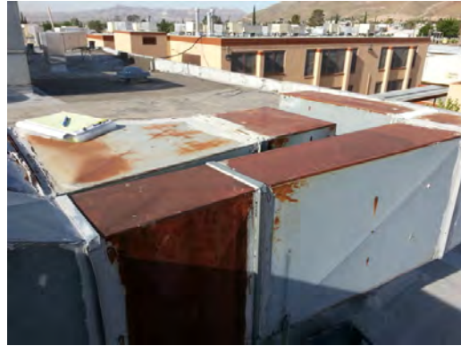
Rusk ES - Rusted Duct
