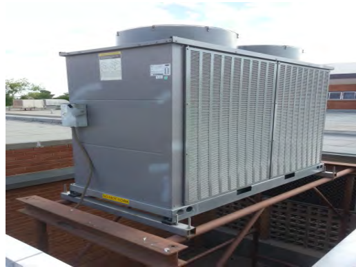
Burgess - Main Building Cooling Tower
