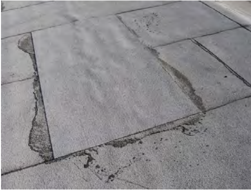
Schuster ES - Roof Patch
