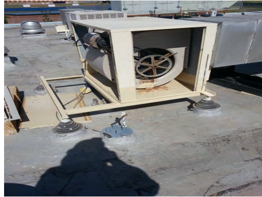
Crosby ES - Damaged Evap 02
