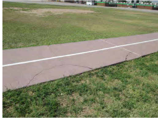
Roberts ES - Damaged Paving at Track
