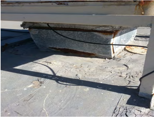
Burleson ES - Corroded Duct
