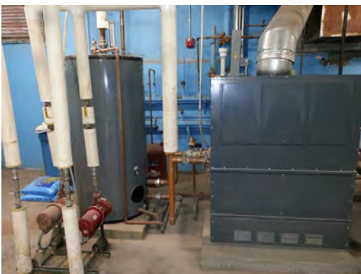
Alta Vista ES - Water Storage and Boiler
