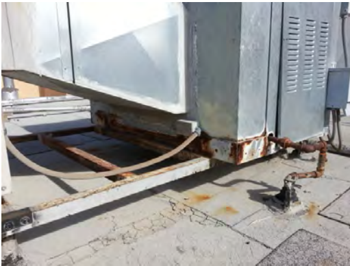
Rusk ES - Rusted Furnace Cabinet
