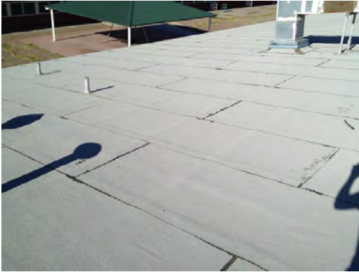
Burleson ES - Roof General Condition 04
