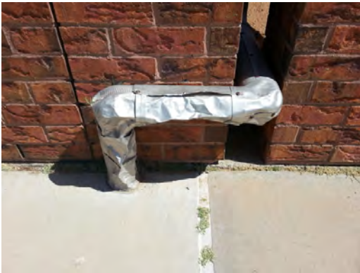
Bradley ES - Damaged Jacketing
