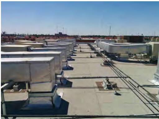
Douglass ES - Rooftop Equipment
