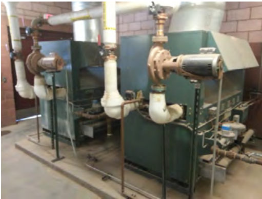
Chapin HS - Hot Water Boiler
