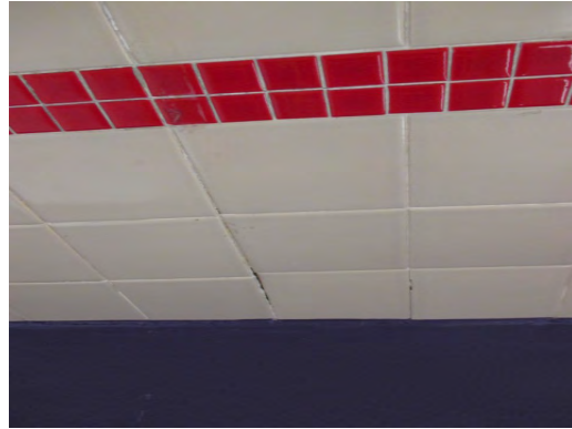
Cooley ES - Damaged Ceramic Tile Wall
