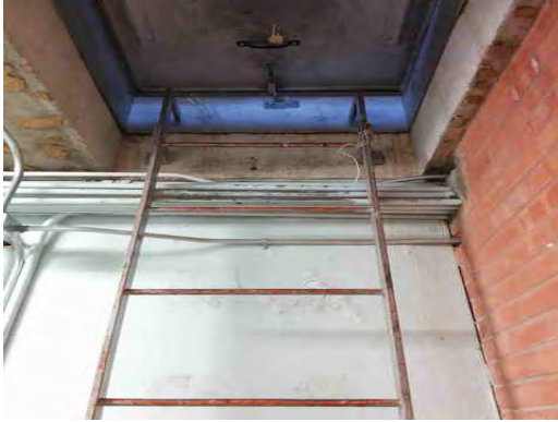
Lamar ES - Aged Ladder to Roof Hatch
