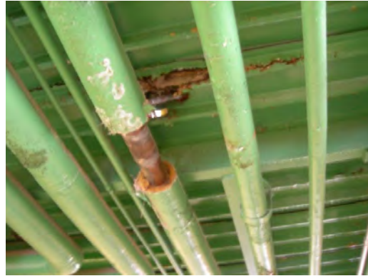
Putnam ES - Corrosion on Covered Walkway
