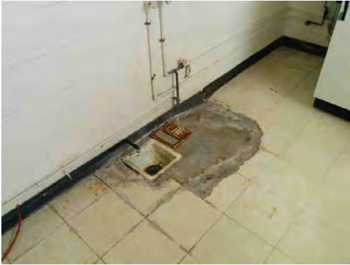
Guillen MS - Damaged Flooring at Floor Drain
