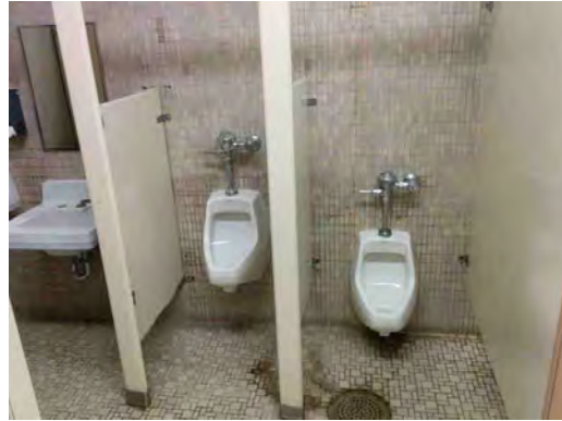
Bonham ES - Restroom Fixtures
