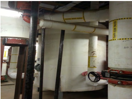
Chapin HS - Hot Water Storage
