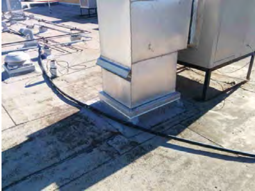
Bliss ES - Worn Roofing Material
