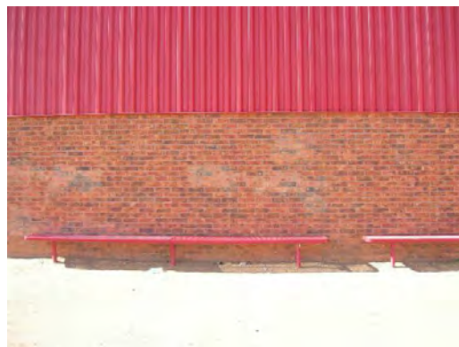
Bradley ES - Exterior Requires Cleaning
