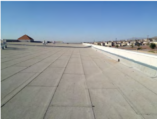
Powell ES - Roof General Condition
