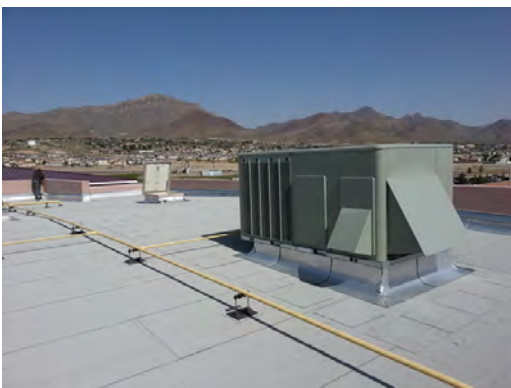
Chapin HS - Rooftop Packaged AC Unit
