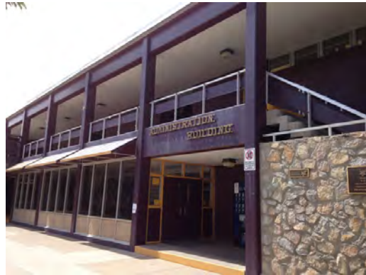
Address HS - Building 4 Entry
