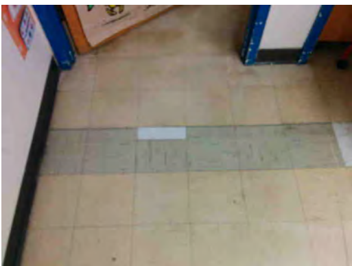
Hawkins ES - Damaged VCT Flooring
