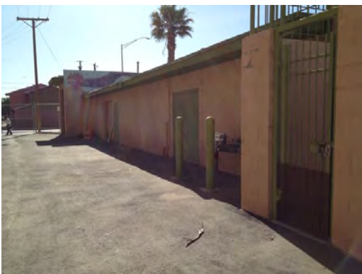
Aoy ES - Maintenance Building
