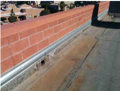
Tippin ES - Evidence of Ponding at Drain
