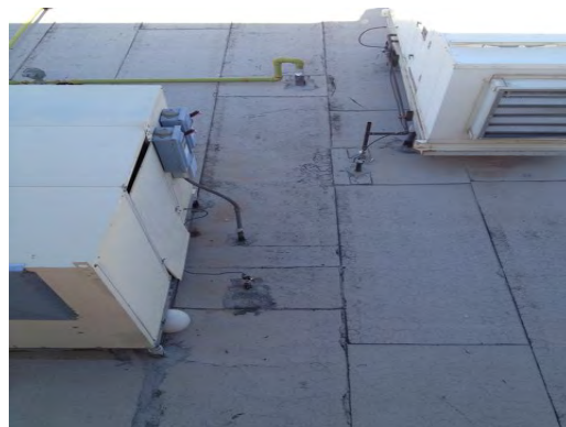
Aoy ES - Kitchen Roof Condition 02
