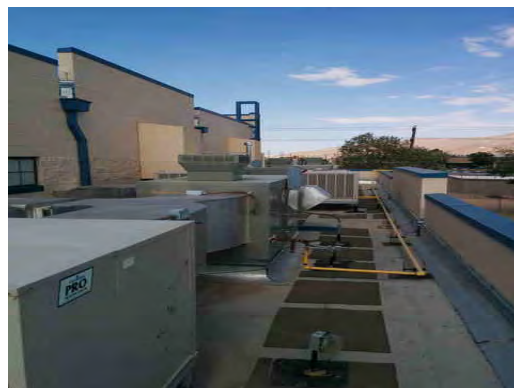
Hughey ES - Rooftop Equipment
