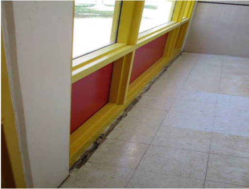
Cooley ES - Damaged VCT Flooring at Wall
