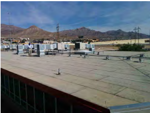
Bliss ES - Typical Rooftop Equipment
