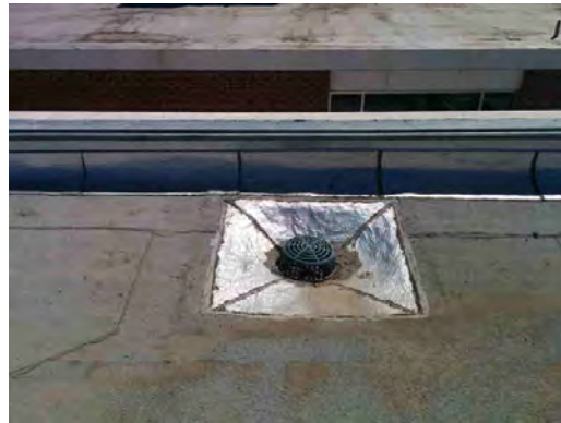
Douglass ES - Roof Drain
