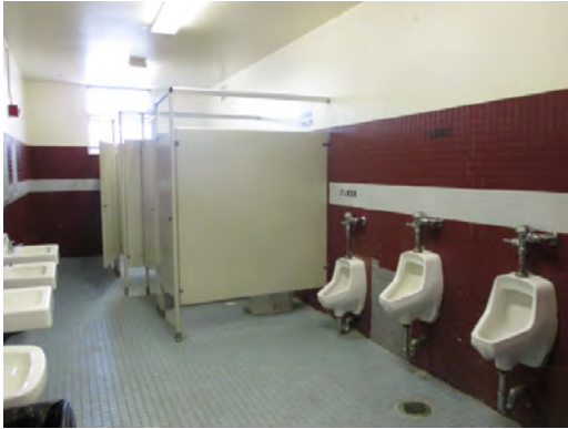
Clardy ES - Restroom Fixtures and Finishes
