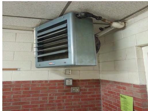
Burleson ES - Hallway Unit Heater
