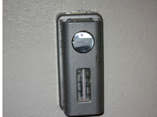
Schuster ES - Abandoned Pneumatic Control
