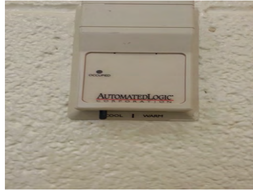
Collins ES - Dated Heating Thermostat
