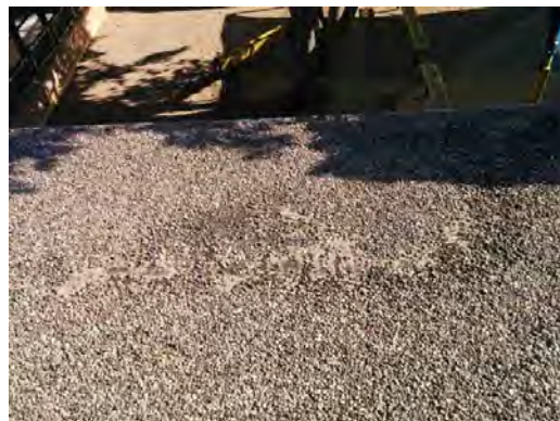
Hughey ES - Evidence of Ponding on Roof
