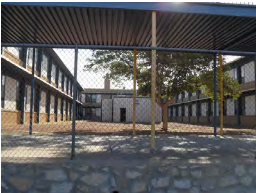
Armendariz MS - Chiller Building Exterior
