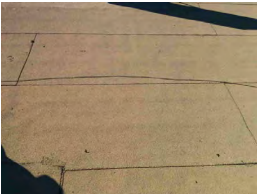
Guerrero ES - Roof General Condition
