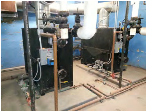
Alta Vista ES - Heating Boilers
