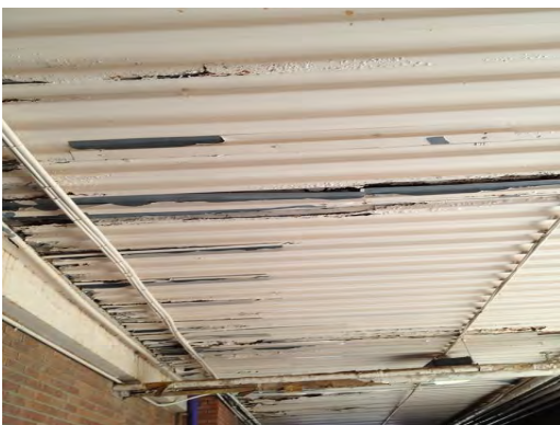
Burgess - Damaged Canopy 02
