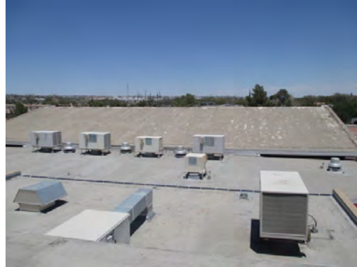
Henderson MS - Rooftop Equipment
