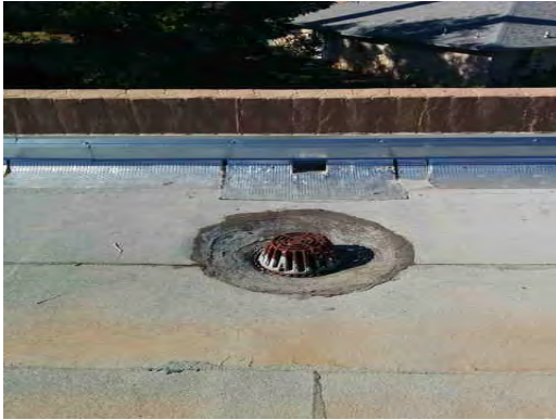
Rivera ES - Roof Drain
