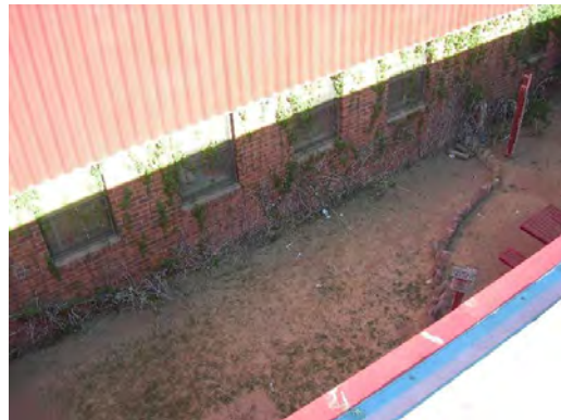
Bradley ES - Courtyard
