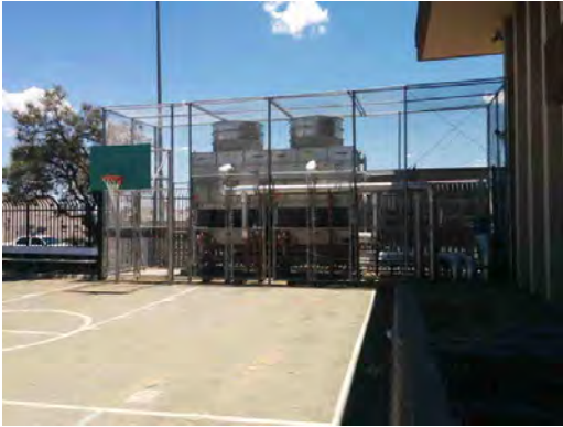
Telles Academy HS - Mechanical Yard
