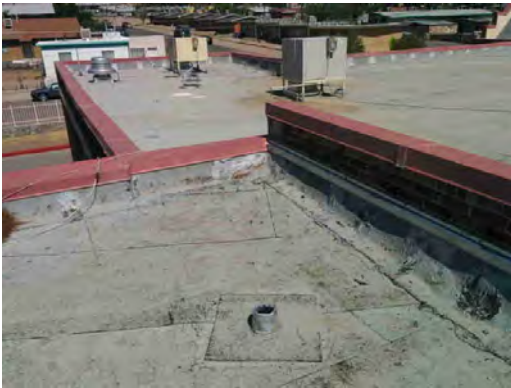
Travis ES - Weathered Roofing Material 02
