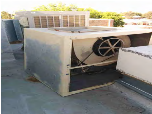
Barron ES - Rooftop Equipment
