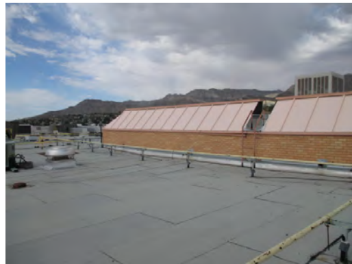
Canyon Hills MS - Roof General Condition 02
