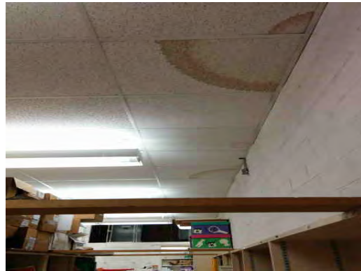
Hawkins ES - Stained Ceiling Tiles 02
