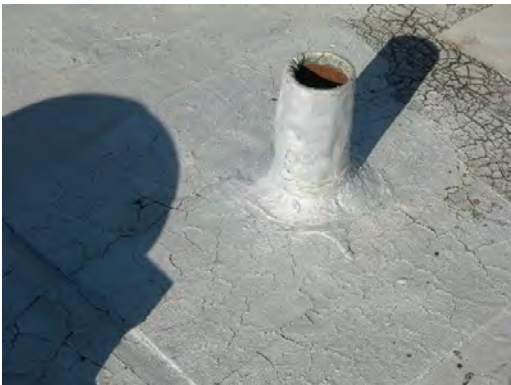
Putnam ES - Roof Flashing 01
