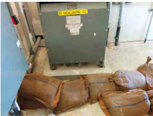
Herrera ES - Sandbags at Electrical Equipment 02
