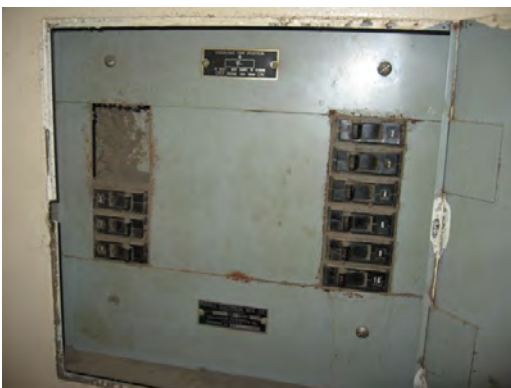
Dowell ES - Aged and Obsolete Panelboard
