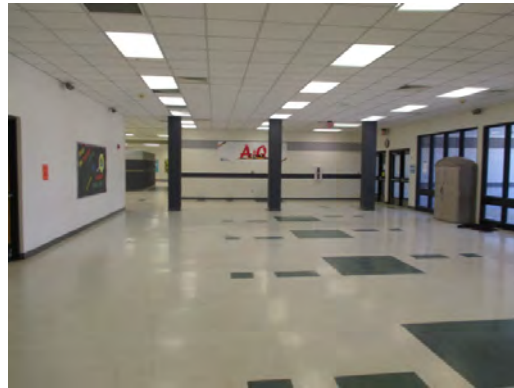
Kohlberg ES - Interior Finishes
