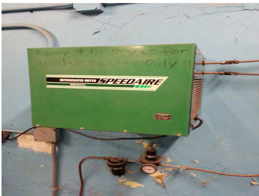
Alta Vista ES - Dated Pneumatic Air Dryer
