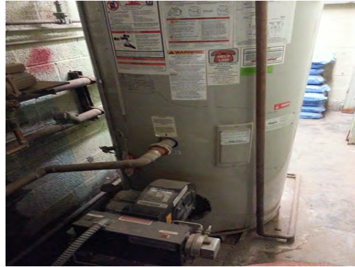
Burleson ES - Hot Water Boiler
