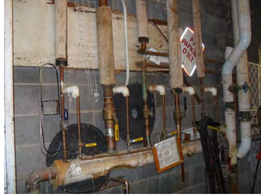
Newman ES - Aged Pipe Insulation
