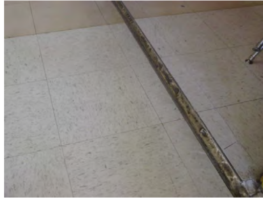
Cooley ES - Damaged VCT Flooring
