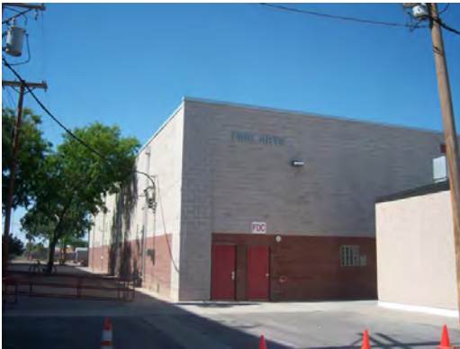
Jefferson HS - Fine Arts Building Exterior
