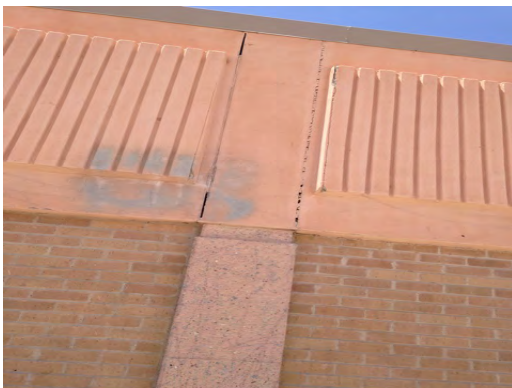
Lincoln MS - Exterior Wall Requires Paint
