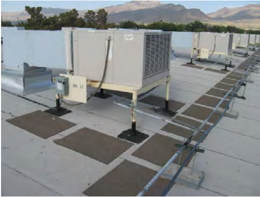
Dowell ES - Newer Evap Cooler for Classrooms
