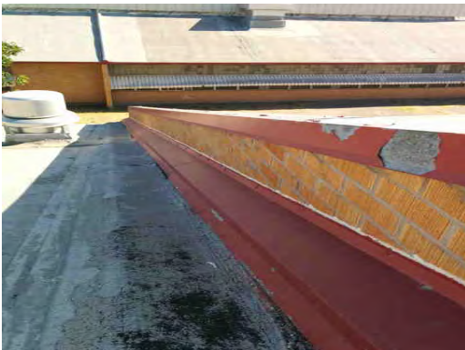
Hillside ES - Weathered Roofing 02
