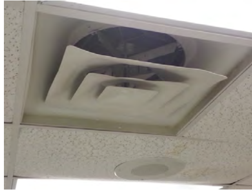
Green ES - Damaged Gym Air Supply Diffuser
