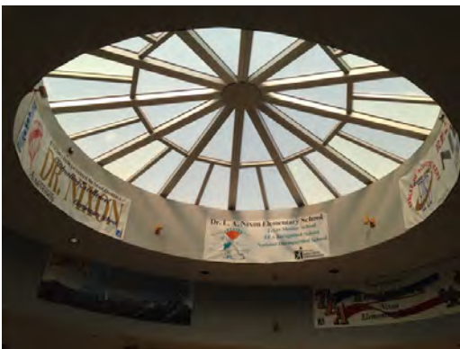
Nixon ES - Main Entry Skylight
