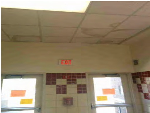
Franklin HS - Stained Ceiling Tiles
