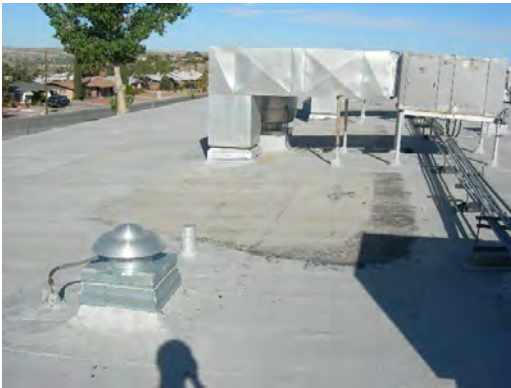
Putnam ES - Roof General Condition 03
