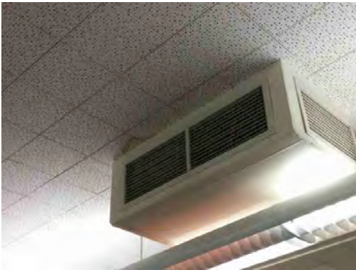
Bonham ES - Evaporative Cooler
