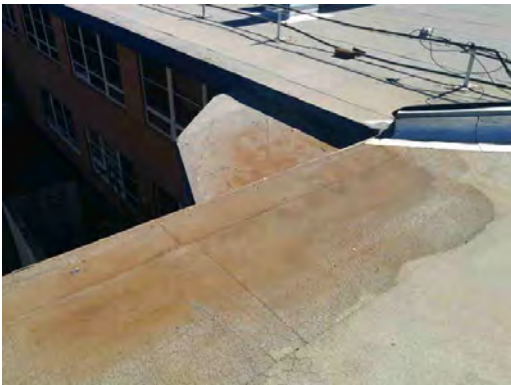
Irvin HS - Evidence of Ponding on Roof
