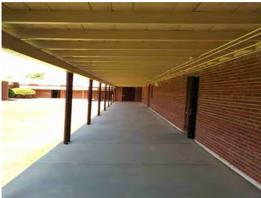
Wainwright ES - Covered Walkway
