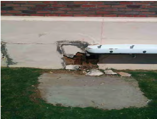
Travis ES - Damaged Exterior Wall at Drinking Fountain
