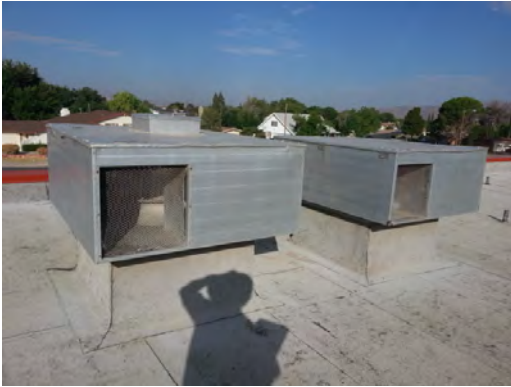
Cielo Vista - Auditorium Exhaust Fans
