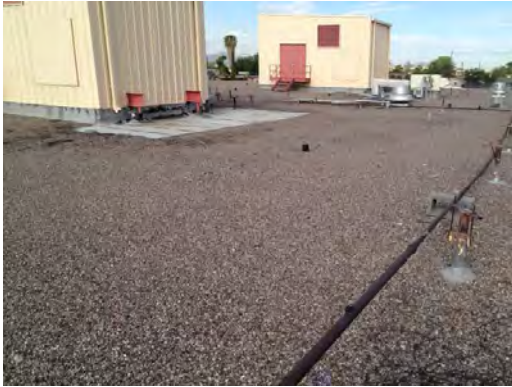
MacArthur ES MS - Roof Condition 01
