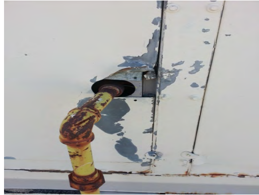
Crosby ES - Modified Gas Burner Pipe Inlet
