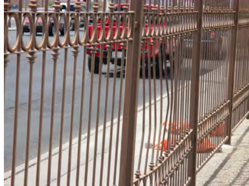
Silva Health Magnet HS - Damaged Ornamental Fence
