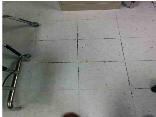
Guerrero ES - Worn VCT Flooring
