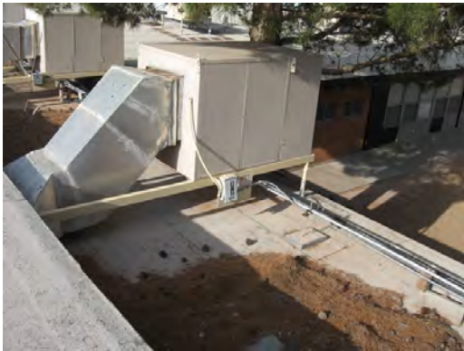
Dowell ES - Evap Coolers For Multipurpose Room
