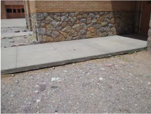
Canyon Hills MS - Erosion at Sidewalk 02
