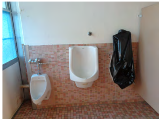
Coronado HS -Restroom Fixtures
