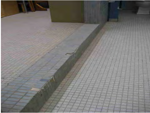
Crosby ES - Damaged Ceramic Tile Floor 01
