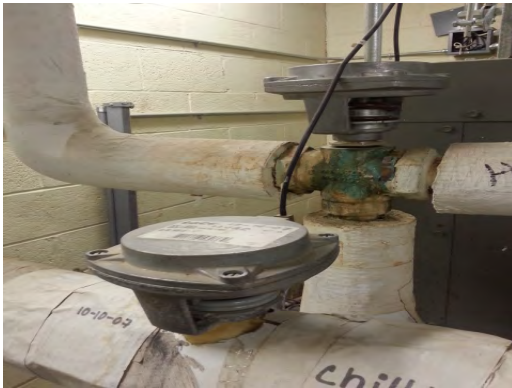
Clendenin ES - Heating and Chilled Water Valves
