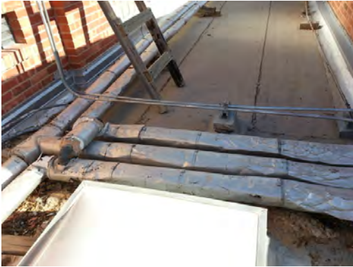
Milam ES - Damaged Insulation and Water Piping Jacketing on Roof
