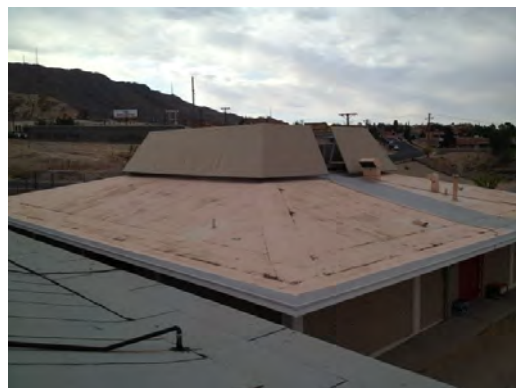
Morehead MS - Roof Condition 02
