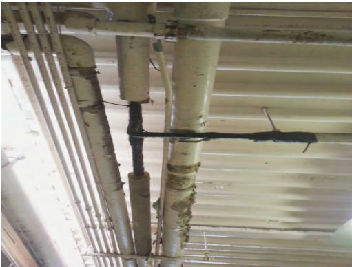
Burgess - Damaged Water Piping
