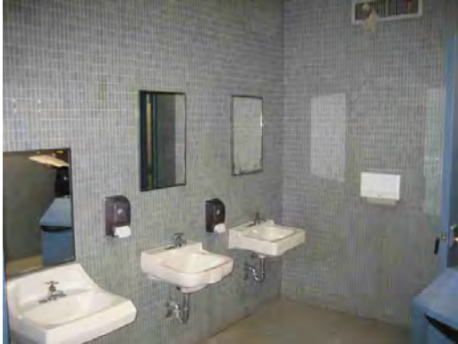
Crosby ES - Restroom Fixtures and Finishes 01
