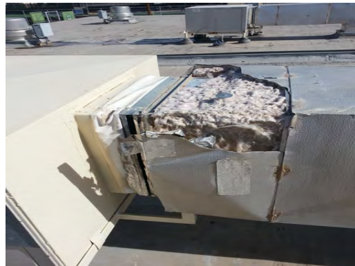
Crosby ES - Torn Duct Insulation on Evap
