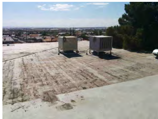
Travis ES - Rooftop Equipment 02
