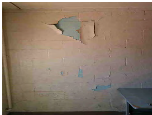
Lamar ES - Paint Peeling on CMU Wall
