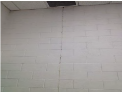
Aoy ES - Crack in Interior Wall 02
