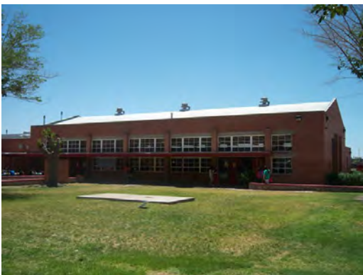
Jefferson HS - Building 3 Elevation
