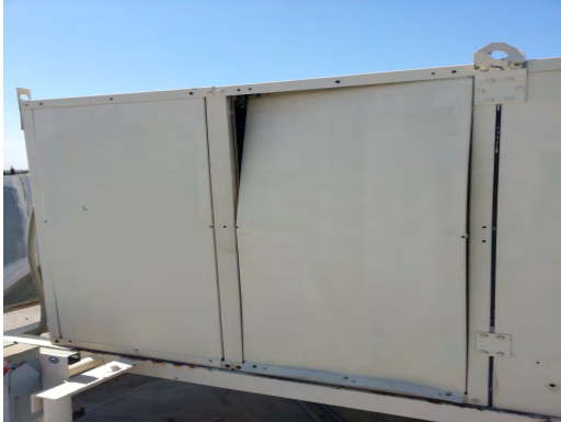
Bradley ES - Bent Evap Panel
