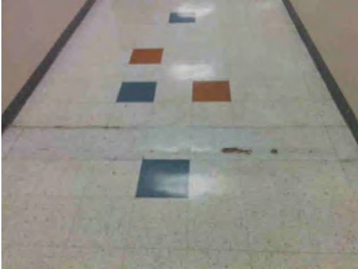
Western Hills ES - Damaged VCT Flooring
