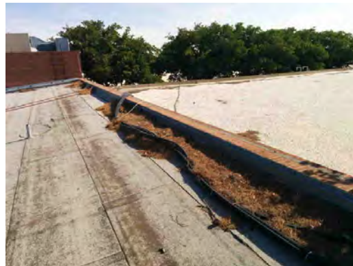
Lee ES - Weathered Roofing Material
