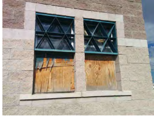
Franklin HS - Damaged Windows Boarded
