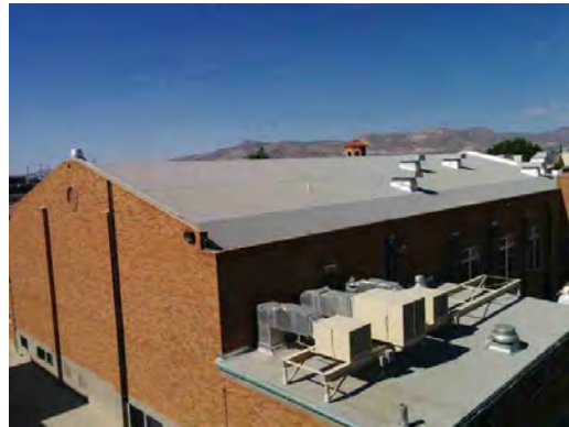
Guillen MS - Rooftop Equipment
