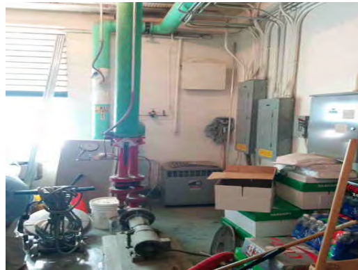
Guillen MS - Electrical Room and Storage
