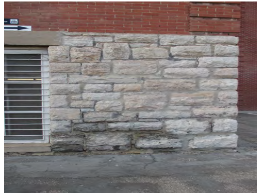
San Jacinto Auit - Exterior Stone Requires Cleaning
