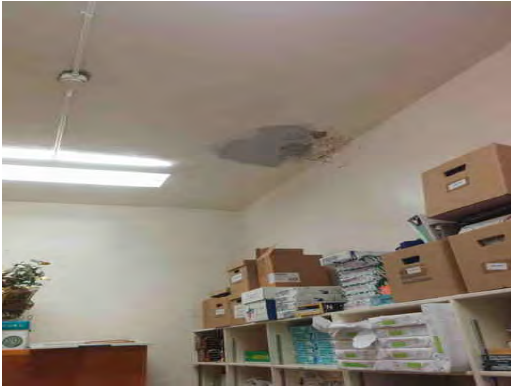
Travis ES - Damaged Ceiling
