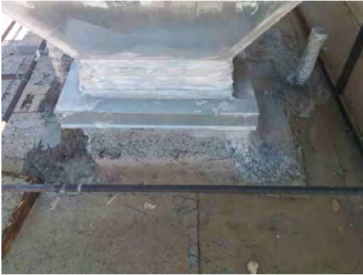
Travis ES - Weathered Equipment Curb
