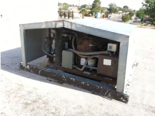
Collins ES - Aged and Weathered Freezer Condensers01
