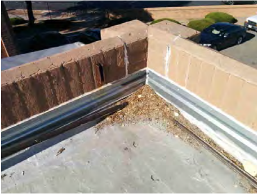
Barron ES - Damaged Roofing
