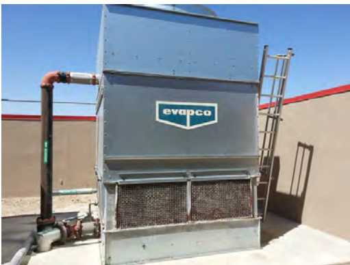
Brown MS - Cooling Tower
