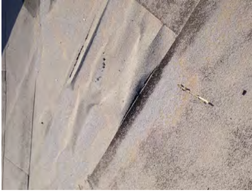
Lincoln MS - Bubbled Roofing Material 02
