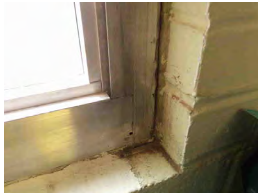
Vilas ES - Damaged, Stained Brick at Window Penetration
