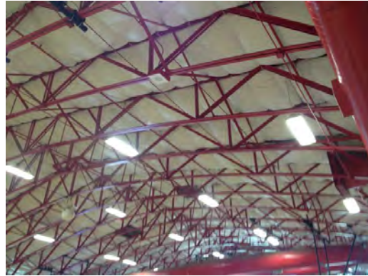
Brown MS - Gyn Exposed Deck Ceiling
