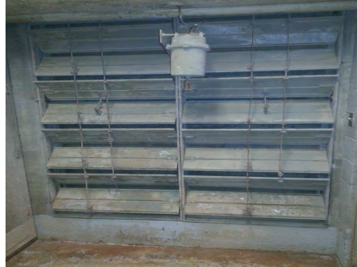
Clendenin ES - Aged Disconnected Return Damper
