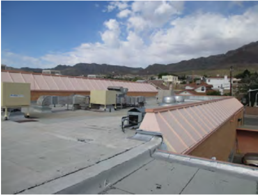
Canyon Hills MS - Rooftop Equipment
