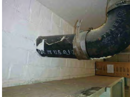
Douglass ES - Cracked Drain
