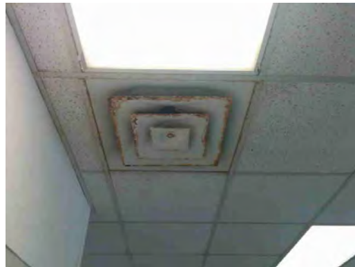
Franklin HS - Rusted Grille
