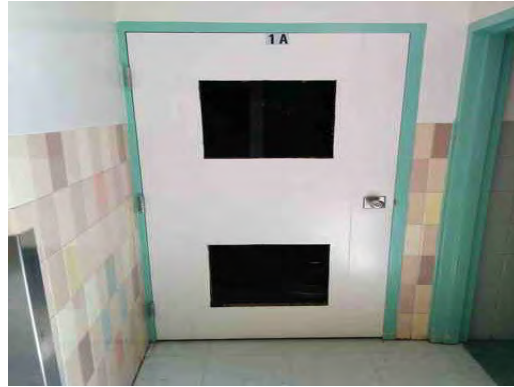
Park ES - Typical Interior Door
