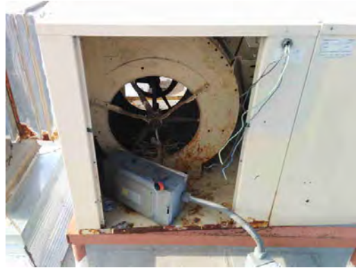
Guillen MS - Damaged Rooftop Equipment
