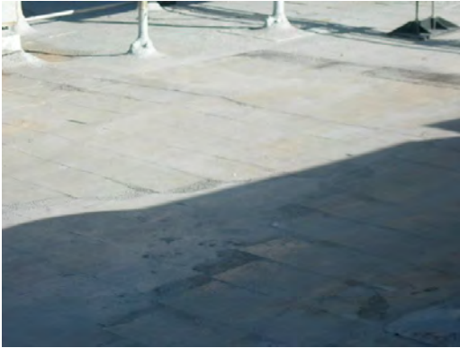
Putnam ES - Roof General Condition 01
