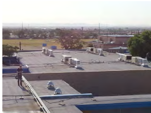
Collins ES - Rooftop Equipment 04
