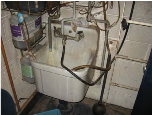
Dowell ES - Service Sink Missing Backflow Preventer
