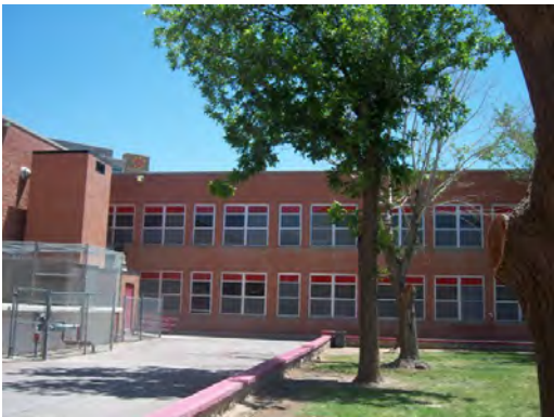
Jefferson HS - Rear Elevation Building 1
