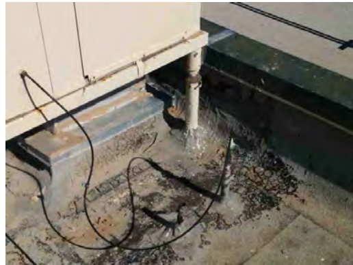
Irvin HS - Damaged Roofing
