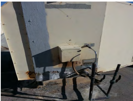
Green ES - Corroded Evap Portion on Furnace Combo
