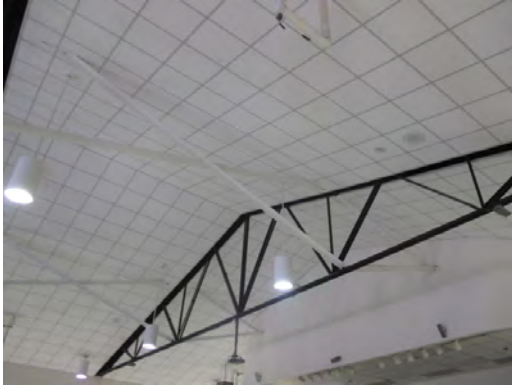
Kohlberg ES - Cafeteria Ceiling
