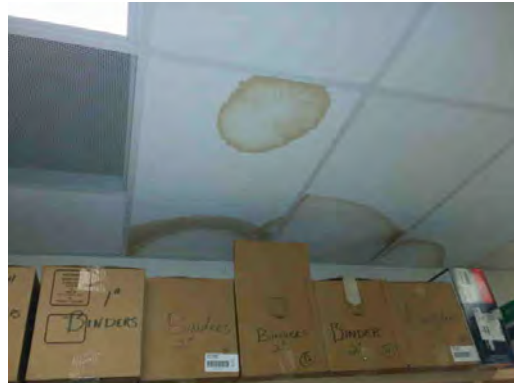
Barron ES - Stained Ceiling Tiles
