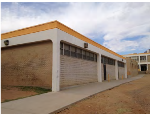
Terrace Hills MS - Exterior Requires Cleaning
