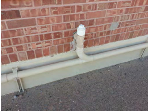
Milam ES - Abandoned PVC Drain Piping
