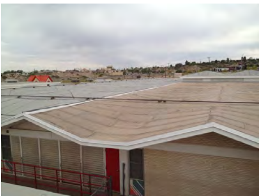
Morehead MS - Roof Condition 01
