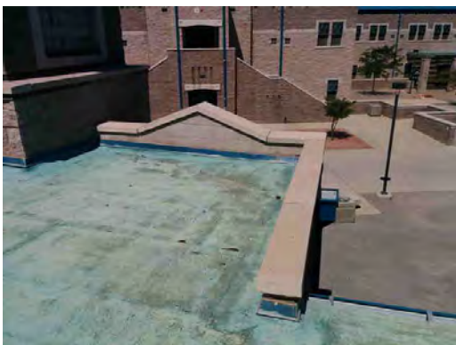
Franklin HS - Weathered Roofing 01
