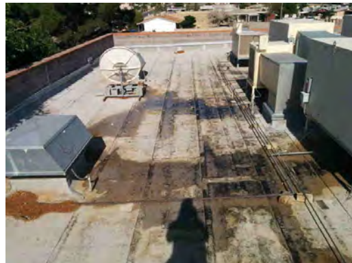
Lee ES - Ponding on Roof
