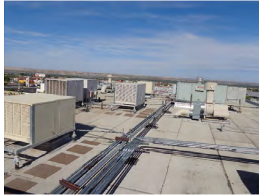
Coronado HS -Rooftop Equipment 01
