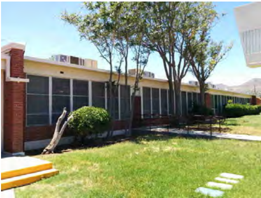
Wainwright ES - Typical Exterior Finishes
