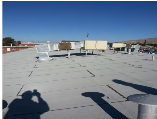
Burleson ES - Typical Classroom Evap Cooler
