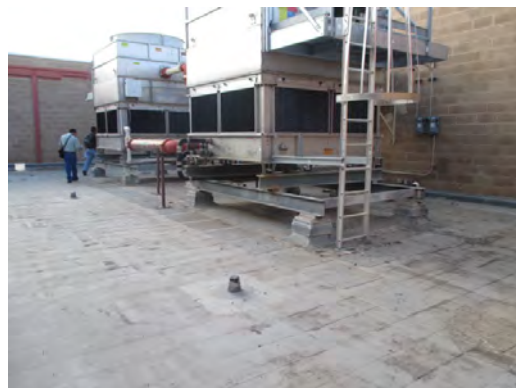
Silva Health Magnet HS - Rooftop Equipment
