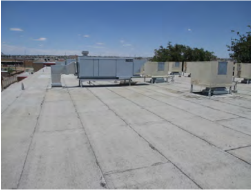
Henderson MS - Roof General Condition
