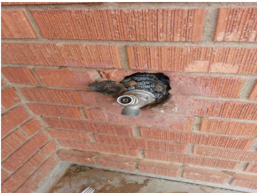
Burgess - Damaged Hose Bibb
