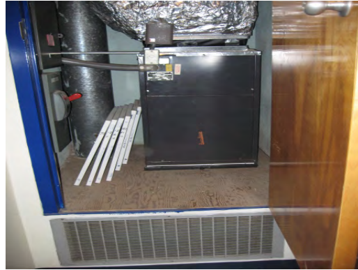
Schuster ES - New Office Electric Furnace
