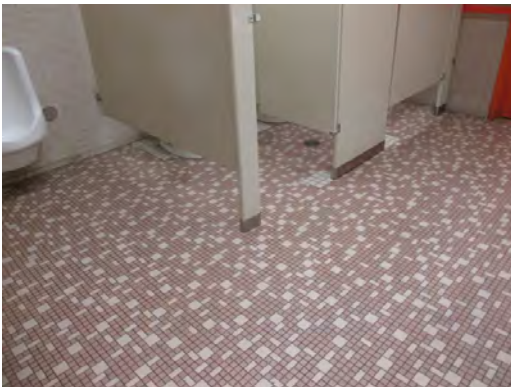
Cooley ES - Restroom Flooring
