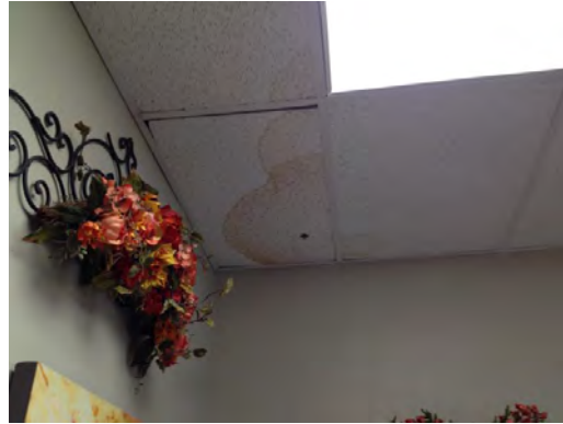
Brown MS - Damaged Ceiling Tiles
