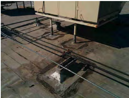
Douglass ES - Evidence of Ponding on Roof
