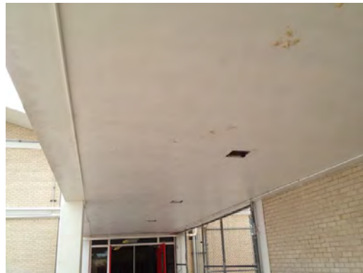
Morehead MS - Covered Walkway
