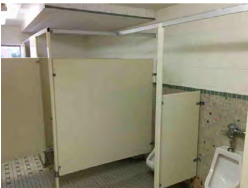
Dowell ES - Restroom Finishes
