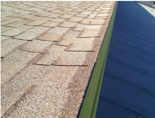
Aoy ES - Roof Condition 03
