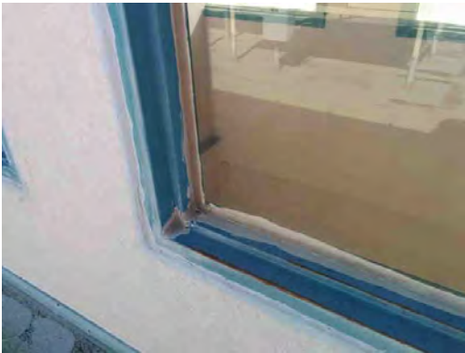
Guillen MS - Damaged Window Frame
