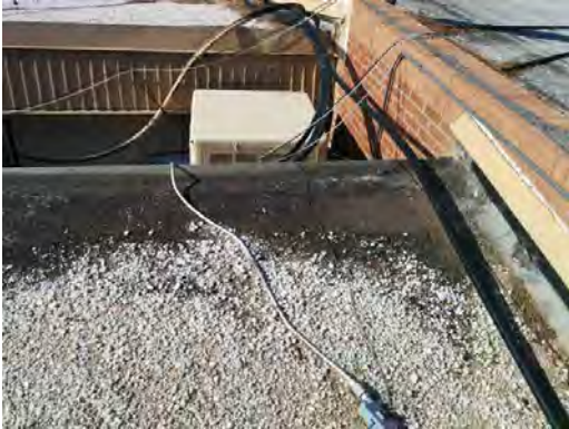
Lee ES - Worn Roofing
