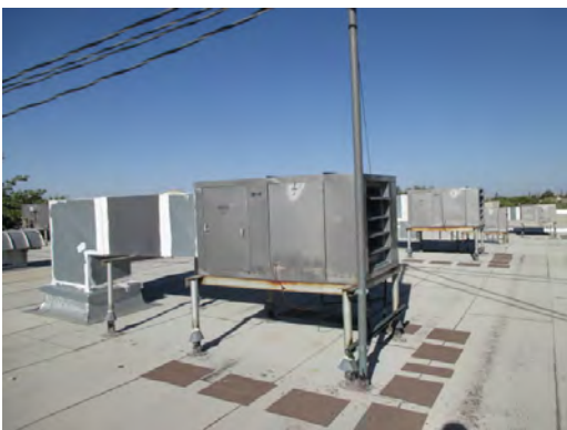
Polk ES - Rooftop Equipment 07
