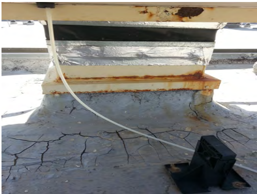
Crosby ES - Rusted Duct Inlet
