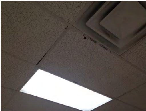
Brown MS - Damaged Grid Ceiling
