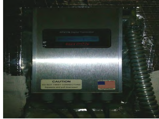
MacArthur ES MS - AHU Digital Sensor Controller
