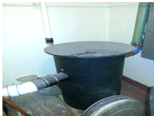
El Paso HS - Sewer Lines in Need of Repair
