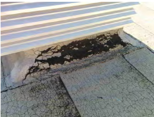
Center for Career & Tech - Damaged Membrane at Equipment
