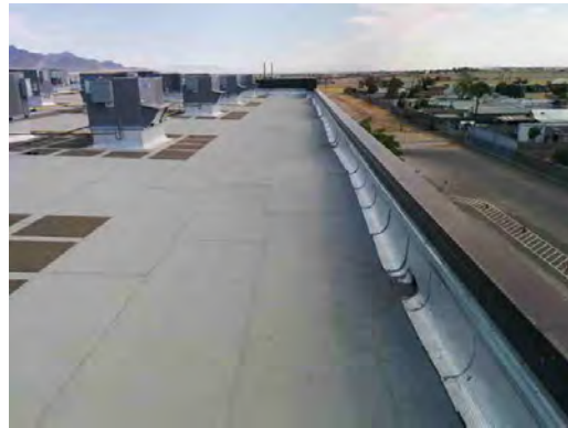
Hughey ES - Roof General Condition
