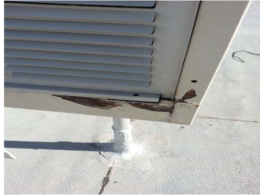
Burleson ES - Rusted Evap Cooler
