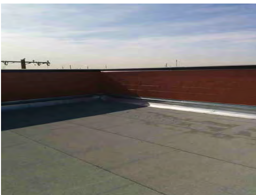
Hawkins ES - Roof General Condition
