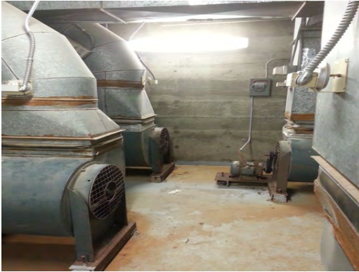
Clendenin ES - Chilled Air Supply Fans
