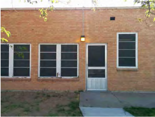
Bonham ES - Damaged Window Frames
