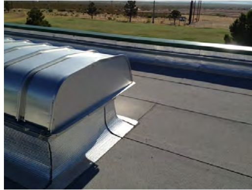
Richardson MS - Roof Exhaust
