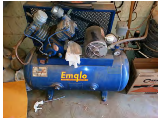
MacArthur ES MS - Air Compressor for Controls
