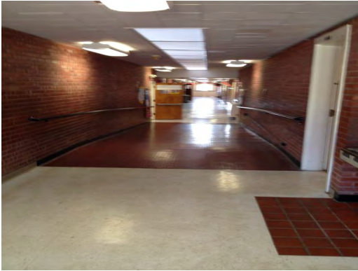
Burnet ES - Hallway Finishes
