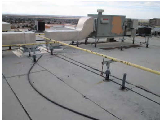
Canyon Hills MS - Rooftop Equipment 04
