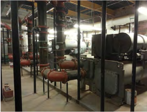
Chapin HS - Chillers
