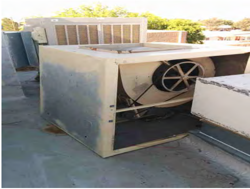
Rivera ES - Rooftop Equipment
