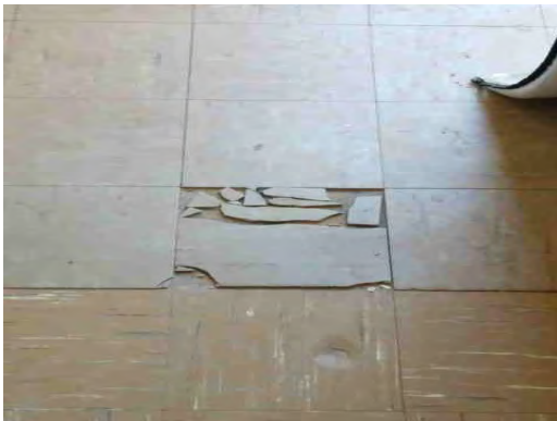
Bliss ES - Broken Tile Floor
