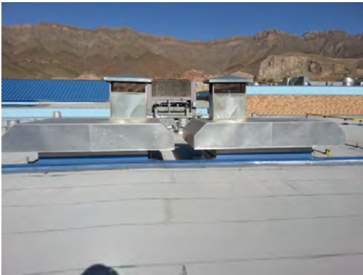
Clendenin ES - Mechanical Room Vents
