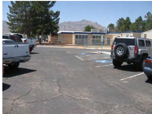
Schuster ES - Damaged Parking Lot Paving
