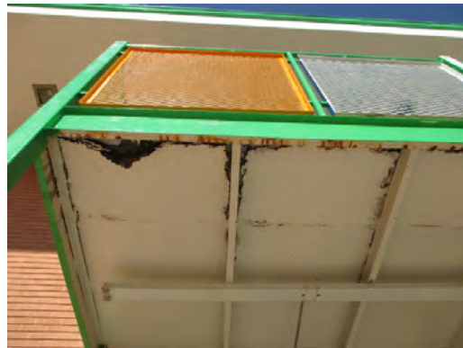
Roberts ES - Corrosion at Stairs 01
