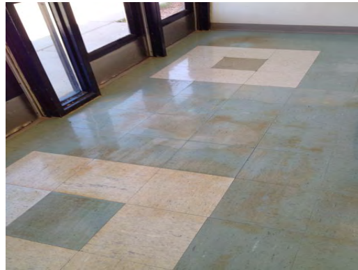
Richardson MS - Water Damaged VCT Flooring
