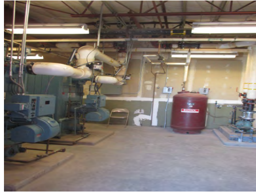
Silva Health Magnet HS - Mechanical Room
