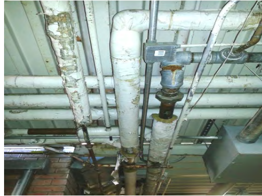
Burgess - Damaged Water Piping Insulation
