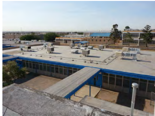
Collins ES - Rooftop Equipment 02
