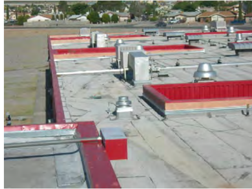
Bradley ES - Roof Condition 03
