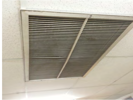
Burgess - Damaged Grilles Entire Building
