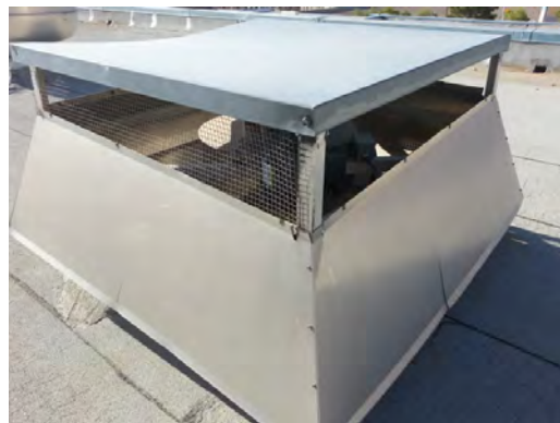
Clendenin ES - Broken Exhaust Fan Housing
