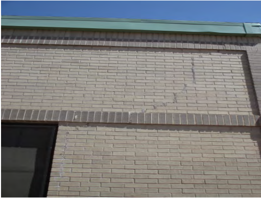
Franklin 9th Grade Center - Cracked Exterior Brick
