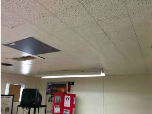
Center for Career & Tech - Adhered Tile Ceiling
