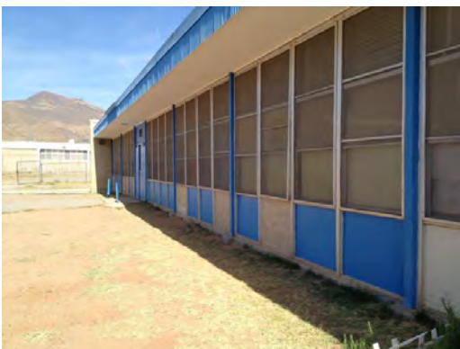
Collins ES - Exterior Finishes
