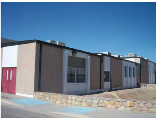
Jefferson HS - Building 8 Elevation
