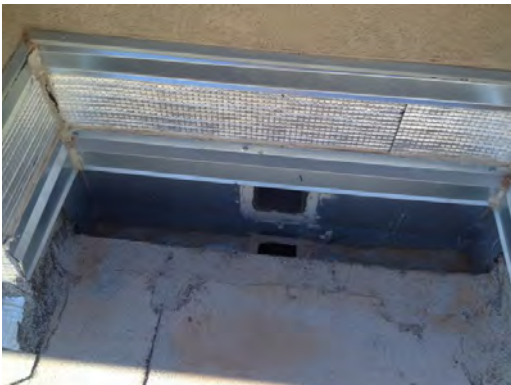
Charles MS - Roof Gutter
