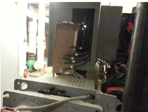
Chapin HS - Chiller Offline for Repair
