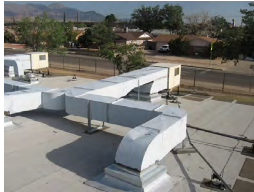
Dowell ES - Rooftop Air Unit and Ductwork
