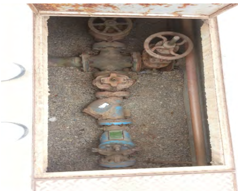
Burgess - Main Entrance Water Supply Valves
