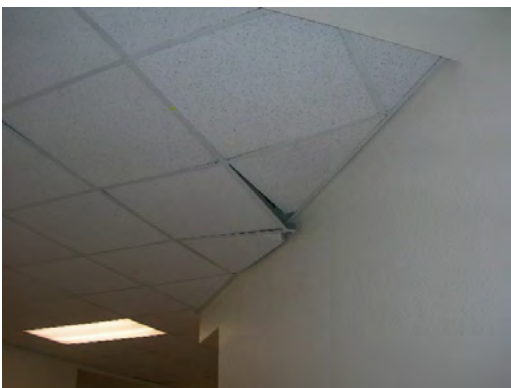
Chapin HS - Damaged Grid Ceiling
