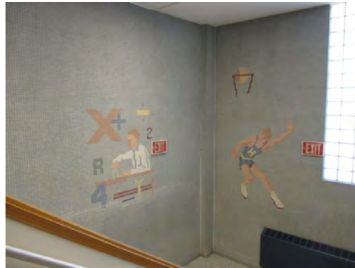
Henderson MS - Interior Ceramic Tile Wall
