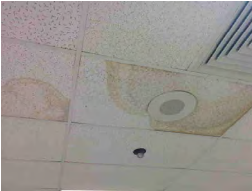
Guerrero ES - Stained Ceiling Tiles
