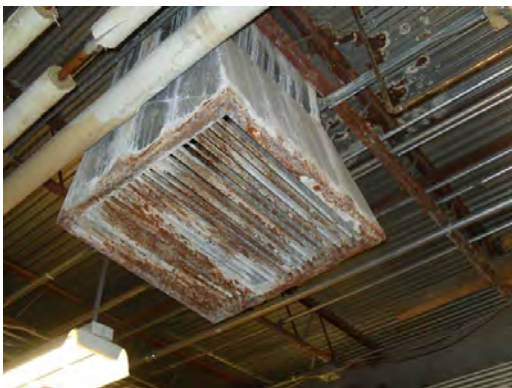
Johnson ES - Corroded Air Register
