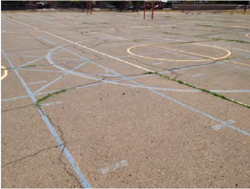
Fannin ES - Cracked Paved Play Area
