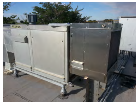
Burgess - Bad Furnace, Evap Combo
