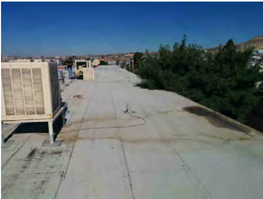
Beall ES - Ponding on Roof 02
