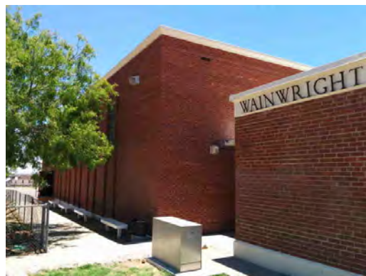
Wainwright ES - Exterior Brick Wall
