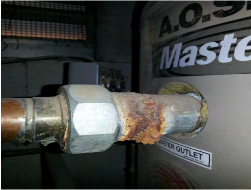
Rusk ES - Corroded Dielectric Union Water Heater
