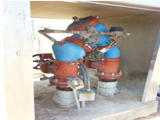
Burgess - Backflow Enclosures Missing Doors
