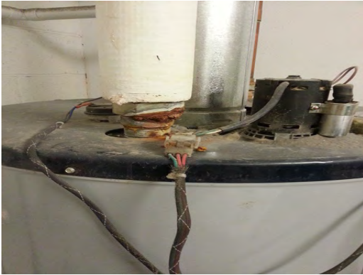
Aoy ES - Corroded Water Heater
