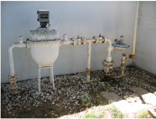
Schuster ES - Rusted Gas Piping
