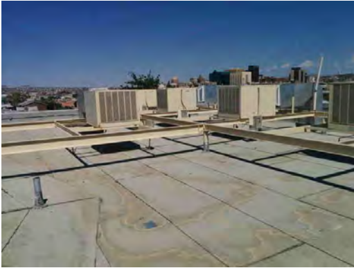
Guillen MS - Evidence of Ponding on Roof
