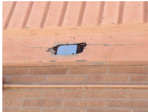
Lincoln MS - Damaged Exterior Wall 01
