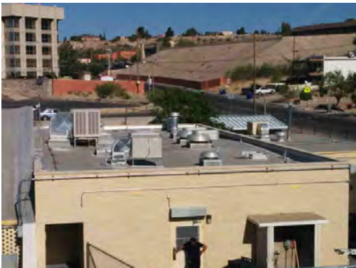
Lamar ES - Rooftop Equipment 02
