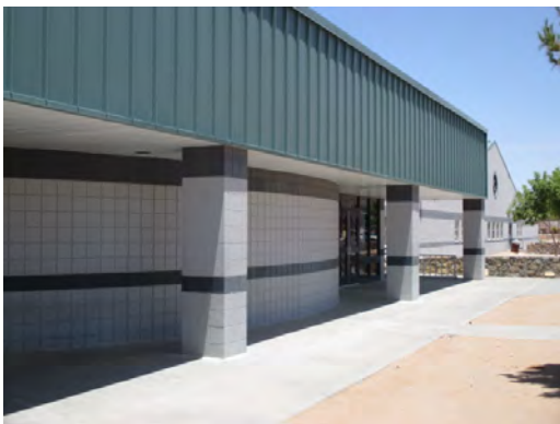
Kohlberg ES - Entry Doors
