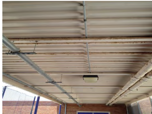
Burgess - Damaged Canopy 01
