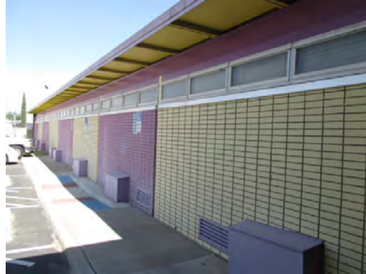
Cooley ES - Original Building Exterior
