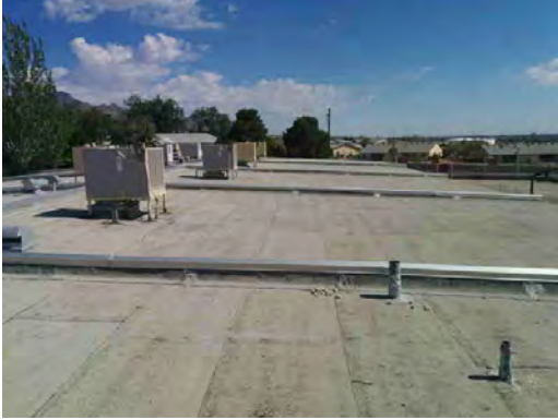
Travis ES - Roof General Condition 02
