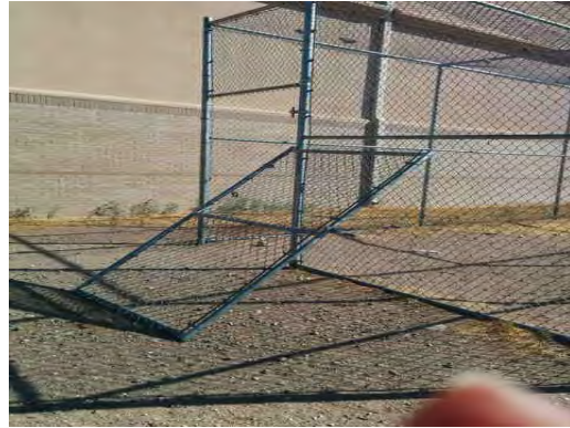
El Paso HS - Damaged Chain Link
