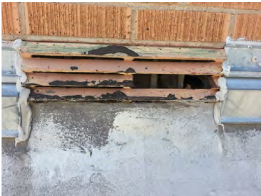
Crosby ES - Damaged Roof Vent
