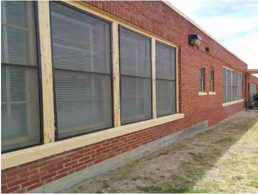
Hawkins ES - Damaged Exterior Windows
