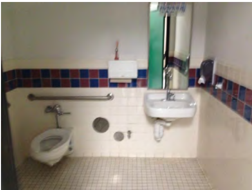
Aoy ES - Restroom Fixtures
