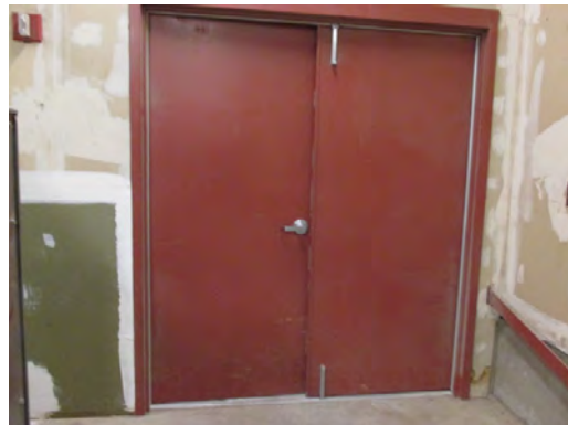
Silva Health Magnet HS - Damaged Exterior Doors Not Closing
