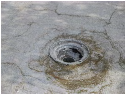
Clardy ES - Roof Drain Missing Cover
