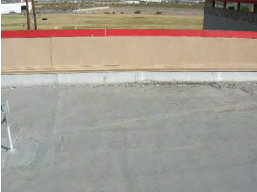
Brown MS - Bubbled Roofing 01
