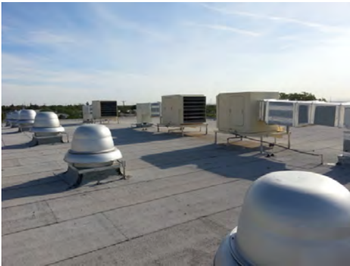
Collins ES - Rooftop Equipment 01
