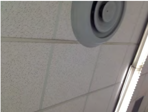
Morehead MS - Typical Ceiling Grid
