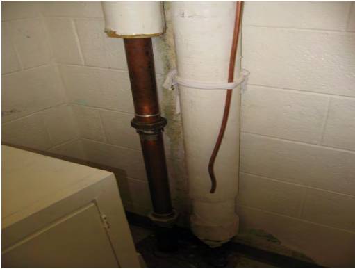
Schuster ES - Unfinished Piping Repair
