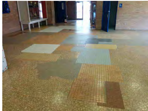
Irvin HS - Damaged Tile Flooring
