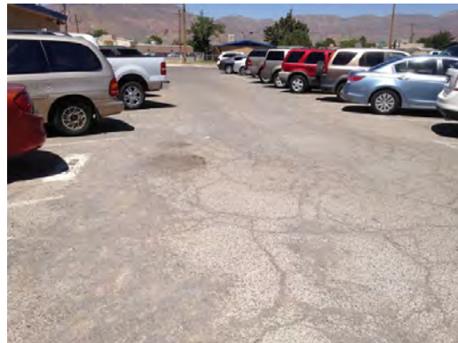
Newman ES - Cracked Parking Lot Paving
