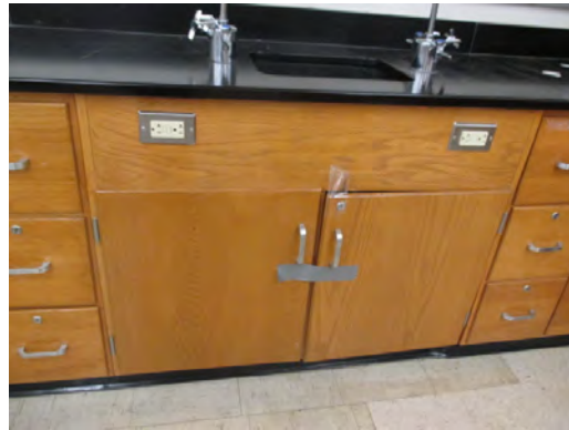
Canyon Hills MS - Damaged Cabinetry
