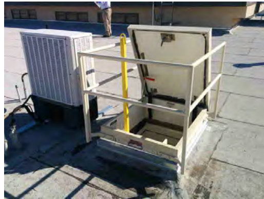
Hornedo MS - Roof Hatch
