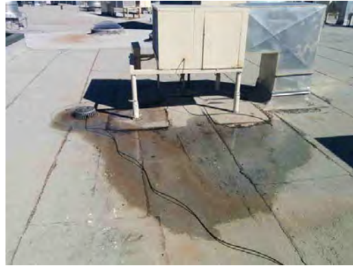
Irvin HS - Ponding on Roof
