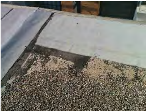
Hughey ES - Weathered Roofing
