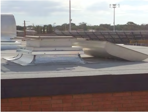
Burgess - Damaged Ventilator
