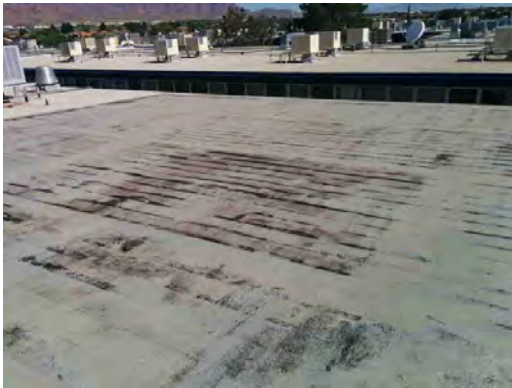
Irvin HS - Weathered Roof
