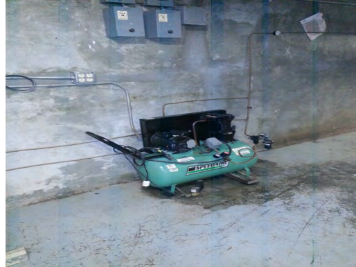
Crosby ES - Pneumatic Air Compressor
