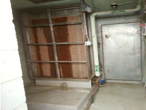
Cielo Vista - Large Room Evap
