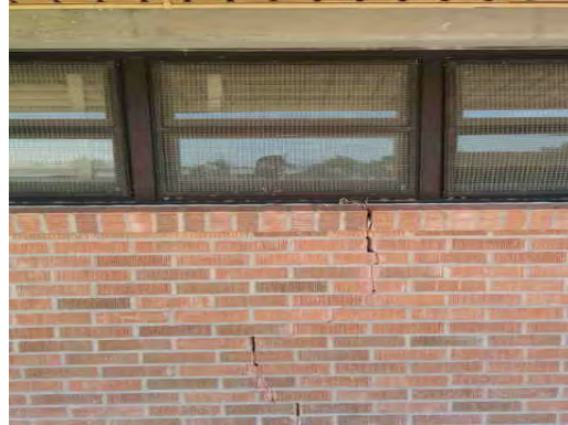
Lee ES - Cracked Exterior Brick Wall
