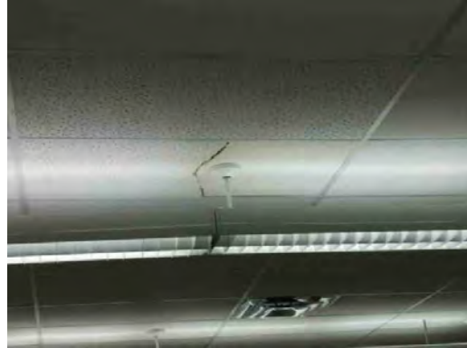
Vilas ES - Damaged Ceiling Tiles
