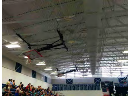
Hornedo MS - Exposed Ceiling in Gym
