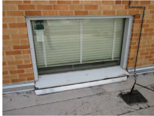
Clardy ES - Roof Window
