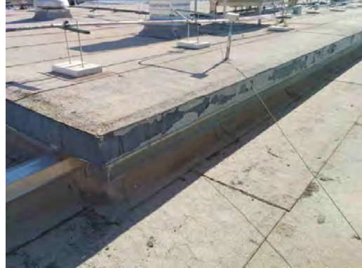
Hughey ES - Weathered Roof
