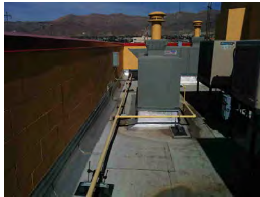
Bliss ES - Rooftop Equipment
