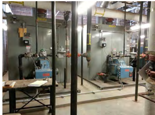
Chapin HS - Heating Boilers
