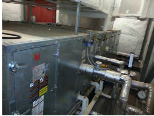
MacArthur ES MS - Typical Rooftop AHU in Penthouses
