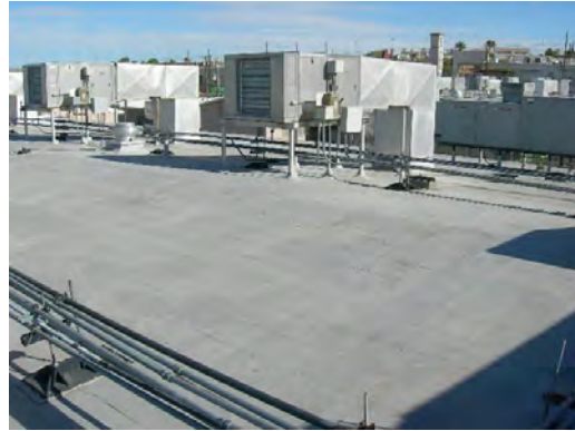
Putnam ES - Roof General Condition 02
