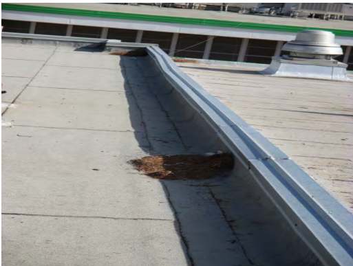
Roberts ES - Clogged Roof Drain
