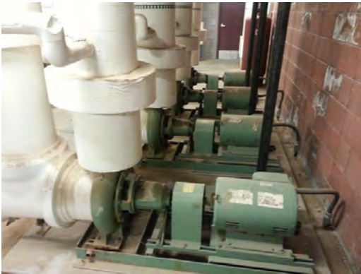
Chapin HS - Chilled Water Return Pumps
