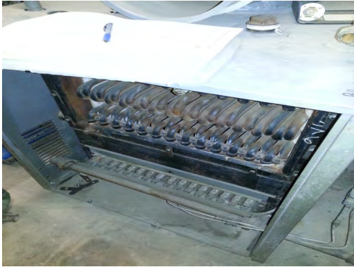
Rusk ES - Hot Water Boiler Under Repair
