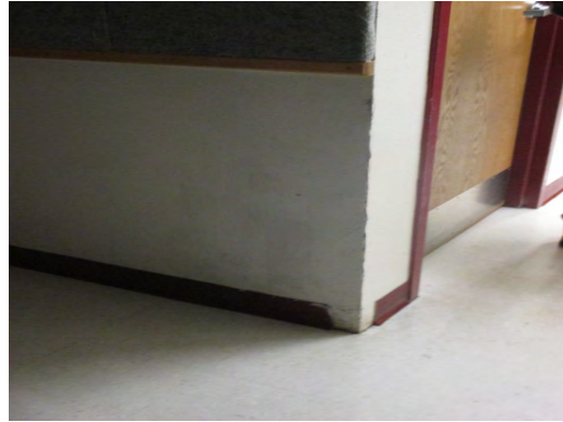
Franklin 9th Grade Center - Damaged Cove Base
