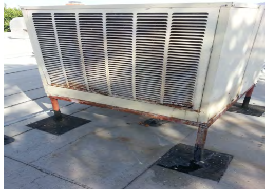
Burgess - Rusted Out Evap Cooler
