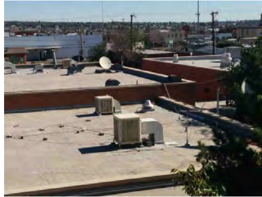
Beall ES - Rooftop Units
