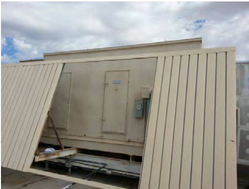
MacArthur ES MS - Large Corroded Evap
