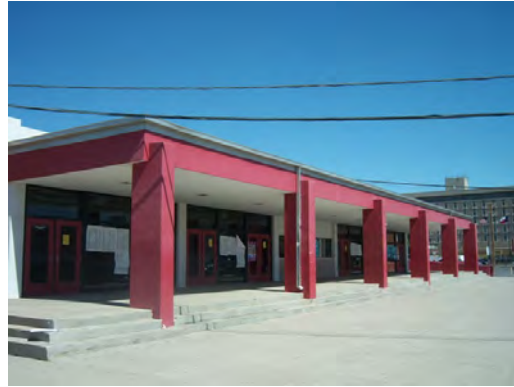
Jefferson HS - Building 6 Elevation
