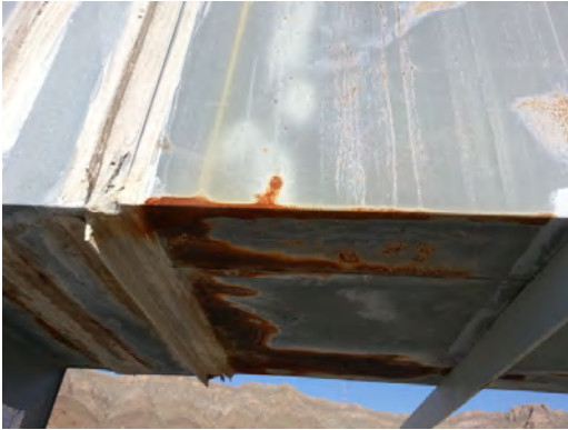
Clendenin ES - Rusted Evap Duct
