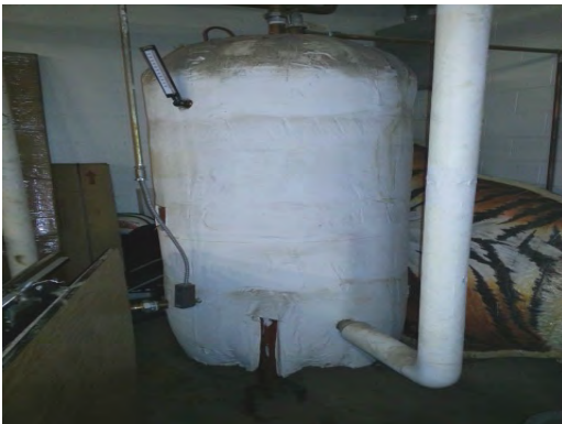
El Paso HS - Hot Water Storage Tank
