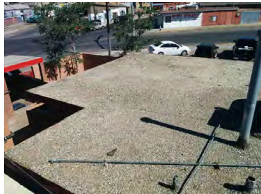
Beall ES - Roof General Condition
