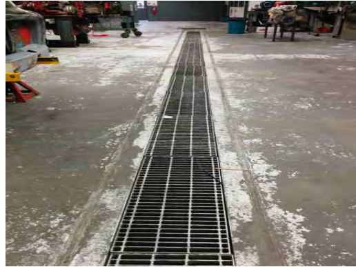
Center for Career & Tech - Worn Concrete Floor
