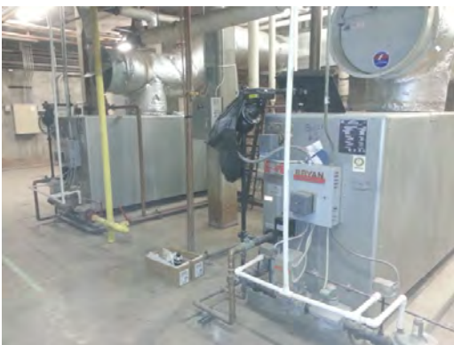
Burgess - Twin Heating Boilers
