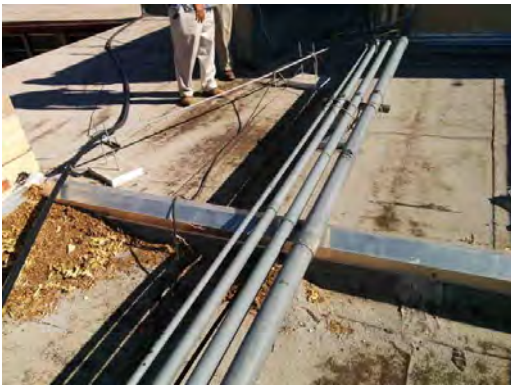
Bliss ES - Evidence of Ponding on Roof
