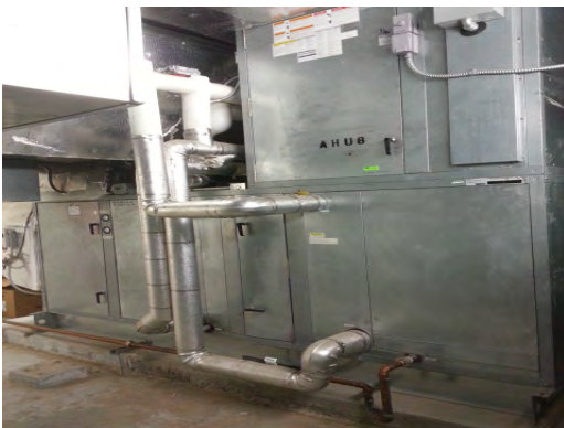
Cielo Vista - Air Handling Unit
