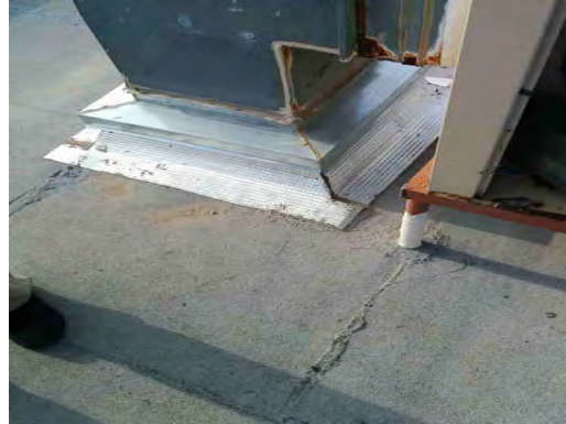
Guillen MS - Corroded Rooftop Equipment
