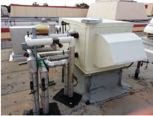
MacArthur ES MS - Small AHU with Hot and chilled Water Coils
