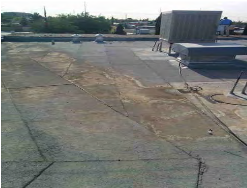
Hawkins ES - Evidence of Ponding on Roof
