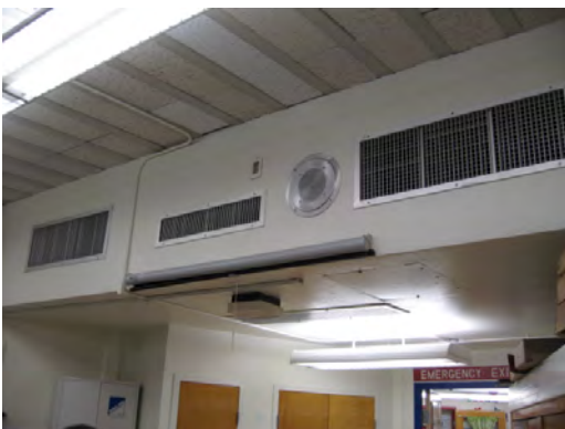
Schuster ES - Typical Heating Cooling Grille Room Setup
