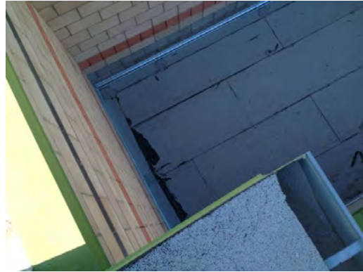
Aoy ES - Roof General Condition 01
