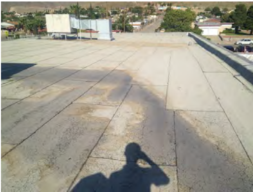
Burnet ES - Roof General Condition
