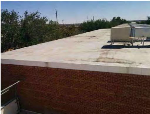
Douglass ES - Worn Roofing Materials 01
