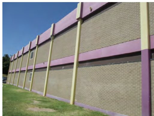
Cooley ES - Exterior Painted Concrete
