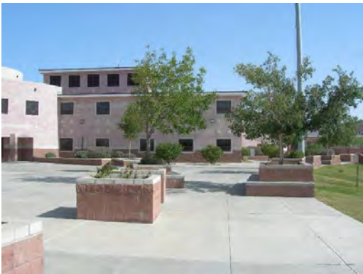
Chapin HS - Rear Elevation 01
