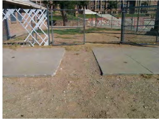
El Paso HS - Damaged Pedestrian Walkway
