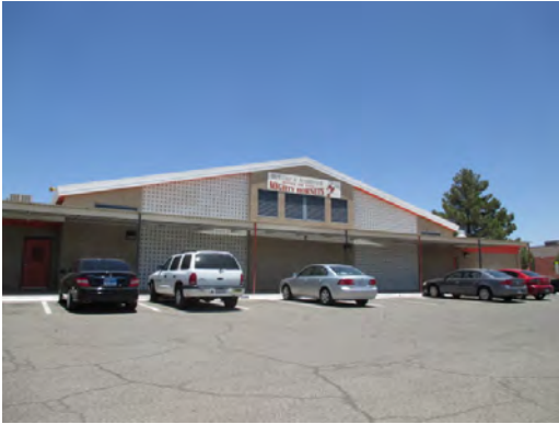
Henderson MS - Gym Exterior
