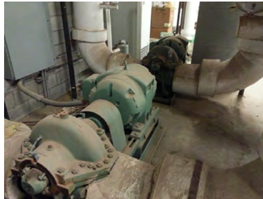
Chapin HS - Chilled Water Supply Pumps
