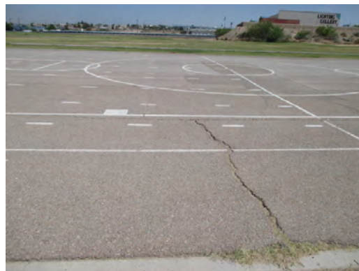
Roberts ES - Cracked in Paved Play Area
