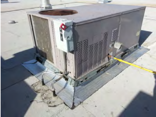
Clendenin ES - Aged and Damaged Package Unit
