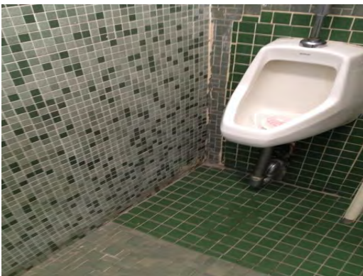
Rusk ES- Mismatched Restroom tile
