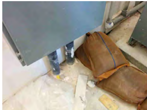
Herrera ES - Sandbags at Electrical Equipment 01
