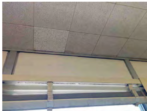
Lamar ES - Damaged Ceiling Tiles
