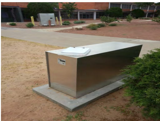
Burgess - Backflow for Irrigation
