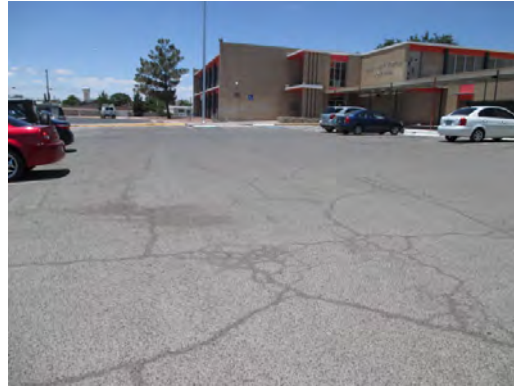
Henderson MS - Cracked Asphalt Paving
