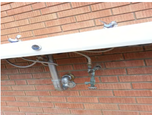
Burgess - Dated Water Supply Piping
