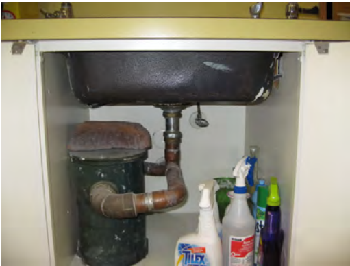
Schuster ES - Inappropriate P-Trap Classroom Sink
