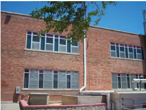
Jefferson HS - Building 1 Exterior Brick
