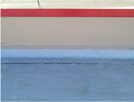
Brown MS - Crack at Roof
