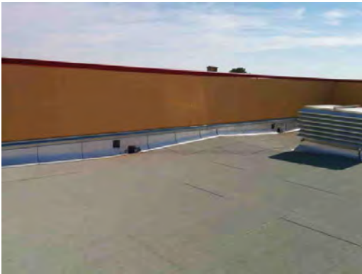
Bliss ES - Roof General Condition 02
