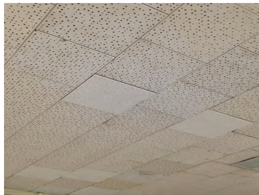
Stanton ES - Mismatched Ceiling Tiles
