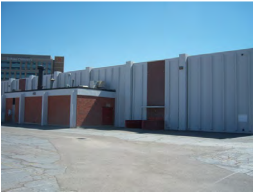
Jefferson HS - Building 6 Rear Elevation
