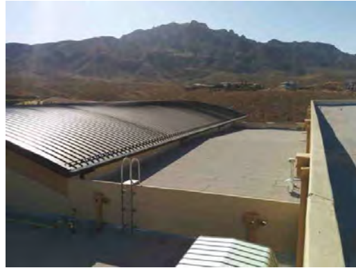
Hornedo MS - Roof Condition
