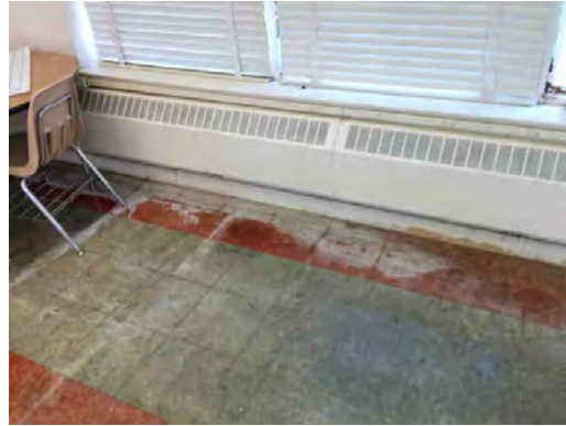
Wainwright ES - Worn VCT Flooring
