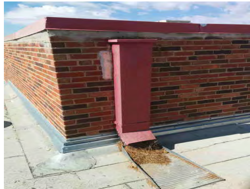
Travis ES - Clogged Downspout
