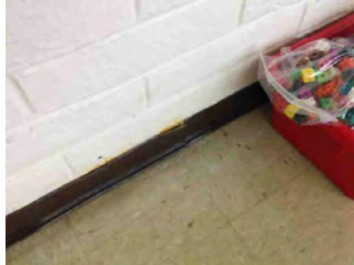
Rivera ES - Damaged Cove Base
