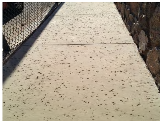
Clendenin ES - Pedestrian Paving
