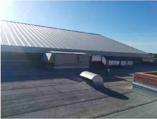
Tippin ES - Roof General Condition
