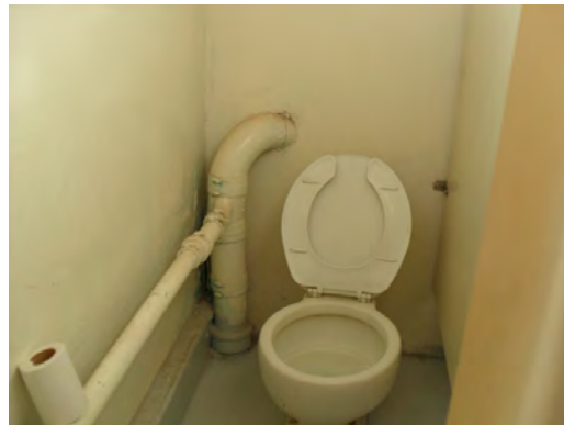
San Jacinto Auit - Resstroom Fixtures
