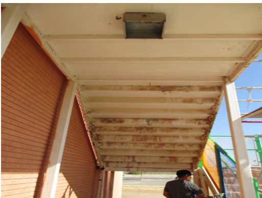
Roberts ES - Corrosion at Stairs 02
