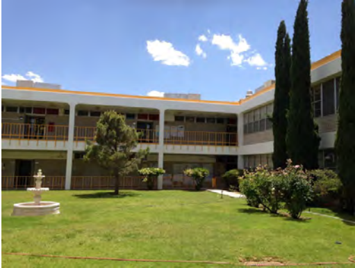
Terrace Hills MS - Building 1 Courtyard
