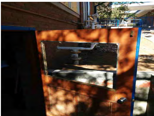
Park ES - Damaged Exterior Door
