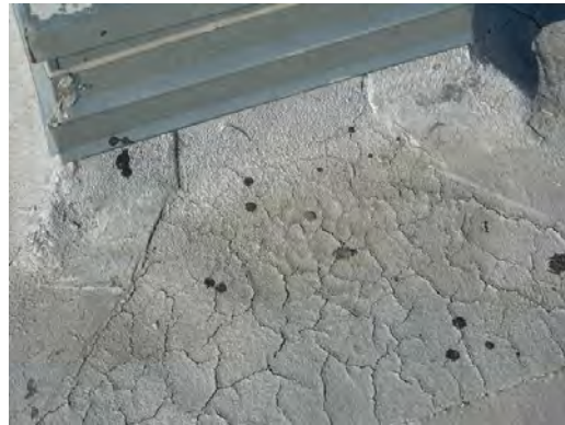
Putnam ES - Cracked Roof Flashing
