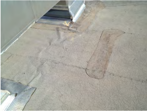
Rusk ES - Bubbling in Roofing Material 02
