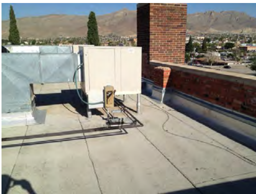
Coldwell ES - Roof General Condition
