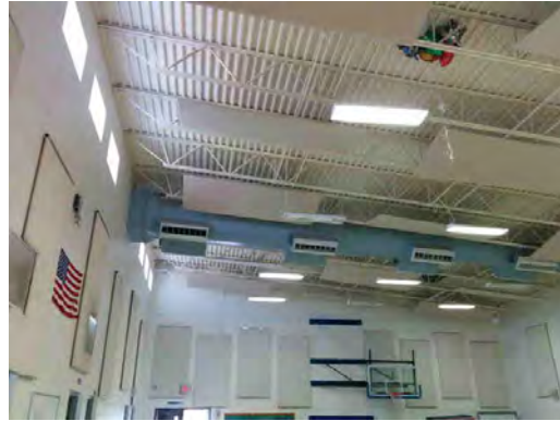
Park ES - Exposed Ceiling in Gym
