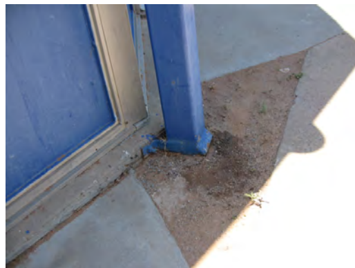
Schuster ES - Buried Storm Water Leader
