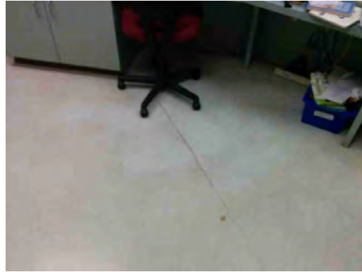
Lamar ES - Damaged Vinyl Tile
