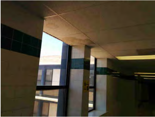
Armendariz MS - Stained Ceiling Tiles
