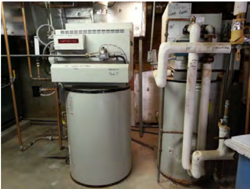
Milam ES - Domestic Water Heaters
