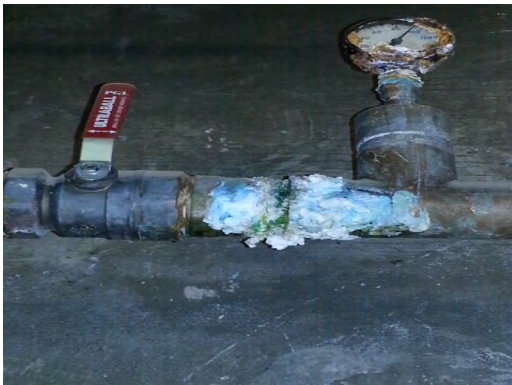
Crosby ES - Water Line Corrosion
