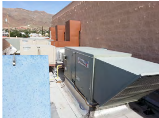
Rusk ES - Gym Furnace Heater
