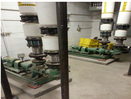
Aoy ES - Heating Water Return Pumps
