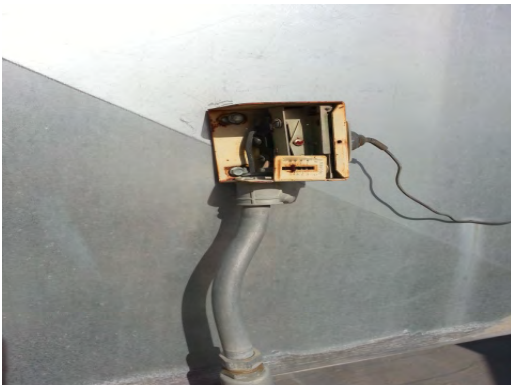
Rusk ES - Damaged EF Sensor
