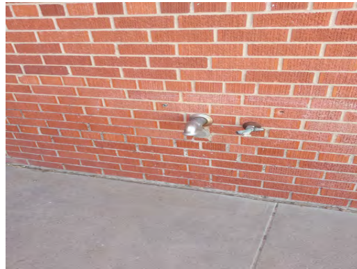
Burleson ES - Missing Foundation
