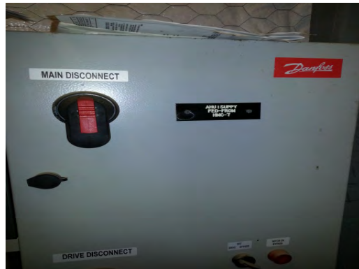
MacArthur ES MS - VFD Controller Disconnect
