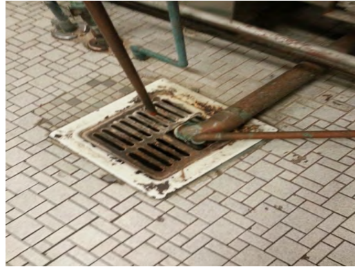
Crosby ES - Corroded Kitchen Drain Cover
