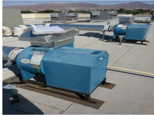
Burgess - Building 12 Rooftop Equipment
