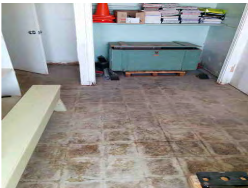
Wainwright ES - Damaged Flooring
