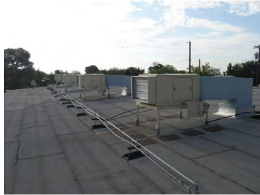
Dowell ES - Older Evap Cooler for Classrooms
