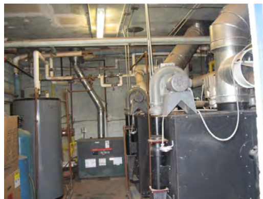
Dowell ES - Mechanical Room
