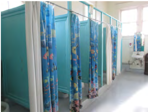
San Jacinto Auit - Restroom Fixtures and Finishes
