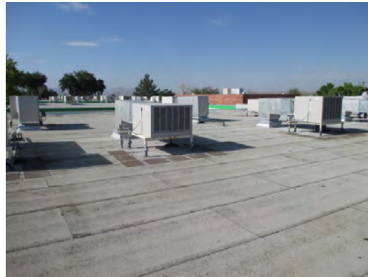
Roberts ES - Roof General Condition
