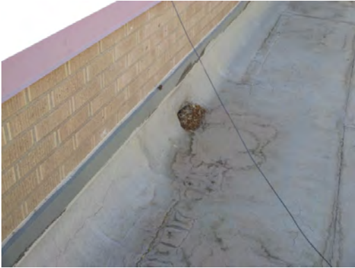
Cooley ES - Clogged Roof Drain
