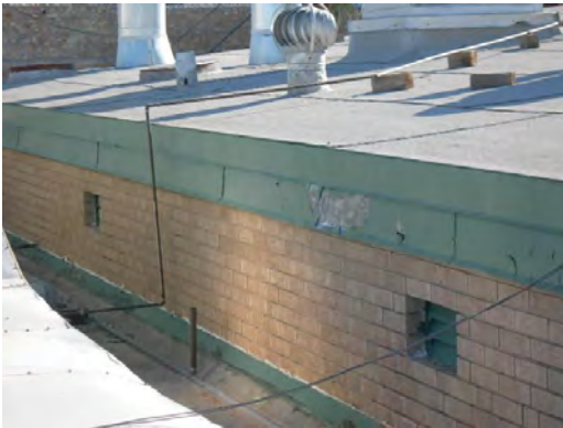
Putnam ES - Paint Peeling on Roof Trim
