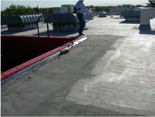
Bradley ES - Roof Condition 02
