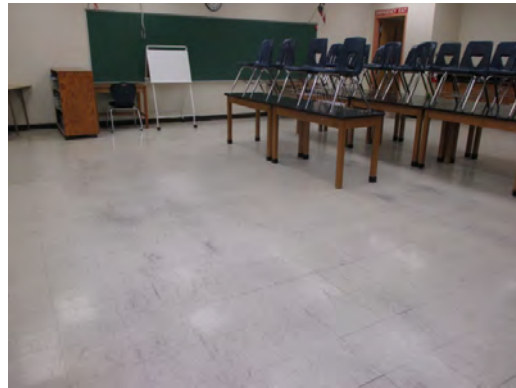
Canyon Hills MS - Worn VCT Flooring 02
