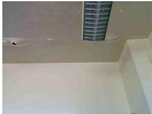
Travis ES - Damaged Ceiling 02
