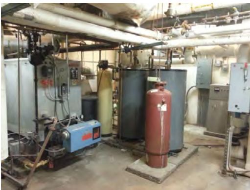
Clendenin ES - Boiler Room
