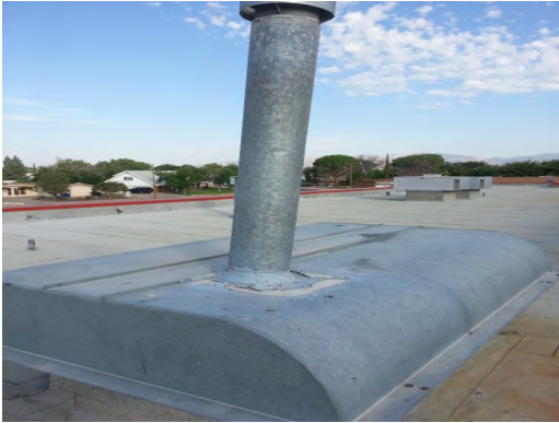
Cielo Vista - Kitchen Roof Ventilator
