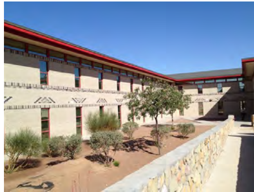
Brown MS - Exterior Finishes
