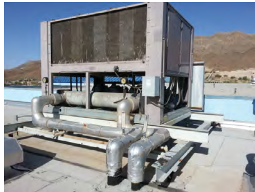
Clendenin ES - Rooftop Chiller
