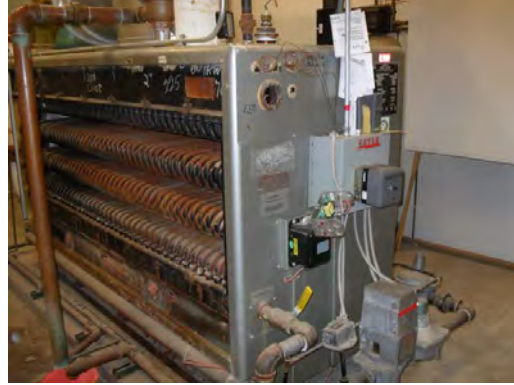
Nixon ES - Damaged Boiler Under Repair
