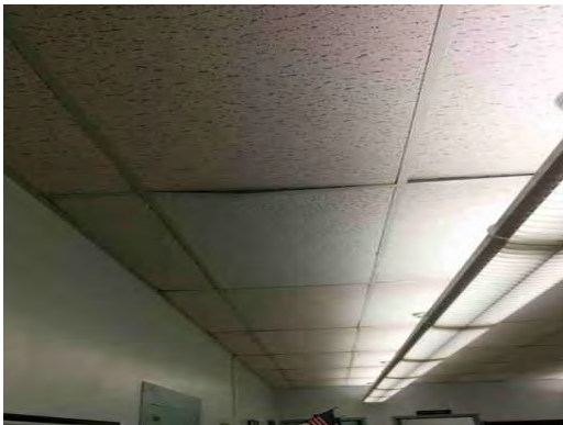
Barron ES - Damaged Ceiling Tiles 01
