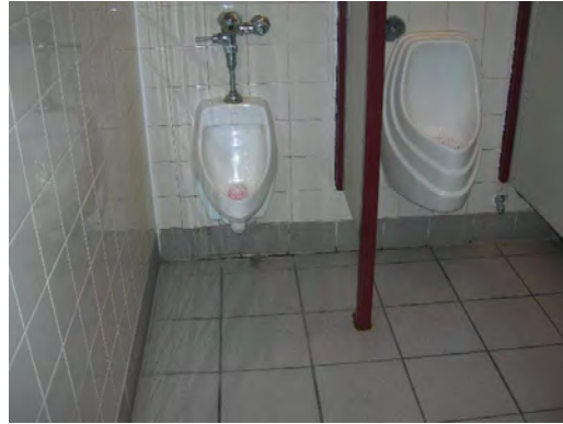
Chapin HS - Restroom Damage
