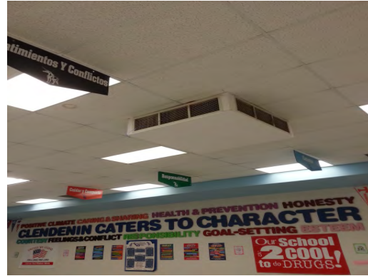
Clendenin ES - Evap Cooler Distribution
