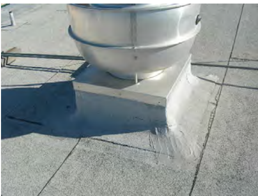
Putnam ES - Roof General Condition 05
