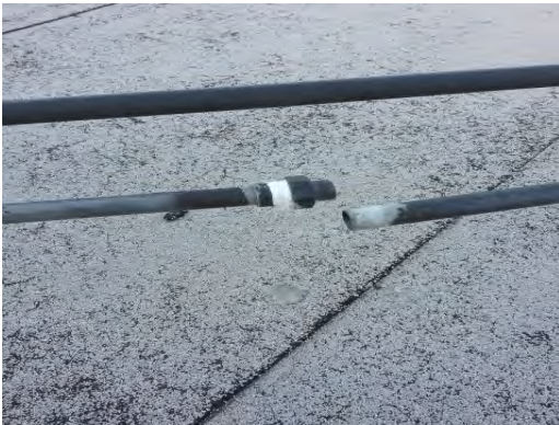
Collins ES - Disconnected Evap Water Line
