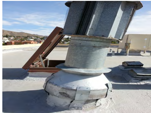
Rusk ES - Damaged Boiler Vent
