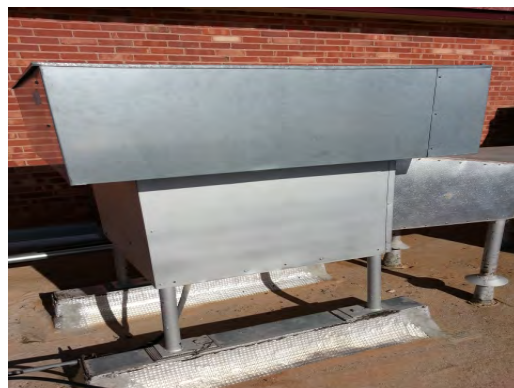
Milam ES - Large Exhaust Fan Above Kitchen
