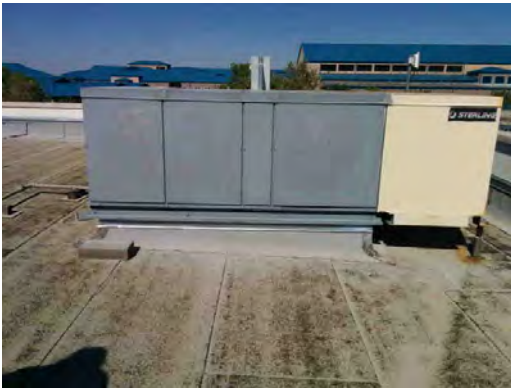
Franklin HS - Rooftop Unit
