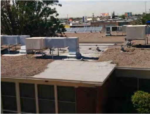
Wainwright ES - Rooftop Units 02
