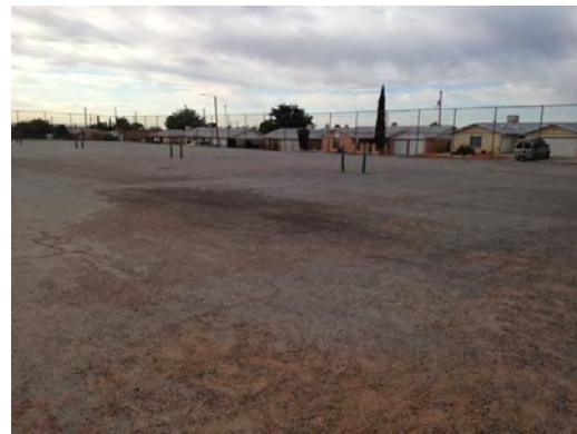
Terrace Hill MS - Worn Play Area Paving
