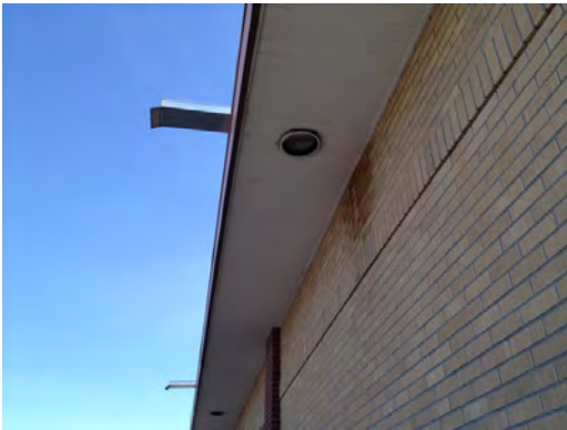
Aoy ES - Evidence of Leak
