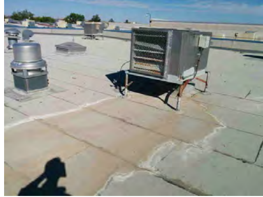
Guerrero ES - Evidence of Ponding on Roof
