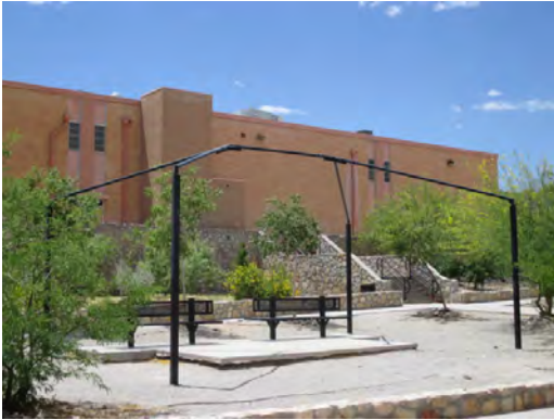
Canyon Hills MS - Missing Canopy
