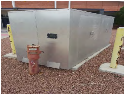
Burgess - Backflow and Post Indicator
