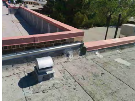
Travis ES - Weathered Roofing Material 01
