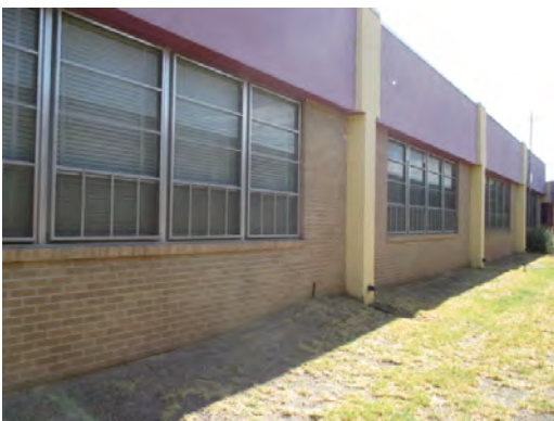
Cooley ES - Exterior Finishes
