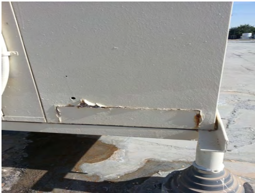
Crosby ES - Damaged Evap
