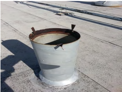
Collins ES - Broken Boiler Stack
