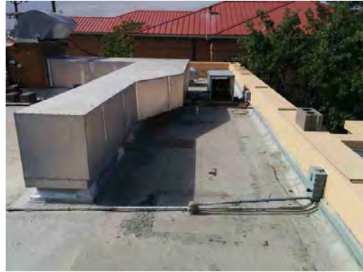
Vilas ES - Rooftop Equipment
