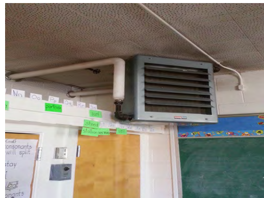
Burleson ES - Classroom Unit Heater
