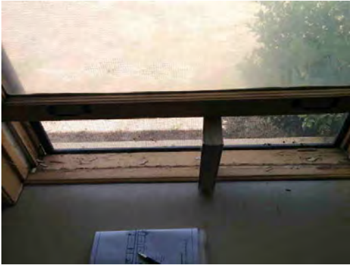
Hawkins ES - Damaged Wood Window 02
