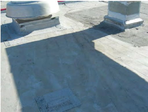
Bradley ES - Roof General Condition
