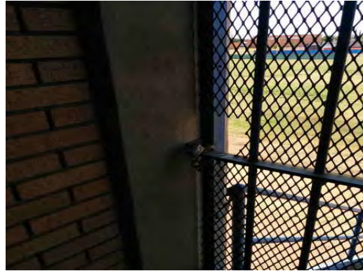
Irvin HS - Damaged Gate
