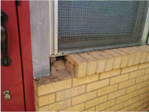
Hillside ES - Damaged Brick Wall at Window
