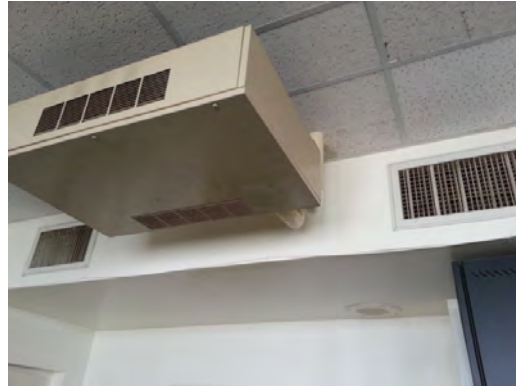
Rusk ES - Typical Classroom Heater
