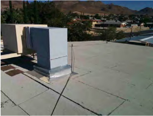
Park ES - Rooftop Equipment 02
