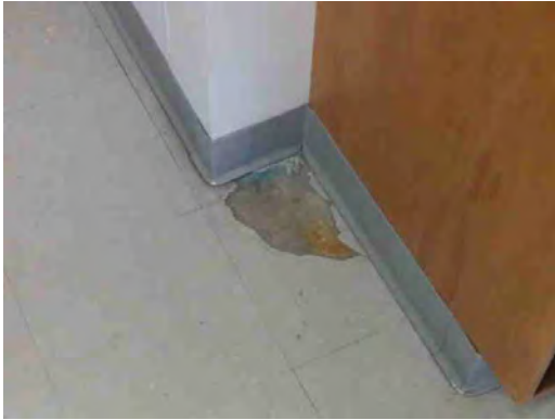
Franklin HS - Damaged VCT Flooring
