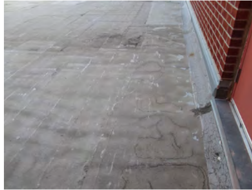
Silva Health Magnet HS - Roofing Material Bubbling
