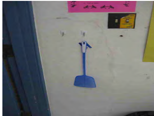
Crosby ES - Damaged Interior Wall
