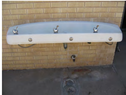
Schuster ES - Inoperable Drinking Fountain
