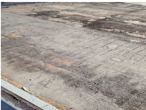
Lincoln MS - Weathered Roofing Material
