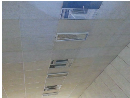
Burgess - Damaged Gym Diffusers
