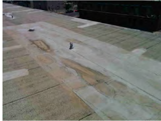
Telles Academy HS - Evidence of Ponding on Roof
