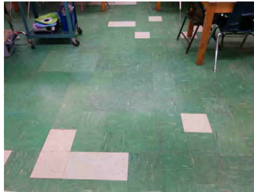
Irvin HS - Mismatched Tile Repair 02
