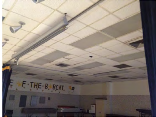
Cielo Vista - Cafeteria Ceiling
