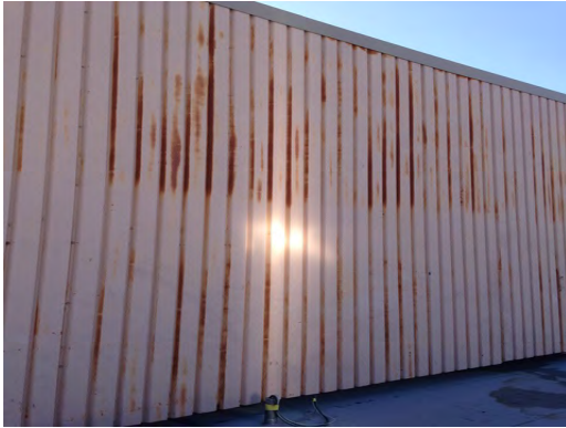
Lincoln MS - Rust at Gym Wall
