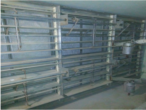
Cielo Vista - Disabled Evap Damper
