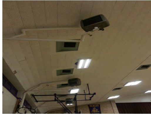
Burges - Typical Gym Unit Heaters
