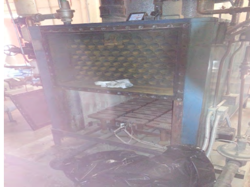
Bradley ES - Boiler Undergoing Repair
