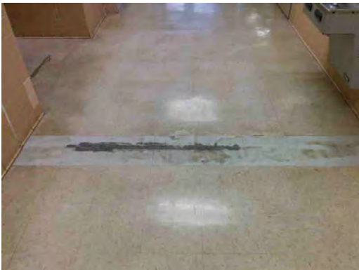
Lee ES - Damaged VCT Flooring
