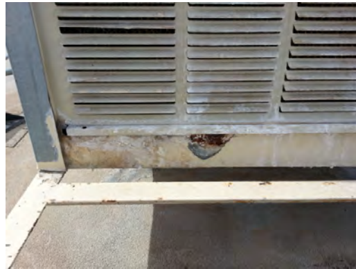
Coronado HS - Corroded Evap
