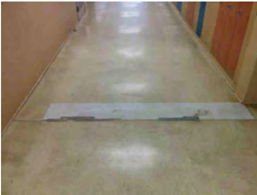
Lee ES - Damaged VCT Flooring 03
