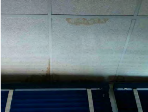
Bowie HS - Stained Ceiling Tiles
