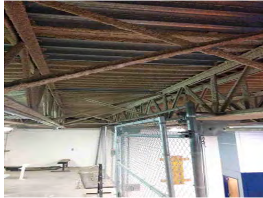
Irvin HS - Exposed Metal Ceiling
