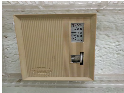
Alta Vista ES - Dated Pneumatic Thermostat
