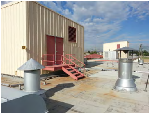
MacArthur ES MS - AHU Rooftop Penthouses
