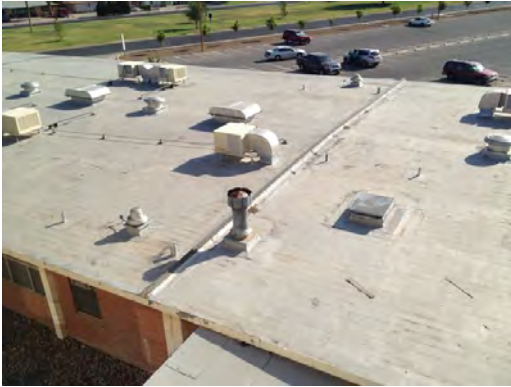
Burgess - Rooftop Equipment
