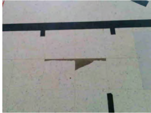
Travis ES - Damaged VCT Flooring
