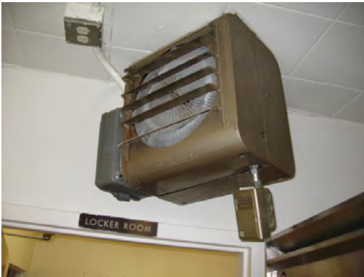
Schuster ES - Electric Unit Heater
