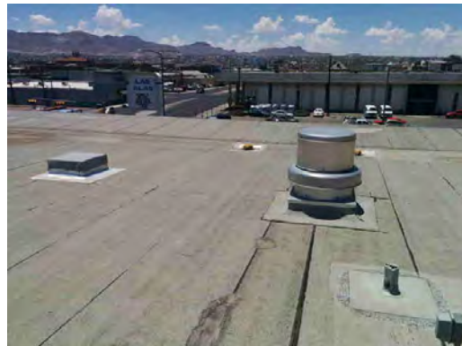
Telles Academy HS - Roof Exhaust
