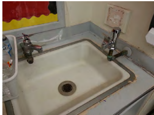
Milam ES - Typical Classroom Lavatory and Faucets
