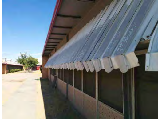
Hillside ES - Damaged Metal Awning
