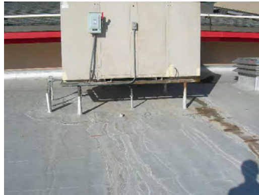
Brown MS - Weathered Parapet Roof
