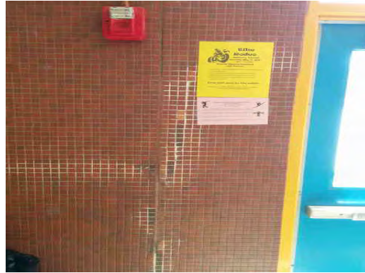
Barron ES - Damaged Tile Wall
