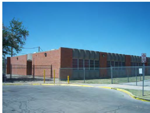
Jefferson HS - Building 4 Elevation
