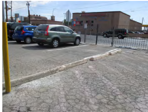
Silva Health Magnet HS - Weathered Asphalt Paving
