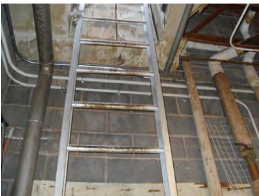
Newman ES - Worn Roof Ladder
