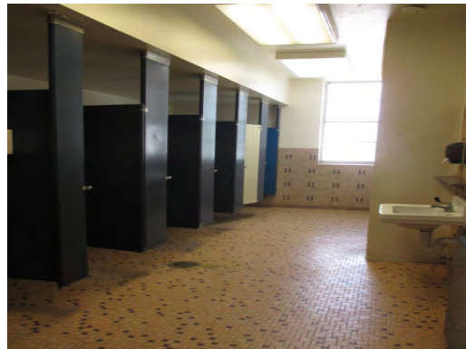
Henderson MS - Restroom Finishes
