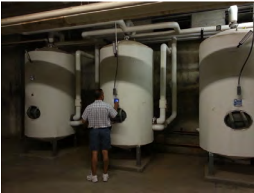
Burgess - Hot Water Storage tanks
