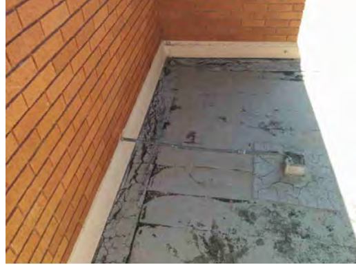
Beall ES - Cracked Roofing
