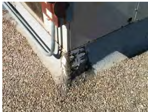
Wainwright ES - Damaged Equipment Curb
