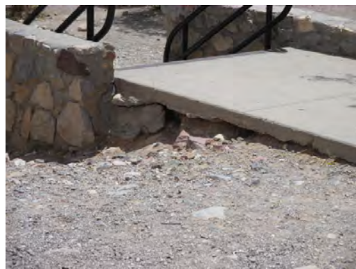
Canyon Hills MS - Erosion at Sidewalk
