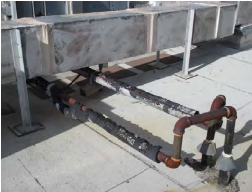
Canyon Hills MS - Rooftop Equipment 03
