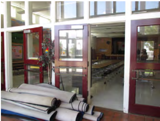
Clardy ES - Cafeteria Entry Doors
