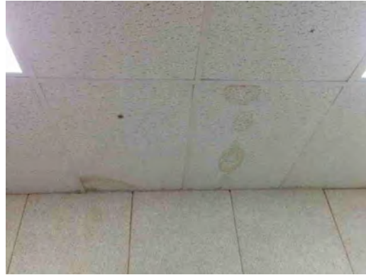
Magoffin MS - Stained Ceiling Tiles
