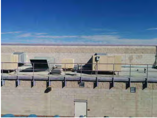
Guerrero ES - Rooftop Equipment
