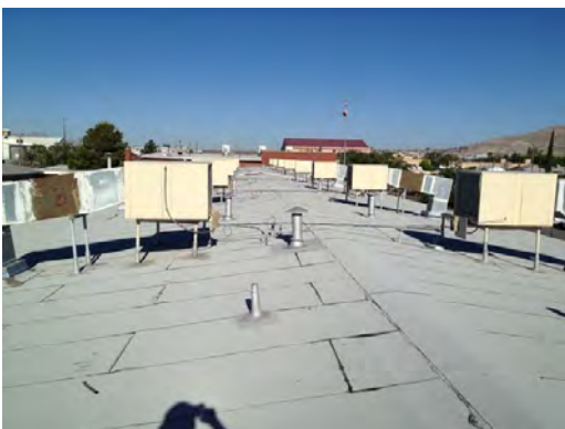
Burleson ES - Roof General Condition 02
