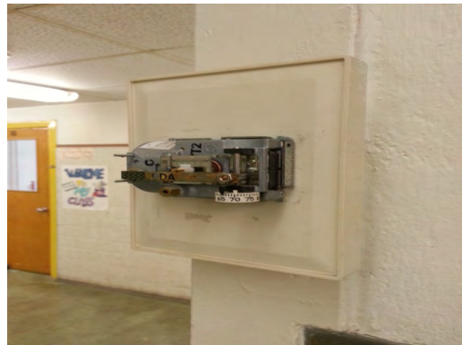
Rusk ES - Damaged Thermostat
