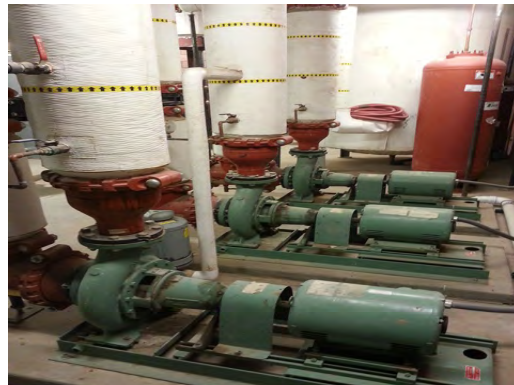
Chapin HS - Hot Water Supply
