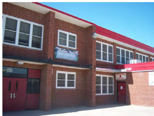
Jefferson HS - Building 9 Elevation
