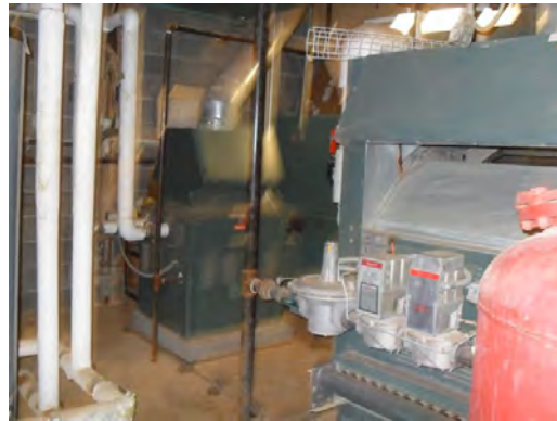
Newman ES - Mechanical Room 02
