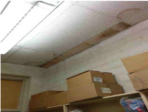
Hawkins ES - Stained Ceiling Tiles 01
