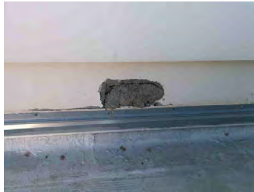
Barron ES - Wall Patch on Roof
