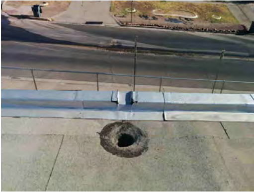
Lamar ES - Roof Drain
