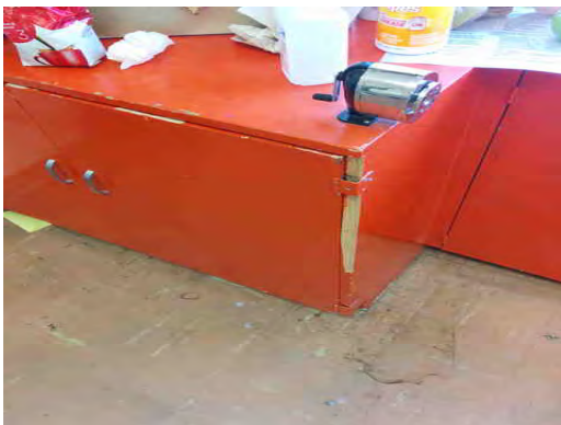
Lamar ES - Damaged Cabinetry
