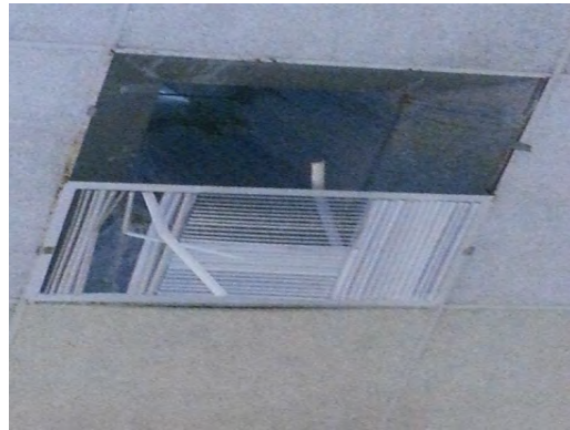
Burgess - Damaged Air Diffusers
