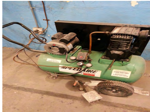
Alta Vista ES - Non-Standard Pneumatic Compressor
