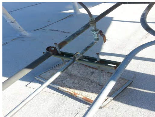
Burleson ES - Non-Insulated Water Piping
