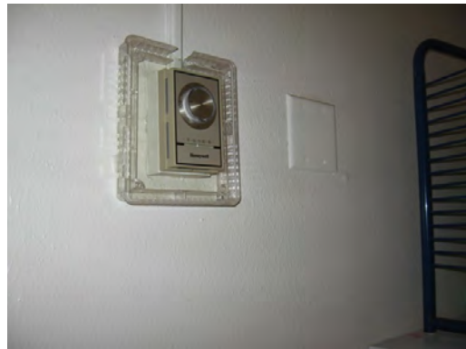
Dowell ES - Typical Electrical Thermostat
