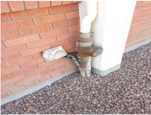
Burgess - Sanitary Sewer Vent
