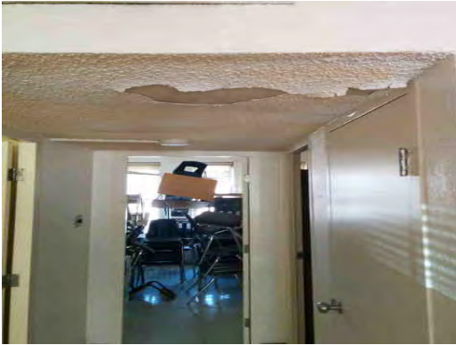
Lamar ES - Damaged Ceiling
