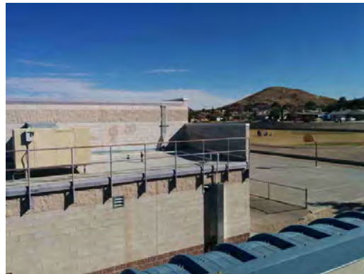
Guerrero ES - Rooftop Equipment 02
