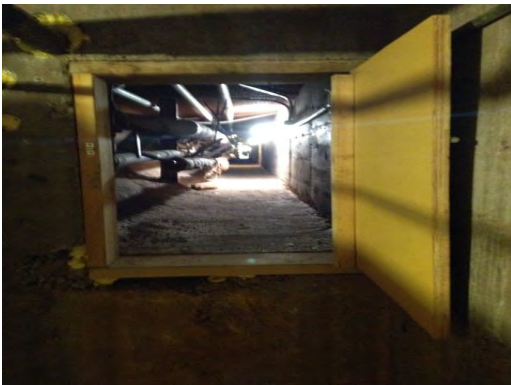
Burnet ES - Tunnel
