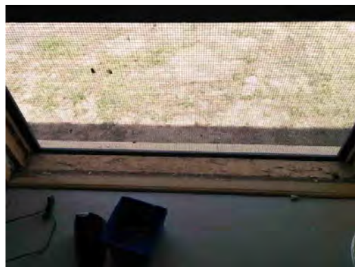
Hawkins ES - Damaged Wood Window 01
