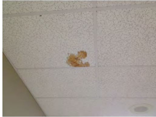
Brown MS - Stained Ceiling Tiles
