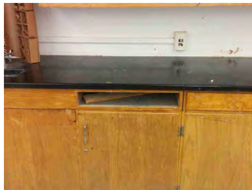
Irvin HS - Damaged Cabinetry
