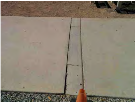
Beall ES - Damaged Pedestrian Paving
