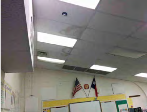
Hillside ES - Stained Ceiling Tiles
