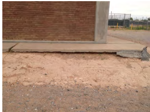
Address HS - Erosion at Sidewalk
