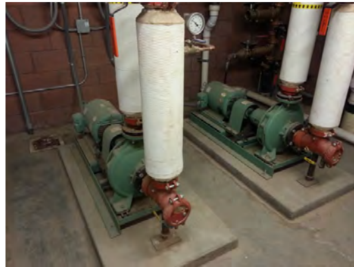
Chapin HS - Hot Water Return Pumps
