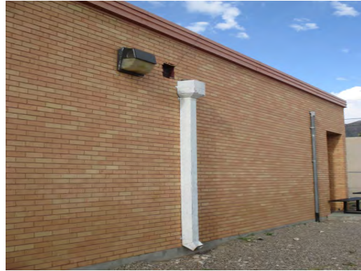
Canyon Hills MS - Downspout Missing Splashblock
