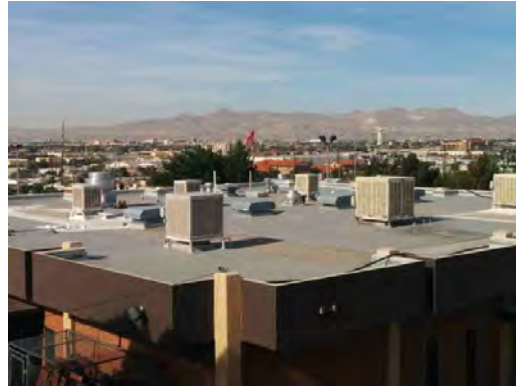
Hawkins ES - Rooftop Equipment 02
