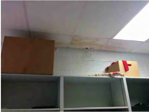
Irvin HS - Stained Ceiling Tiles
