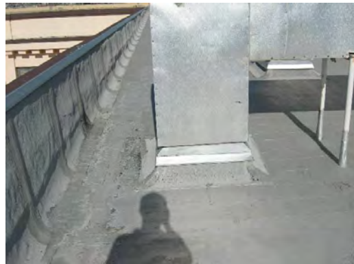
Alta Vista ES - Roof General Condition 2
