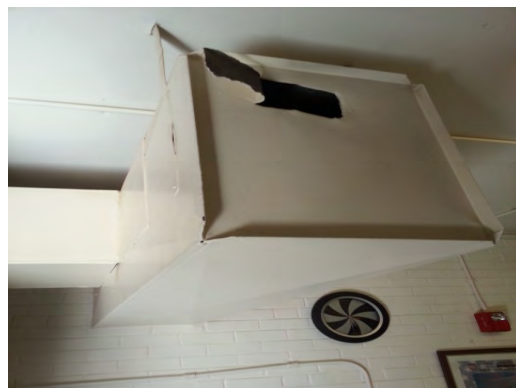
Burgess - Damaged Duct at ROTC Office
