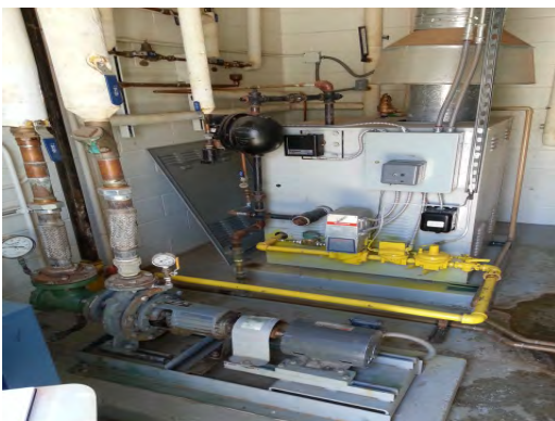
Green ES - Heating Boiler and Circulation Pump
