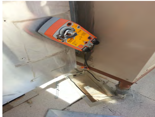
Rusk ES - Dislodged Damper Motor on Duct 01
