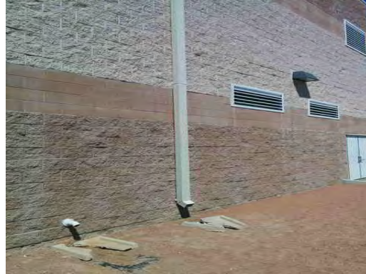
Western Hills ES - Downspouts
