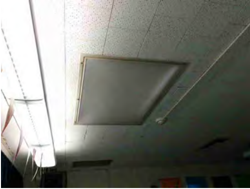
Dowell ES - Adhered tile Ceiling
