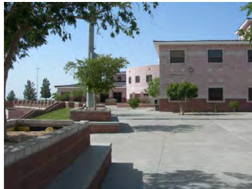
Chapin HS - Rear Elevation 02
