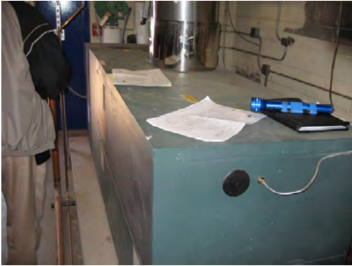
Schuster ES - Heating Boiler
