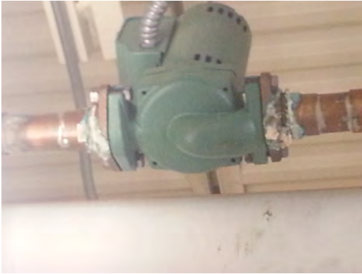
Burgess - Building 12 Heating Pumps Leakings
