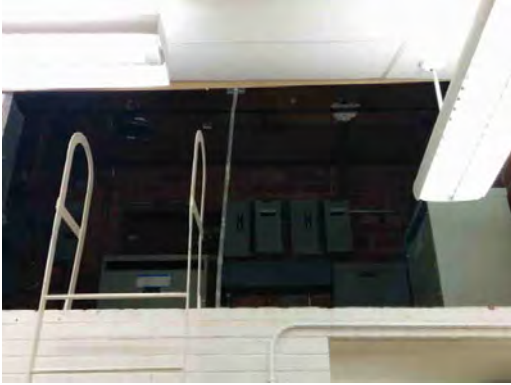
Hawkins ES - Access Blocked to Panels
