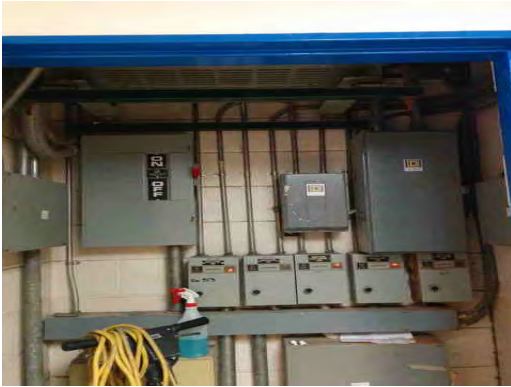
Lee ES - Electrical Room
