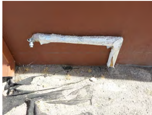
Rusk ES - Reinsulate Hose Bibb Piping
