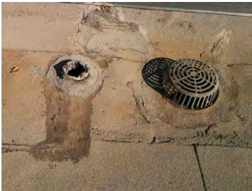
Guerrero ES - Weathered Roof at Drain and Vent
