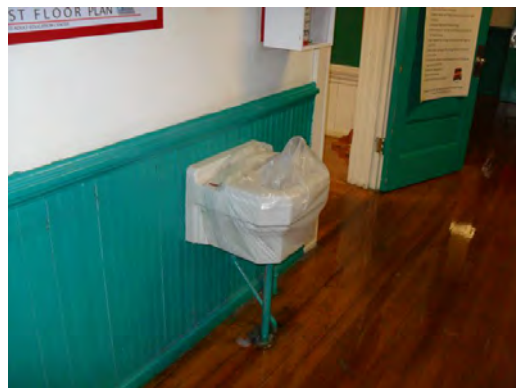
San Jacinto Auit - Damaged Drinking Fountain
