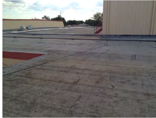
MacArthur ES MS - Roof Condition 02
