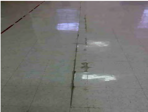
Hillside ES - Damaged VCT Flooring
