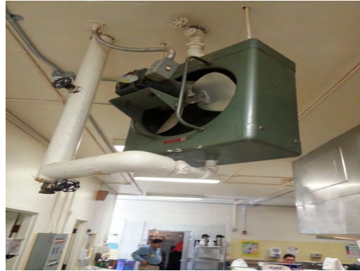
Crosby ES - Kitchen Unit Heater
