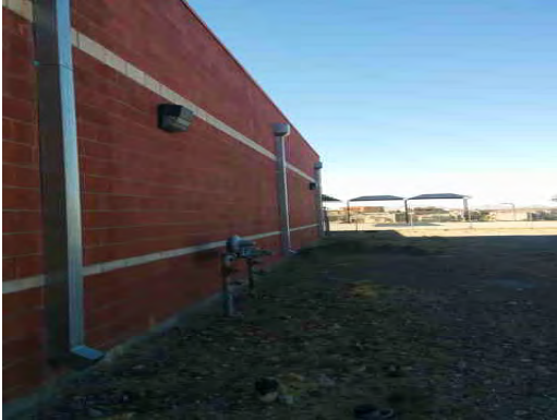
Tippin ES - Downspouts Missing Splashblocks
