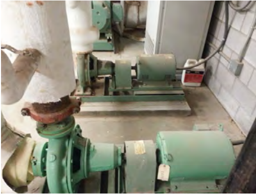
Chapin HS - Heating Water Return Pumps
