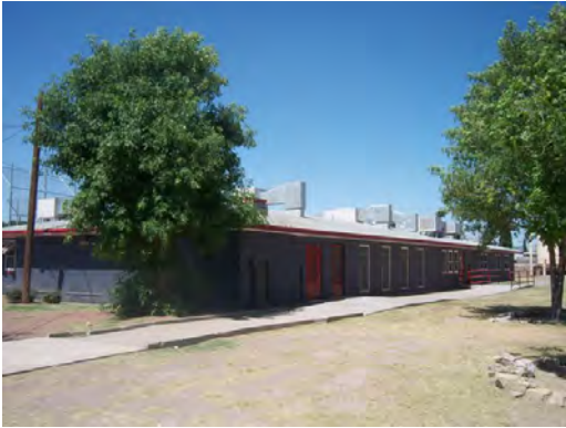
Jefferson HS - Building 5 Elevation
