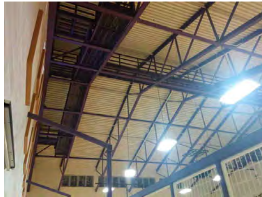
Franklin HS - Exposed Ceiling
