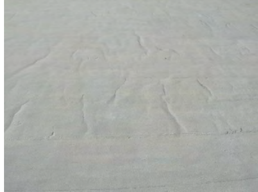
Brown MS - Bubbled Roofing 02
