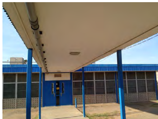
Collins ES - Covered Walkway
