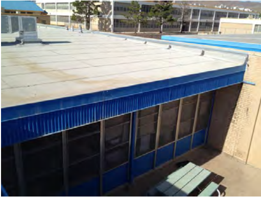
Collins ES - Roof General Condition 01
