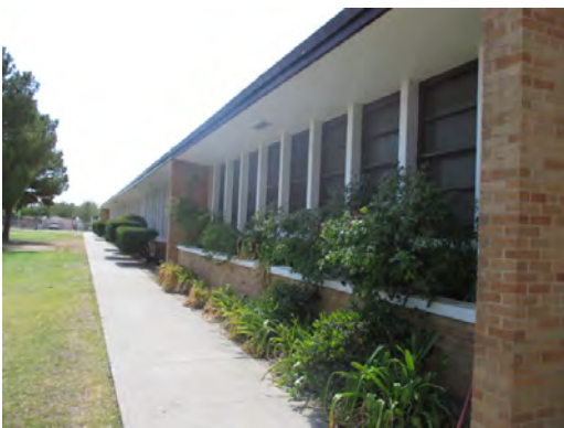
Clardy ES - Exterior Finishes
