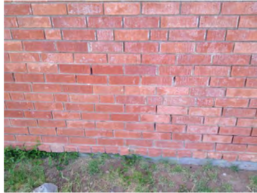
Burgess - Exterior Brick Wall
