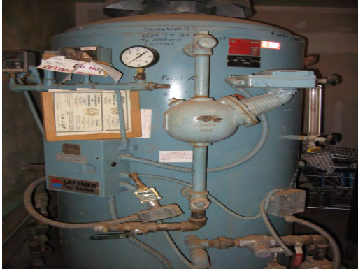
Schuster ES - Abandoned Domestic Water Boiler
