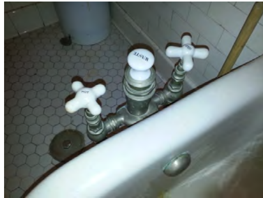
El Paso HS - Dated Tub Valves
