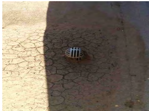
Hughey ES - Cracked Roofing Material
