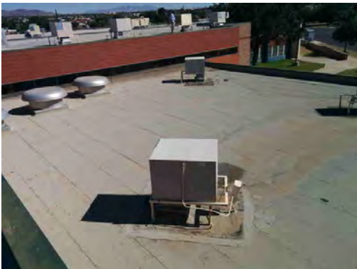
Irvin HS - Rooftop Equipment
