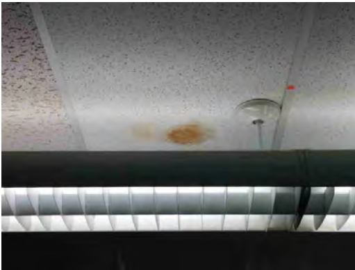
Vilas ES - Stained Ceiling Tiles
