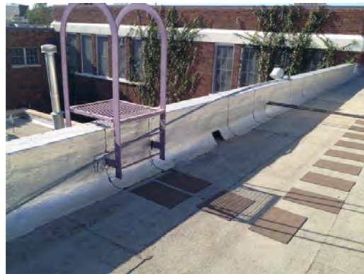
Coldwell ES - Roof Ladder
