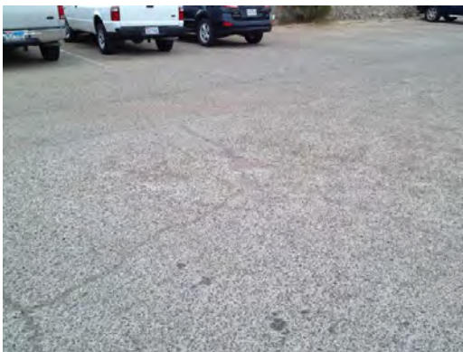
Coronado HS -Parking Lot Paving
