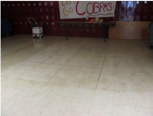
Canyon Hills MS - Worn VCT Flooring
