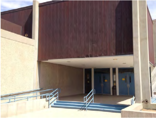
Johnson ES - Entry Doors
