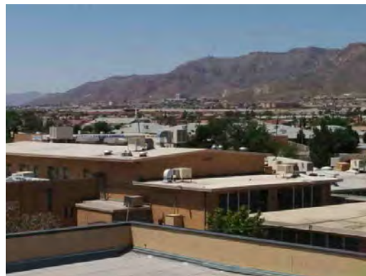
Magoffin MS - Rooftop Equipment 02
