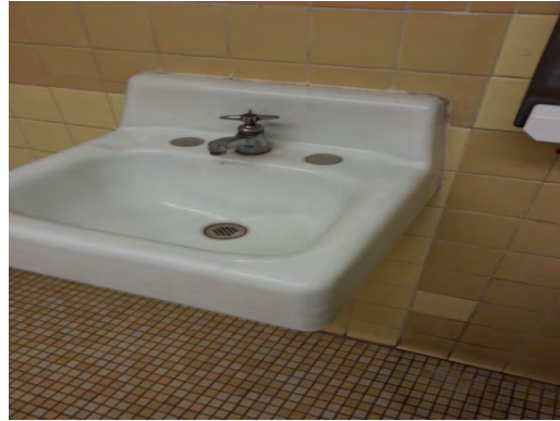
Rusk ES - Dated Plumbing Fixtures
