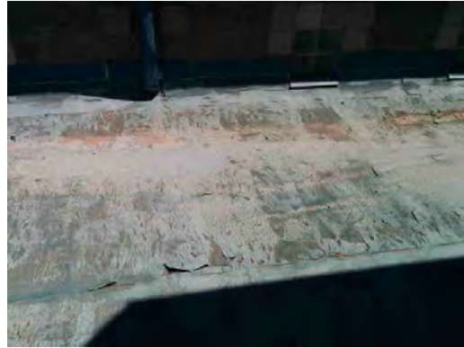
Franklin HS - Weathered Roofing 02
