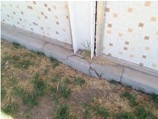
Burleson ES - Crack in Foundation
