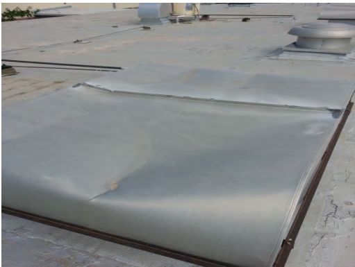
Burges - Repair Roof Vent Housing
