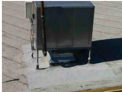
Lamar ES - Rooftop Equipment
