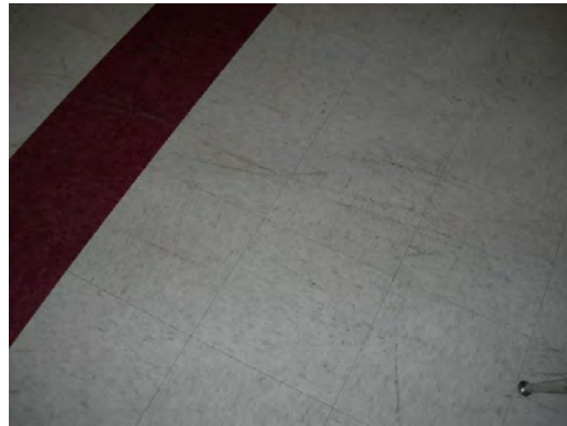
Chapin HS - Flooring General Condition
