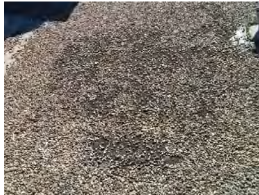
Wainwright ES - Evidence of Ponding on Roof
