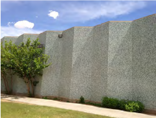
Address HS - Building 5 Side Elevation
