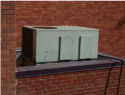
Burges - Old Trane AC Unit
