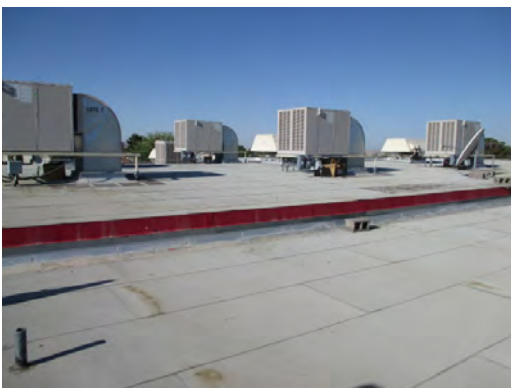
Polk ES - Rooftop Equipment 01
