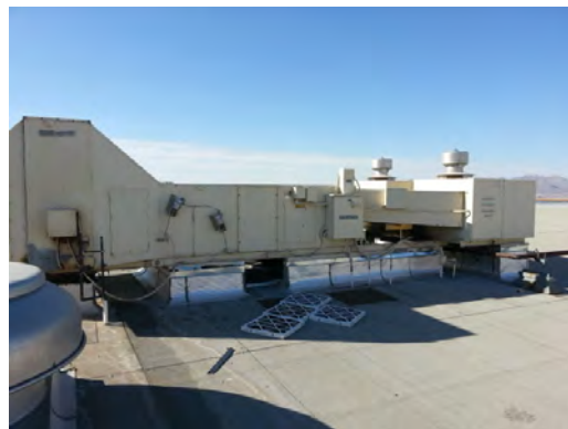
Green ES - Corroded Furnace-Evap Combo Unit
