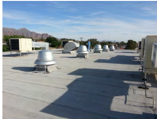
Collins ES - Classroom Roof Exhaust Hoods
