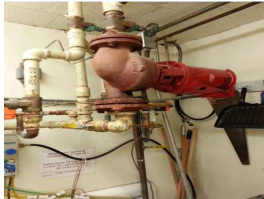
Milam ES - Heating Pump in Custodial Closet
