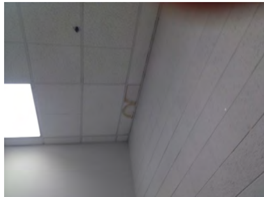
Aoy ES - Stained Ceiling Tiles
