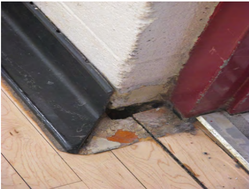
Franklin 9th Grade Center - Damaged Cove Base at Gym
