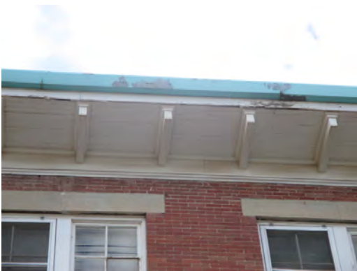
San Jacinto Auit - Damaged Soffit
