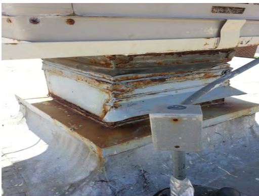
Crosby ES - Rusted Duct Inlet
