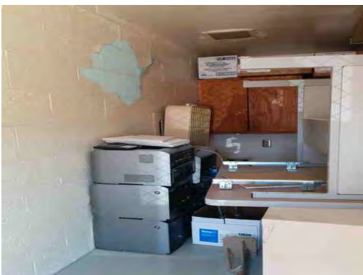
Lamar ES - Paint Peeling at Storage
