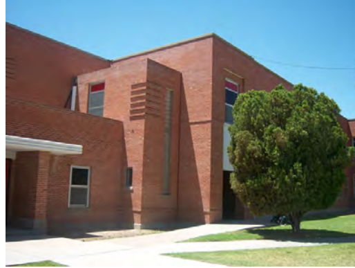
Jefferson HS - Building 1 Exterior 02
