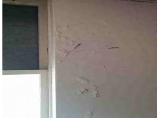
Hawkins ES - Damaged Interior Wall 01
