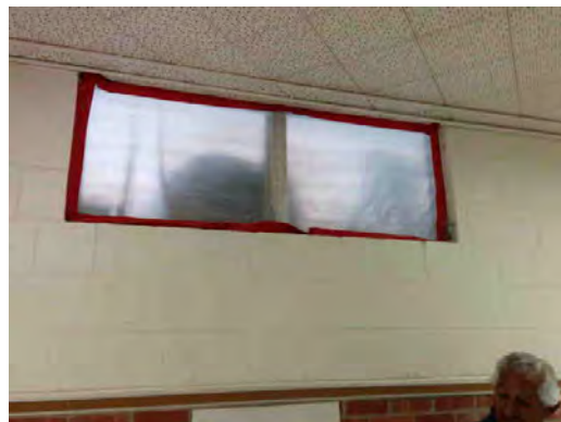
Dowell ES - Damaged Window
