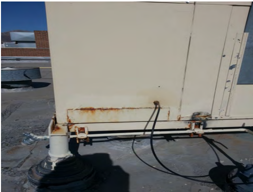
Crosby ES - Corrosion on Evap
