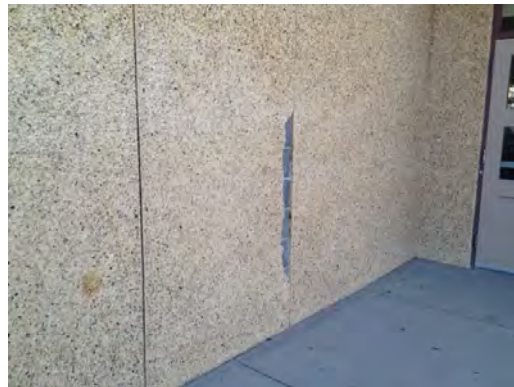
Charles MS - Damaged Stone Wall
