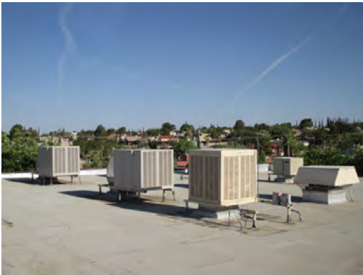
Polk ES Rooftop Equipment 05
