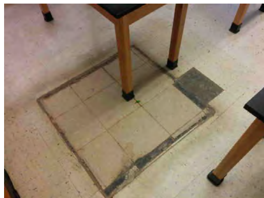
Irvin HS - Damaged VCT Flooring
