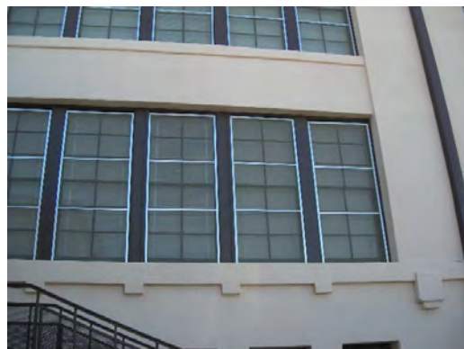
Alta Vista ES - Windows General Condition
