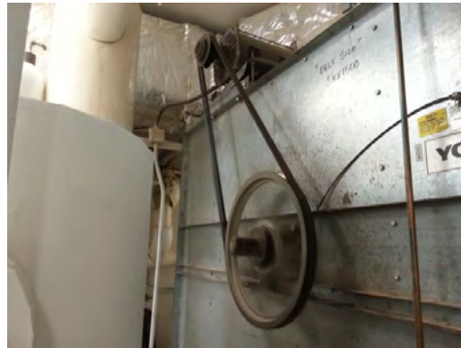
Clendenin ES - Missing Pulley Guard
