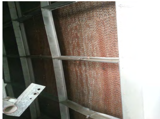
Cielo Vista - Room Evap
