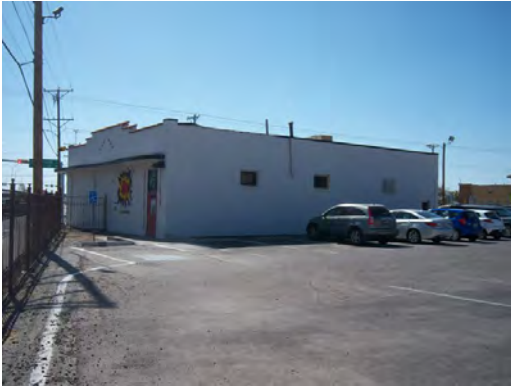
Jefferson HS - Building 11 Elevation
