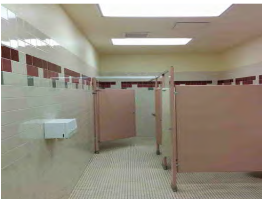
Guillen MS - Restroom Finishes
