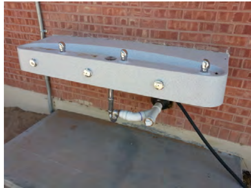
Milam ES - New Exterior Water Fountain
