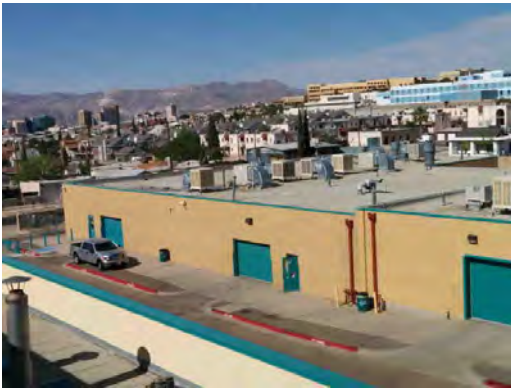
Center for Career & Tech - Roof Elevation
