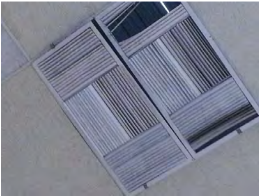
Burgess - Damaged Gym Air Diffusers
