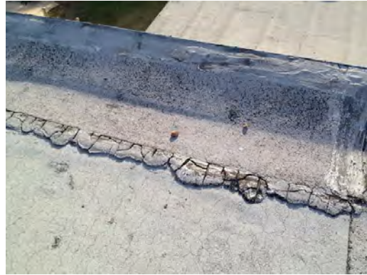
Collins ES - Damaged Roof Flashing
