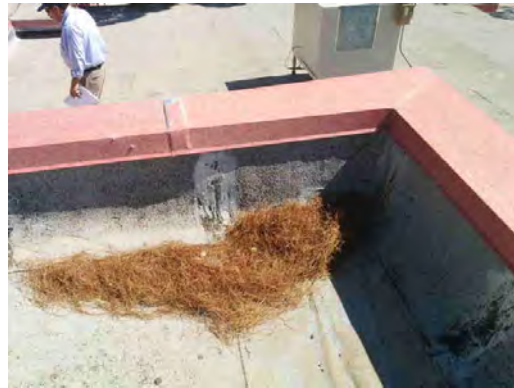
Travis ES - Debris on Roof
