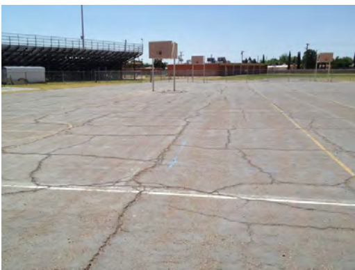
Burgess - Damaged Asphalt Basketball Paving
