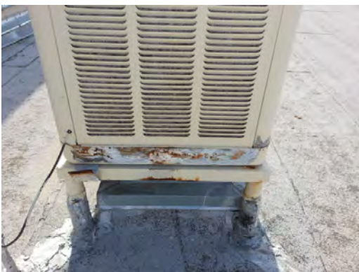
Collins ES - Corroded Evap
