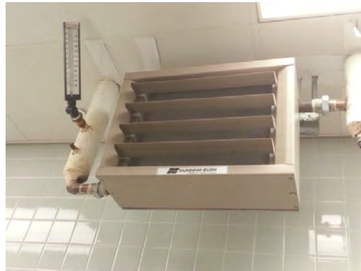
Clendenin ES - Unit Heater
