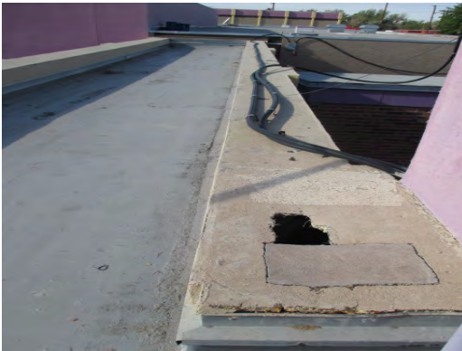
Cooley ES - Damaged Coping
