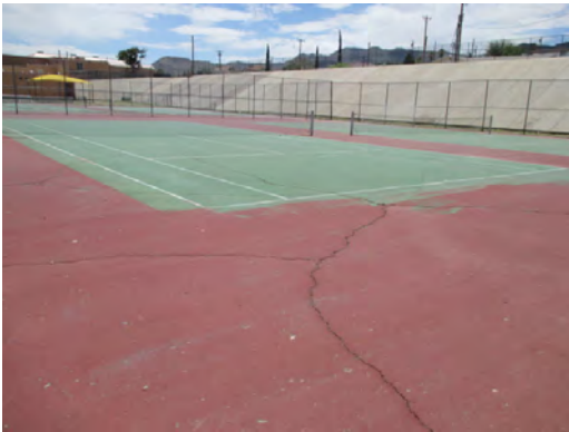
Canyon Hills MS - Crack in Paved Play Area
