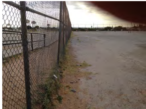
Terrace Hills MS - Damaged Chain Link Fence
