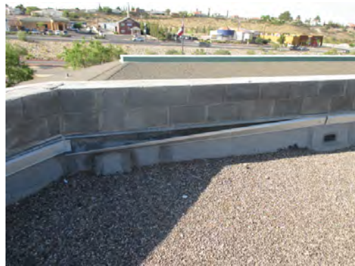
Franklin 9th Grade Center - Damaged Flashing
