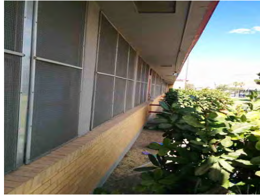
Hillside ES - Typical Weathered Windows
