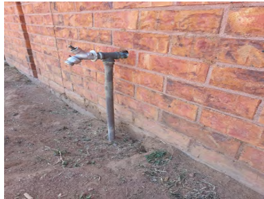
Bradley ES - Insulated Piping 02
