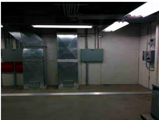
Hornedo MS - Electrical Room
