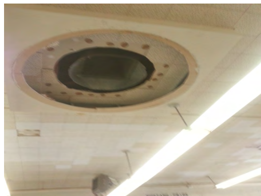
Burgess - Missing Diffusers
