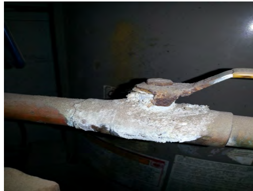
Rusk ES - Leaking Ball Valve
