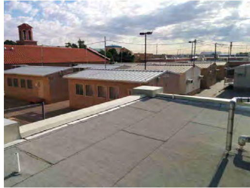
Guillen MS - Roof General Condition
