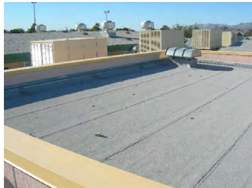
Putnam ES - Roof Flashing 02
