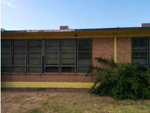
Hughey ES - Typical Window Condition
