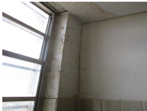
Canyon Hills MS - Damaged Interior Wall and Ceiling, Evidence of Leak
