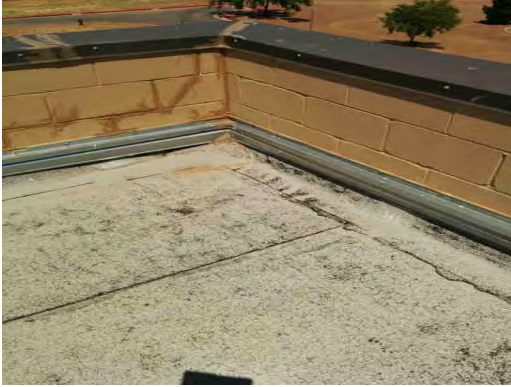
Magoffin MS - Weathered Roofing Material
