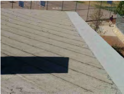
Lamar ES - Roof General Condition
