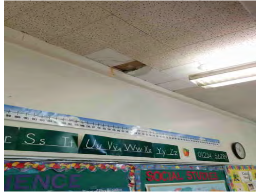
Bliss ES - Damaged Ceiling Tiles
