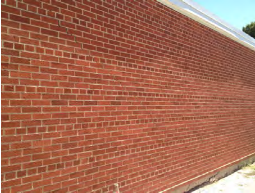
Burleson ES - Cracked Exterior Brick 02
