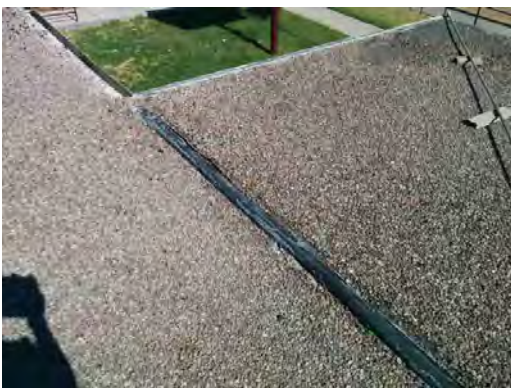
Wainwright ES - Evidence of Ponding on Roof 02
