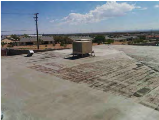
Travis ES - Roof General Condition 01
