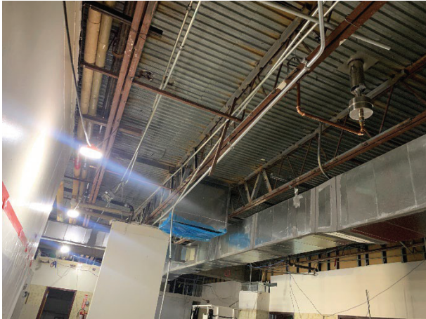
Figure 1. Missing web reinforcement on the north end of joist "F".
