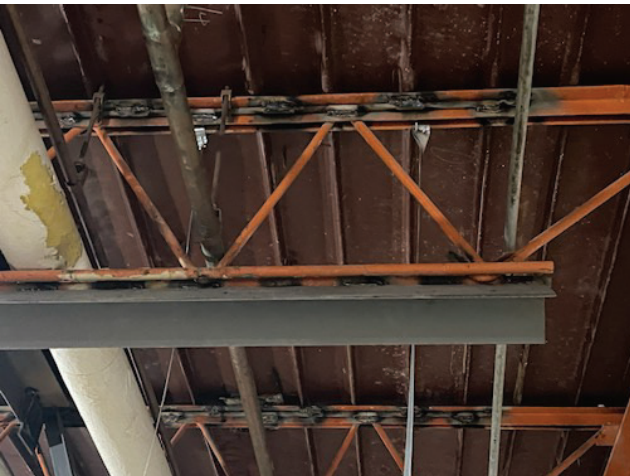
Reinforcement of existing joist.
