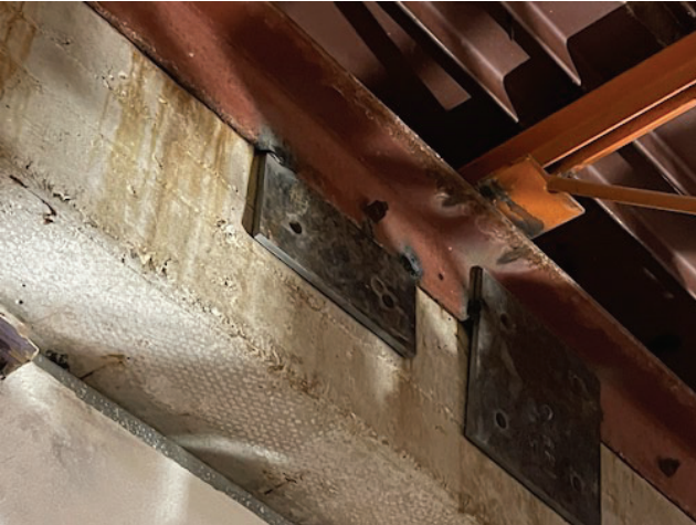
Contractor has installed alternate variation of specified joist seat support.
