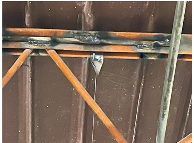
Welding of reinforcement to existing joist.
