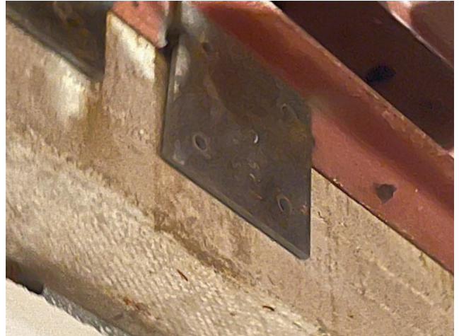
Reinforcement plate at face of existing concrete beam.
