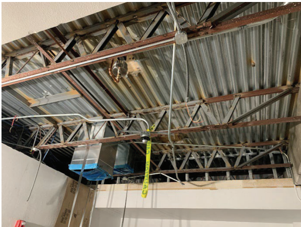
Figure 3. Reinforcement at Joist "G" north end.
