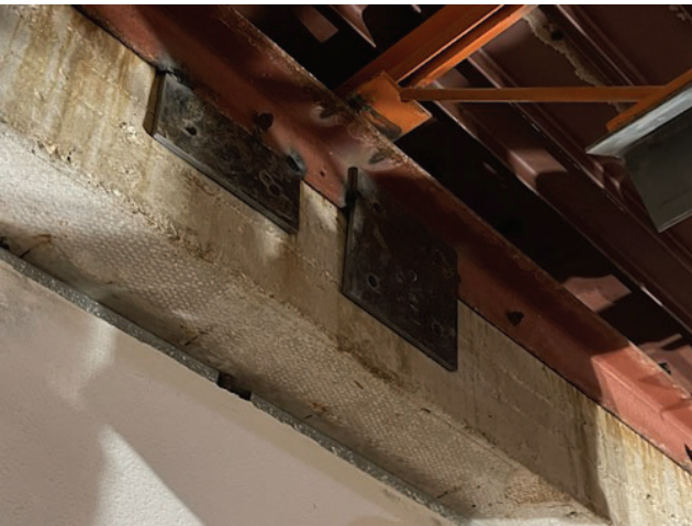
Contractor has installed alternate variation of specified joist seat support.
